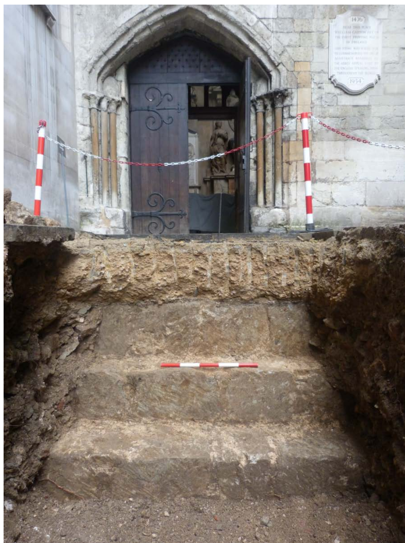
Plate 3: Stepped Footing [8] for South Transept, View to West
