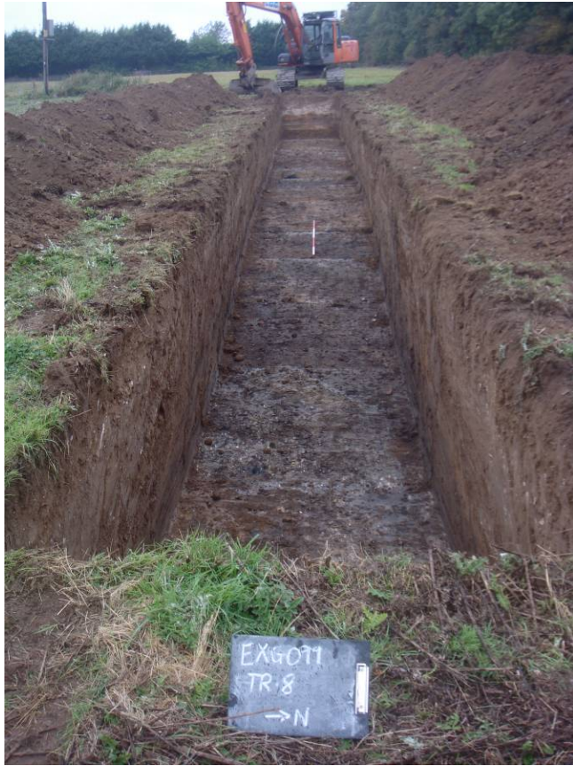
PLATE 9: Trench 8, view west. Excavation ceased within the fill (13) of a large quarry pit.
