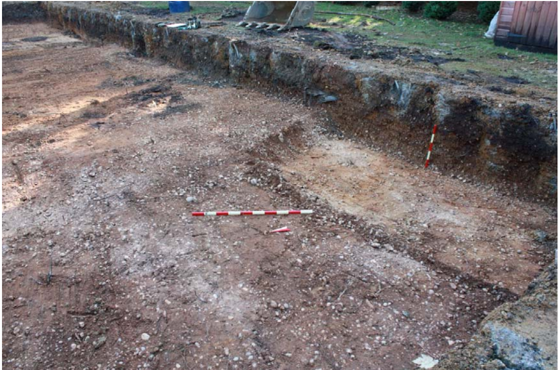
Plate 1: D1.4 taken 16/10/12. TR 1. Machine dug slot in the south western corner of the site showing the lighter sandy gravel [3] below the darker red brown gravelly sand [2]. Scales 1m and 0.5m looking E. The newly installed concrete pile wall can be seen flanking the trench edge.
