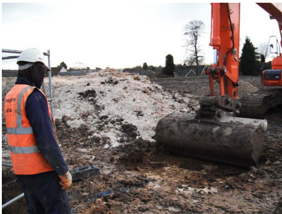
PLATE 14: Cutting of pipe trench under watching brief conditions
