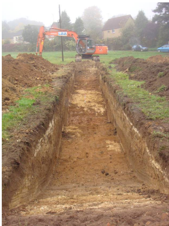
PLATE 9: Trench 5, view west
