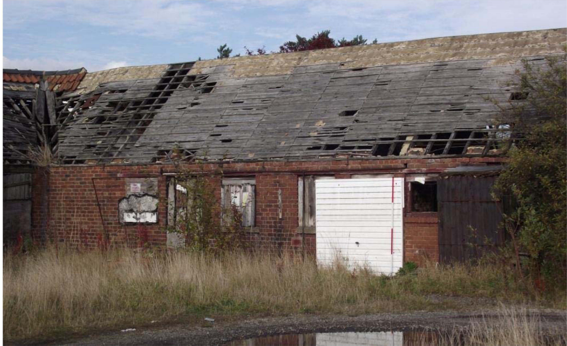
Photograph 15: North range, south-east facing elevation, oblique view (2m scale)
