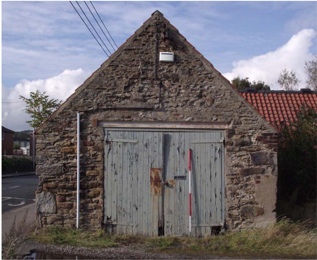
Photograph 11: South range, south-east facing gable elevation, front on view (2m scale)
