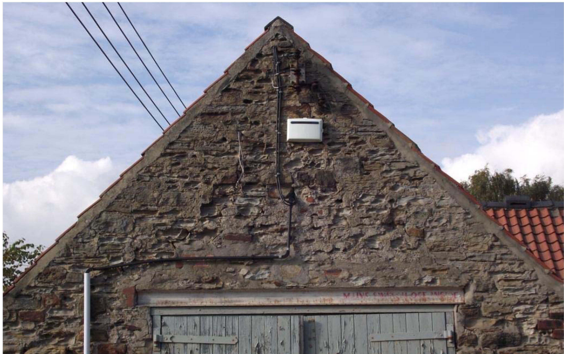
Photograph 12: South range, south-east facing gable elevation, upper part detail (no scale)
