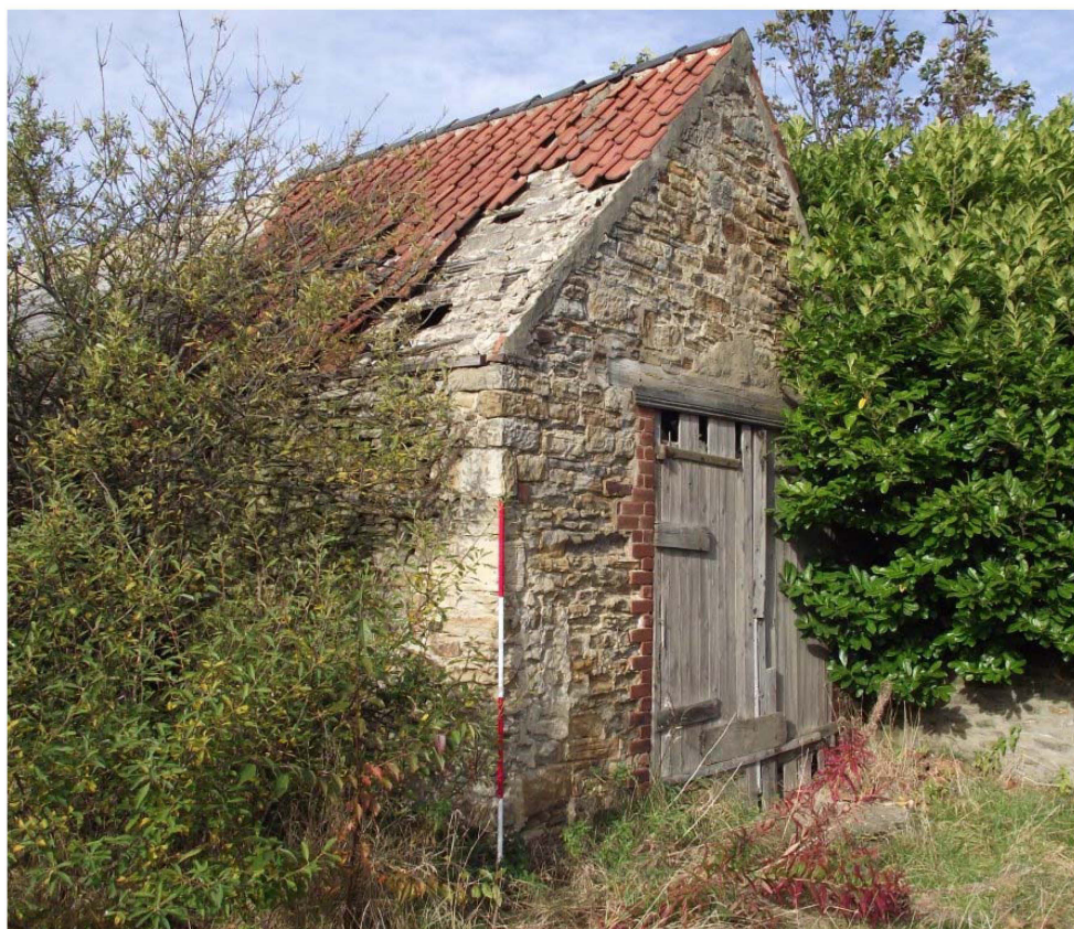
Photograph 18: North range, southern gable end, looking north (2m scale)
