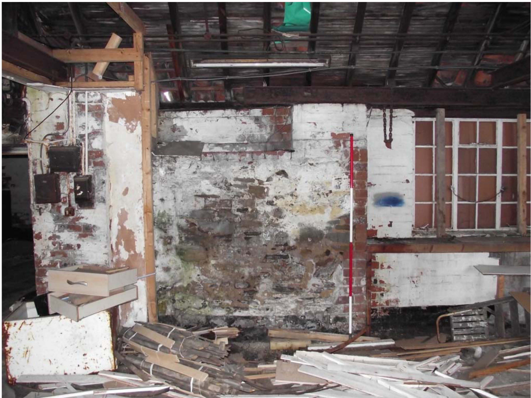
Photograph 30: South range, internal, north wall, detail, looking north-west (2m scale)
