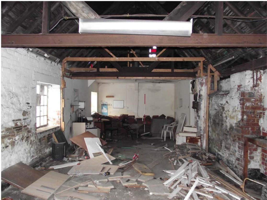
Photograph 25: South range, internal, looking north-west (2m scale)
