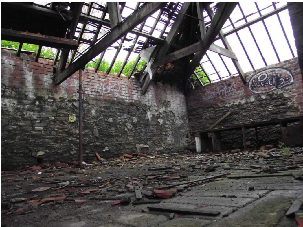
Photograph 36: West range, internal, north-eastern room, looking north (no scale)
