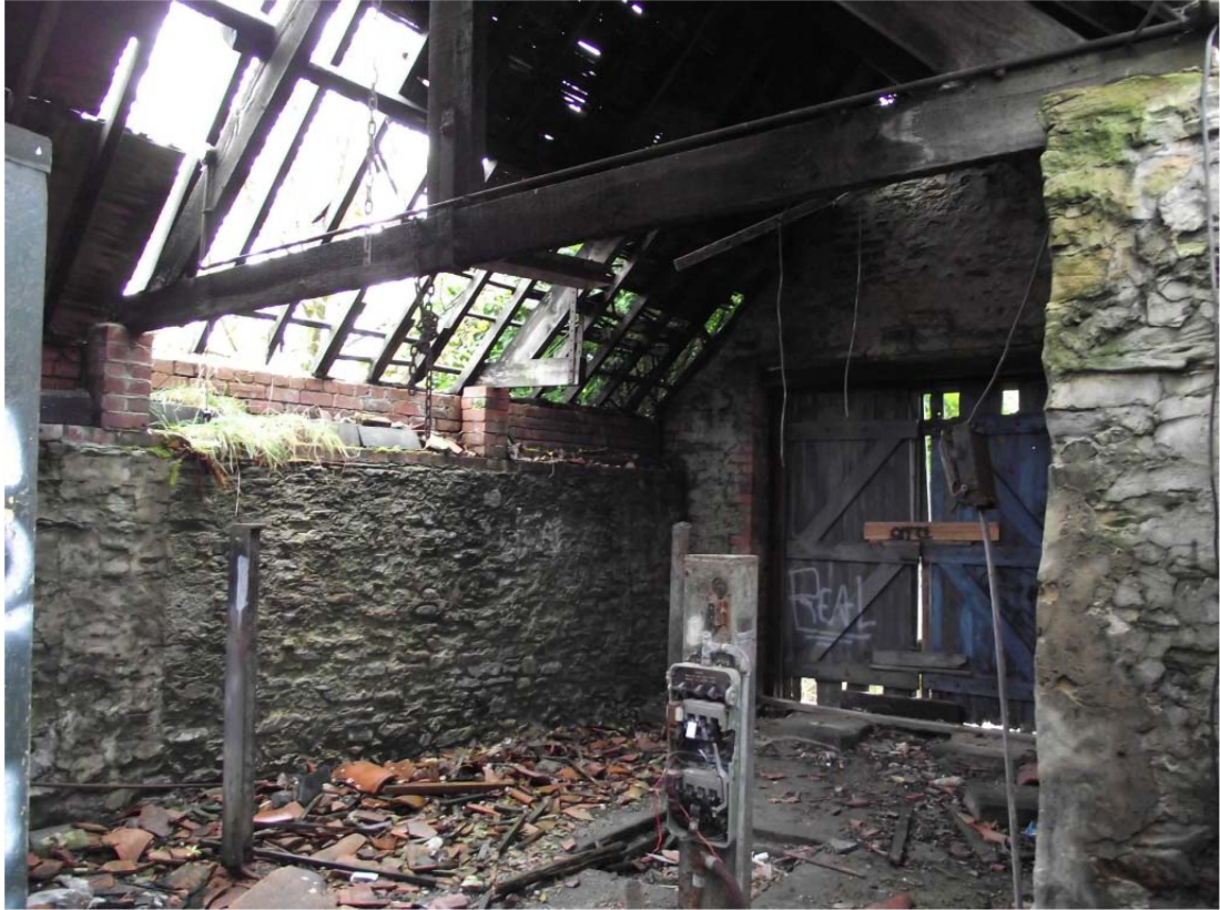
Photograph 33: North range, internal, south-eastern room, looking east (no scale)
