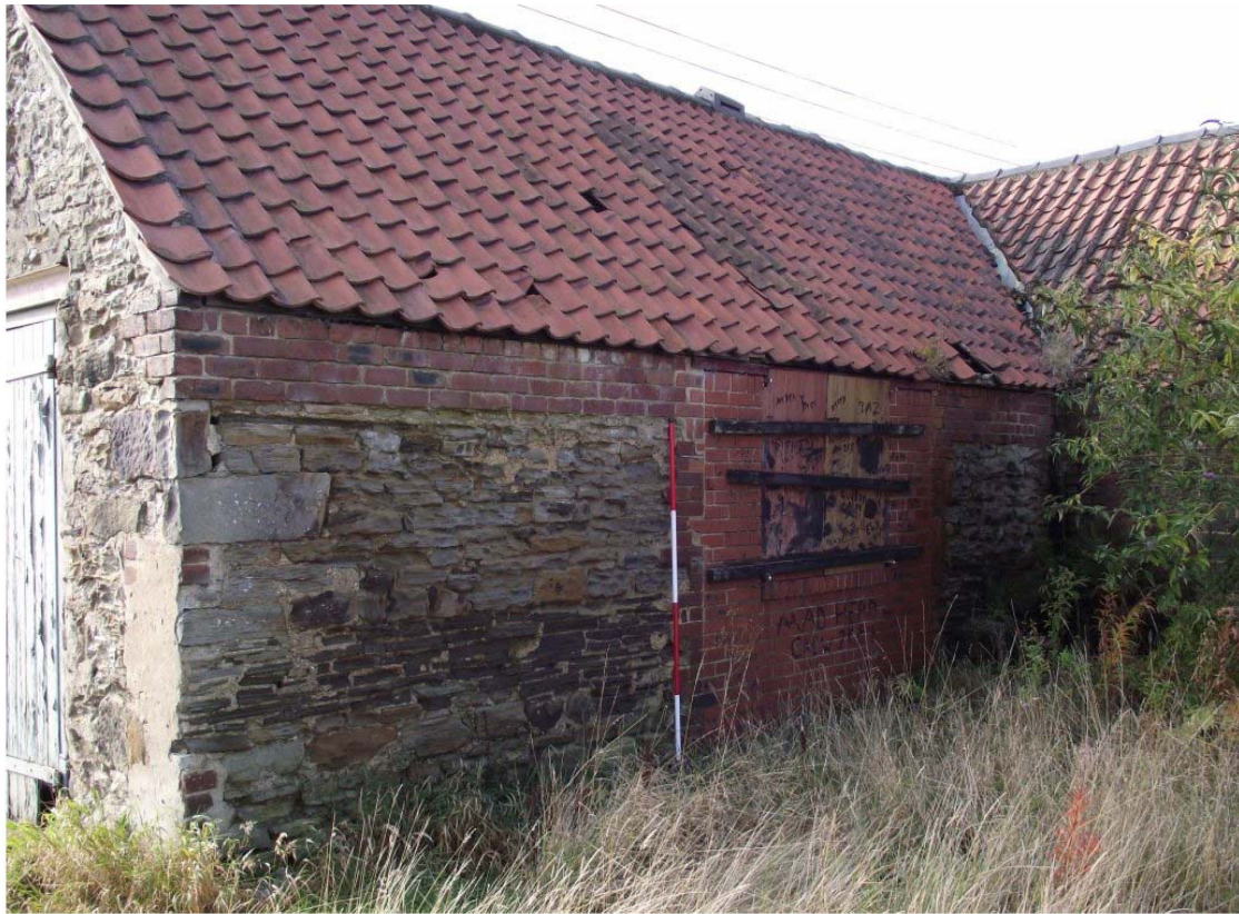
Photograph 13: South range, north-west facing elevation, oblique view (2m scale)
