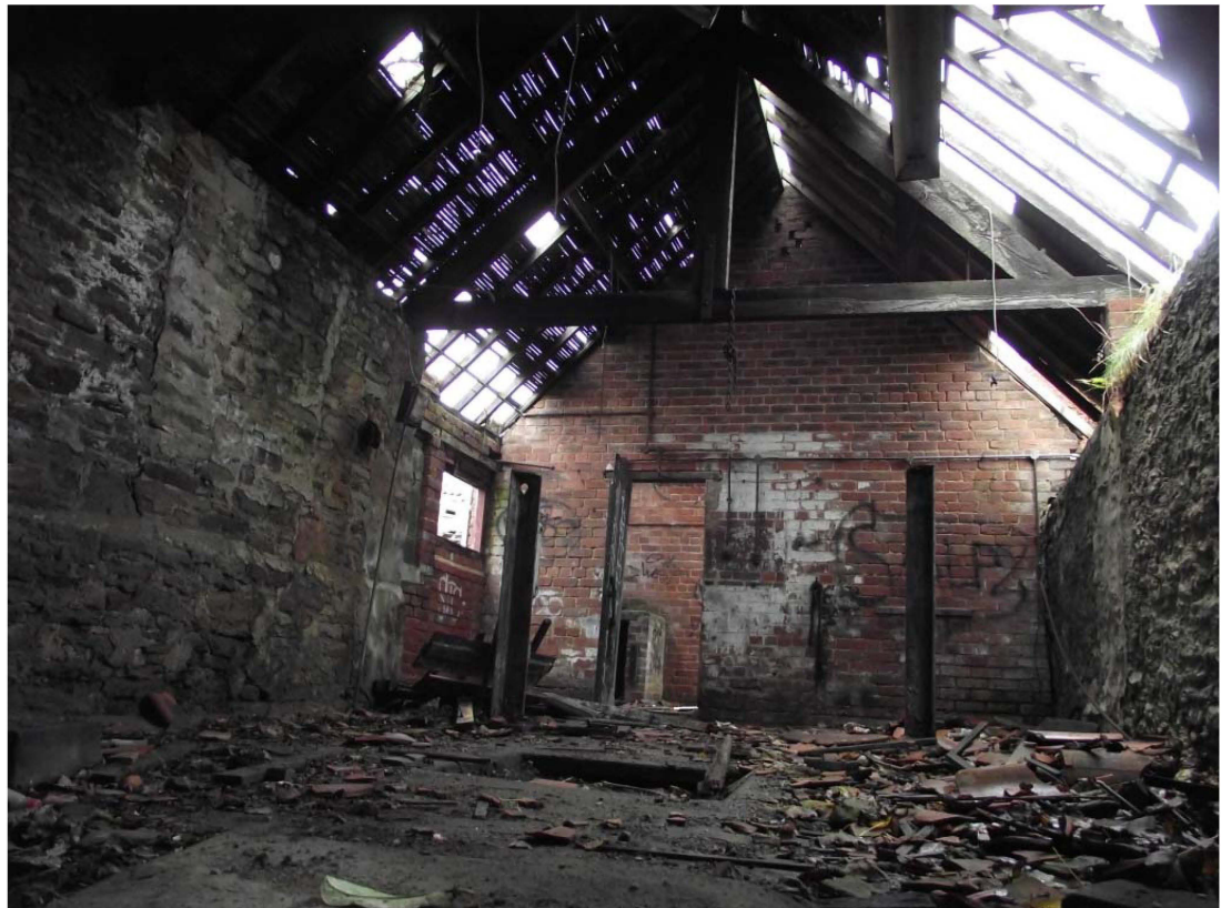
Photograph 34: North range, internal, south-eastern room, looking north-west (no scale)
