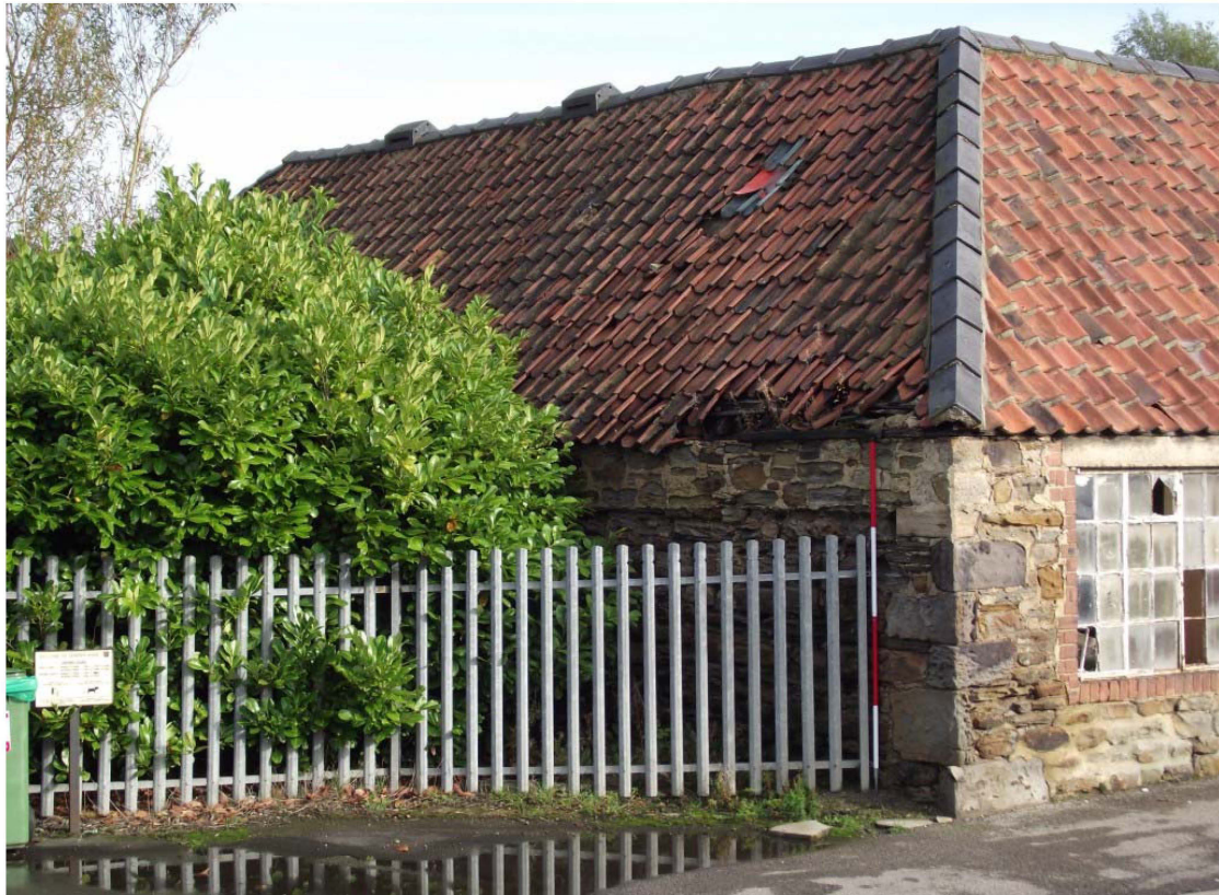
Photograph 7: West range, north-west facing elevation, south end, oblique view (2m scale)
