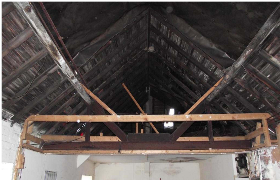
Photograph 26: South range, internal, roof space, looking north-west (no scale)
