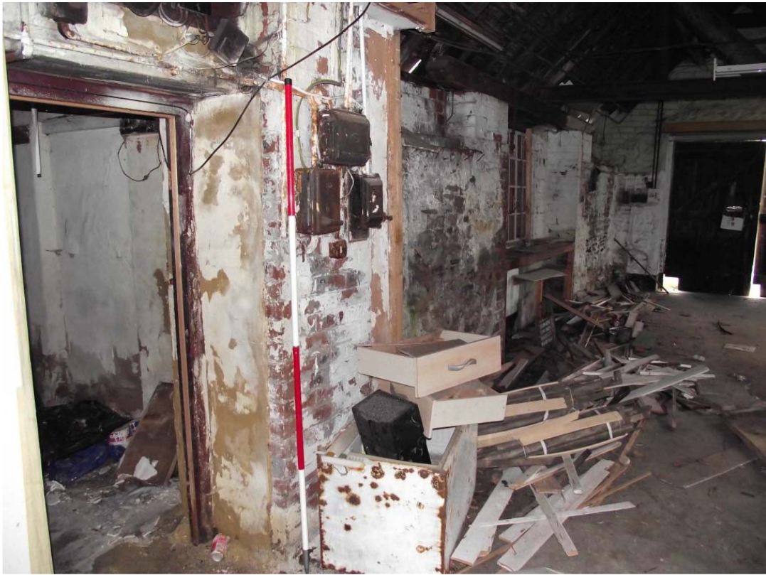
Photograph 29: South range, internal, north wall, looking east (2m scale)
