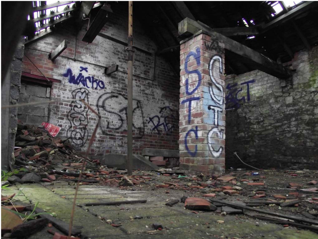
Photograph 35: West range, internal, north-eastern room, looking west (no scale)
