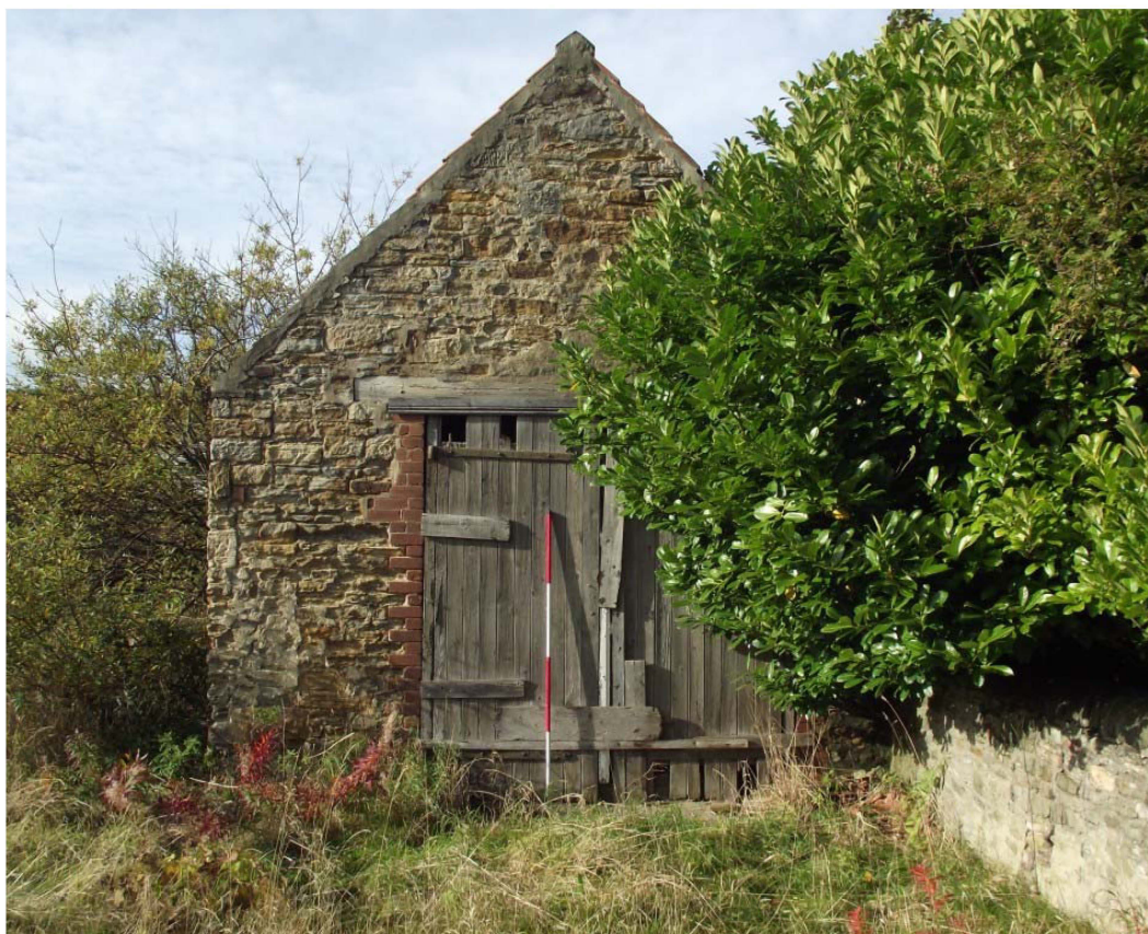
Photograph 19: North range, south-east facing gable elevation, front on view (2m scale)
