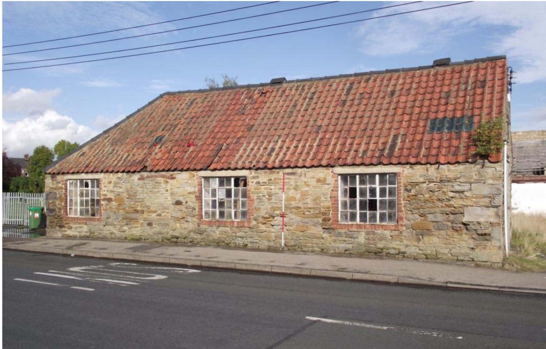
Photograph 3: South range, south-west facing elevation, oblique view (2m scale)
