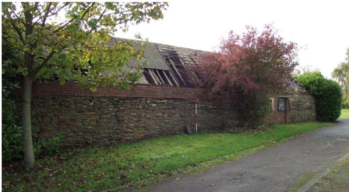
Photograph 8: North range, north-east facing elevation, oblique view (2m scale)
