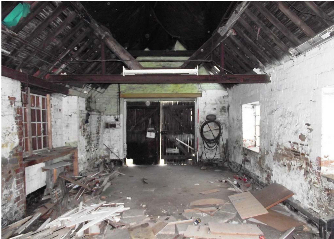
Photograph 23: South range, internal, looking south-east (2m scale)
