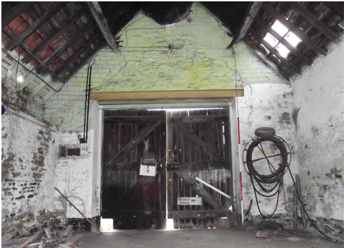
Photograph 24: South range, internal, gable-end doorway, looking south-east (2m scale)
