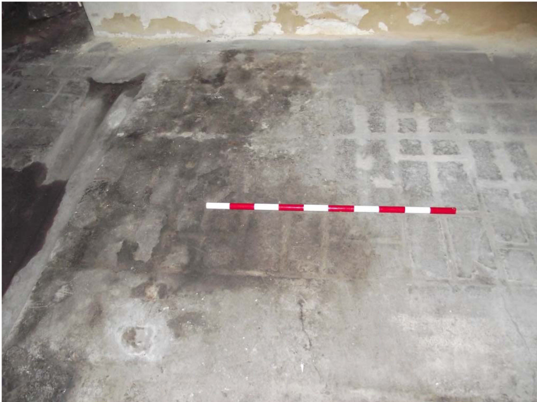
Photograph 32: West range, internal, south-western room, floor detail, looking south-west (1m scale)
