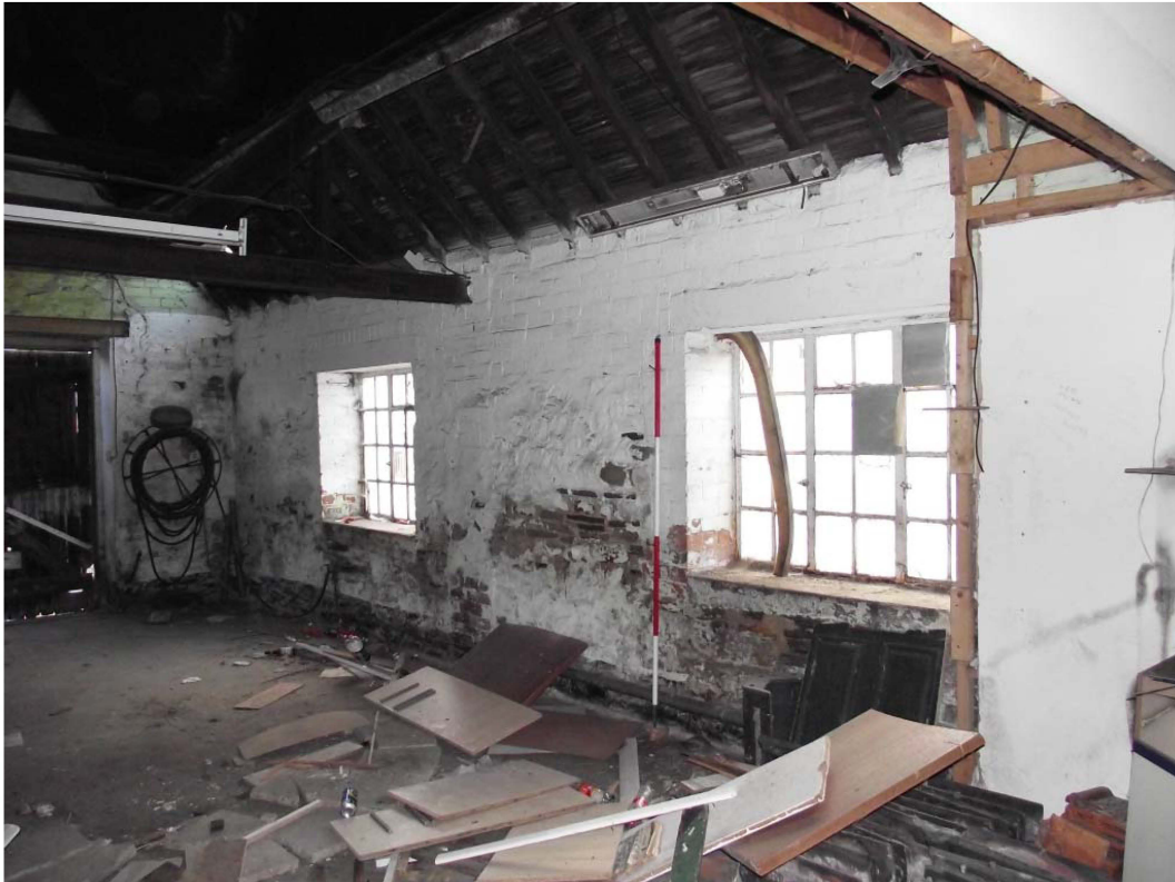
Photograph 27: South range, internal, south wall, looking south (2m scale)
