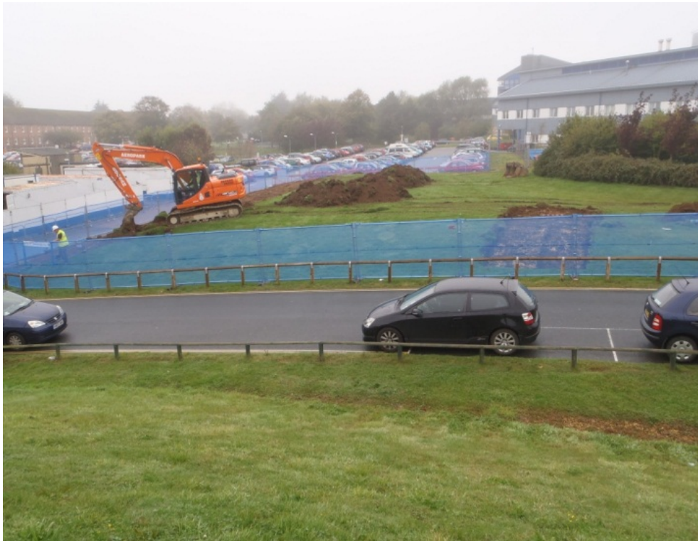
Plate 2: General view of site and stripping operation, view to west
