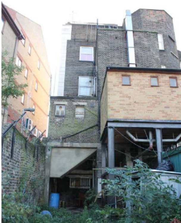
Plate 6: East side of rear elevation of the Walpole, looking south
