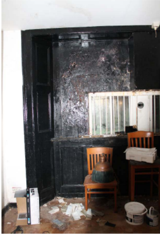
Plate 13: Basement back room of the Walpole (showing blocked window)
