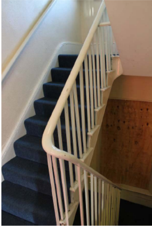
Plate 11: Original staircase, 403 New Cross Road
