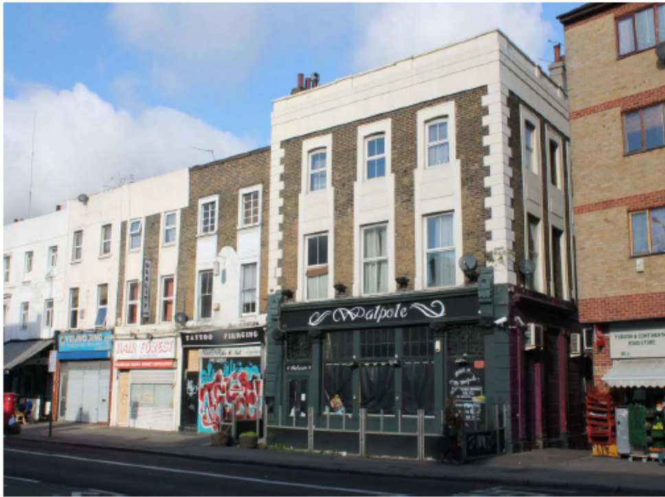
Plate 1: Front elevations of the Walpole (407) and 403-405 New Cross Road, looking north-west
