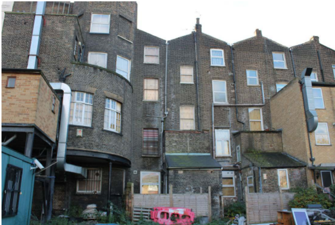
Plate 4: Rear elevations of 403 and 405 New Cross Road, looking south
