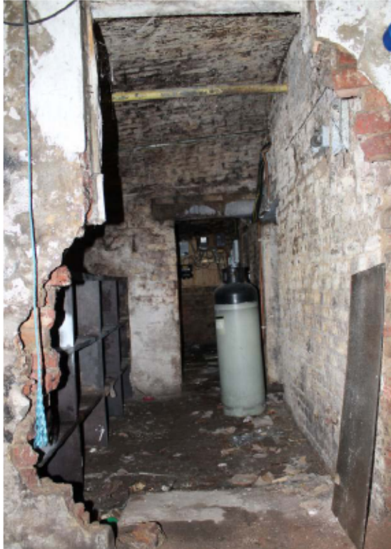
Plate 14: Vaulted cellars along road frontage
