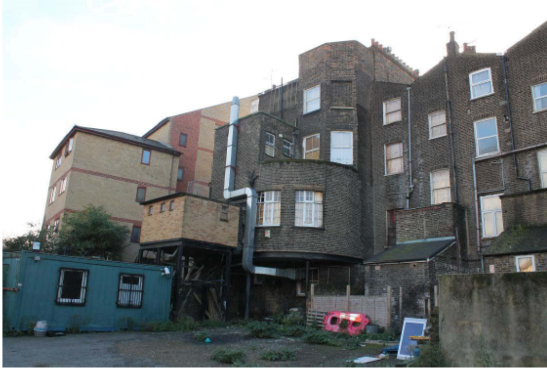
Plate 3: Rear elevations of the Walpole, looking south-east
