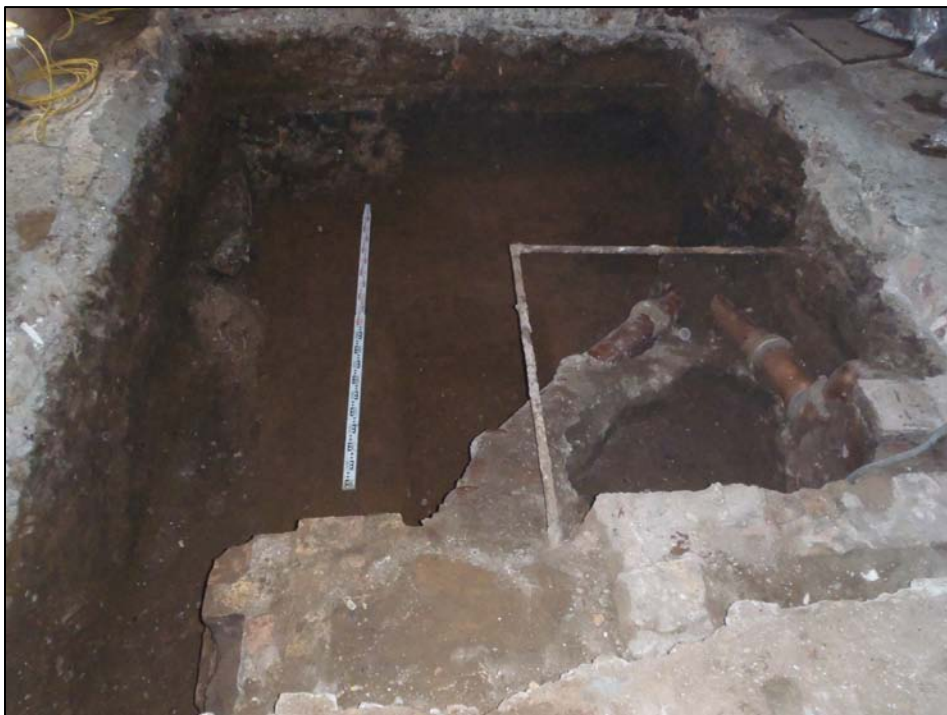
Plate 1: Overview of Trench 1, looking NE
