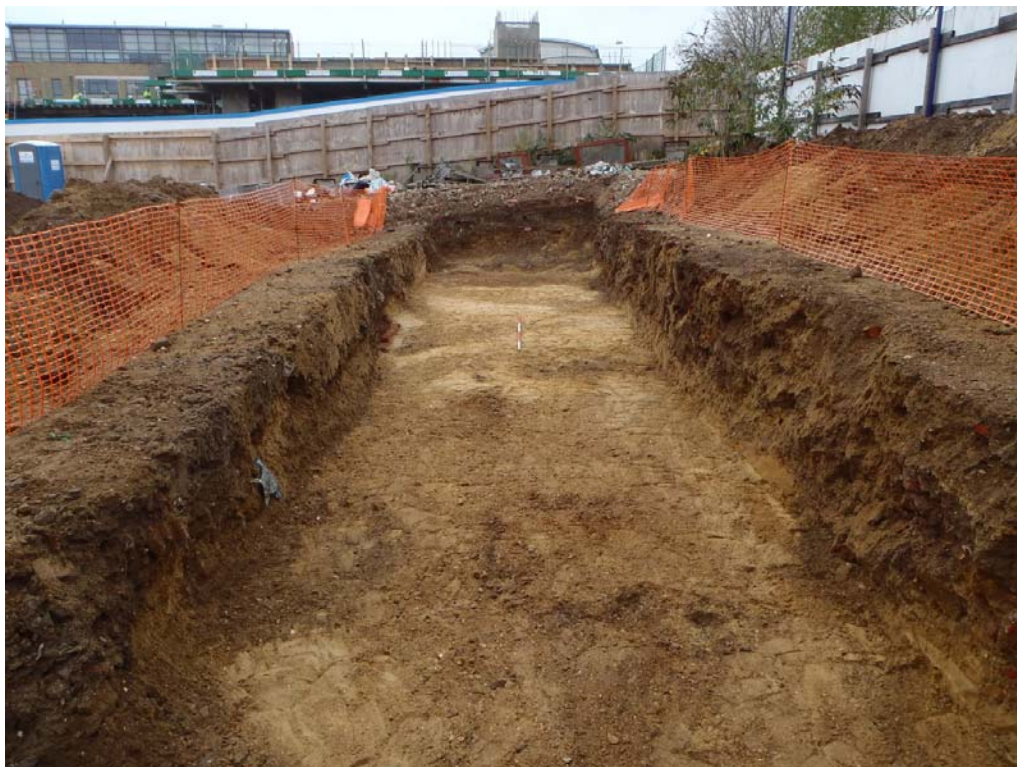
Plate 10: Trench 2 looking southwest
