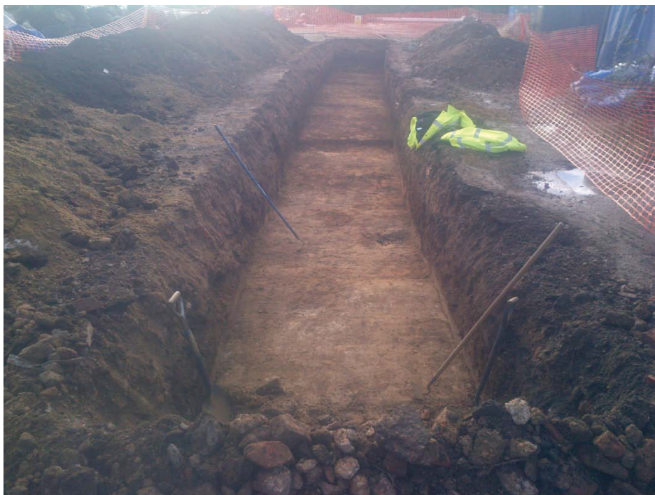
Plate 1: Overview of Trench 1, View to the South
