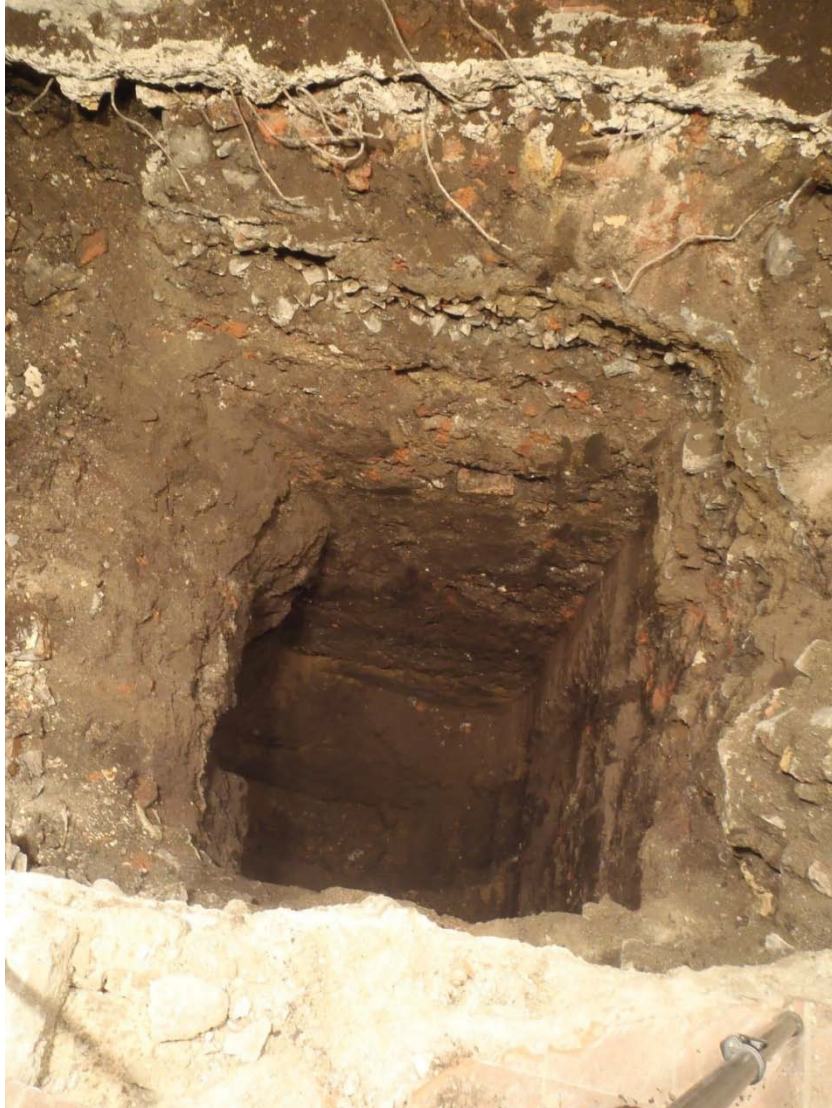
Plate 7, Trench 3, Section 3, facing south
