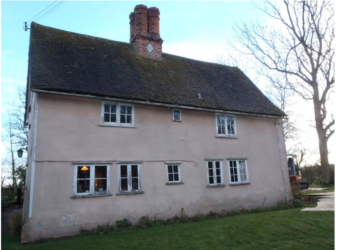
Plate 2: Moat Farm House, west elevation
