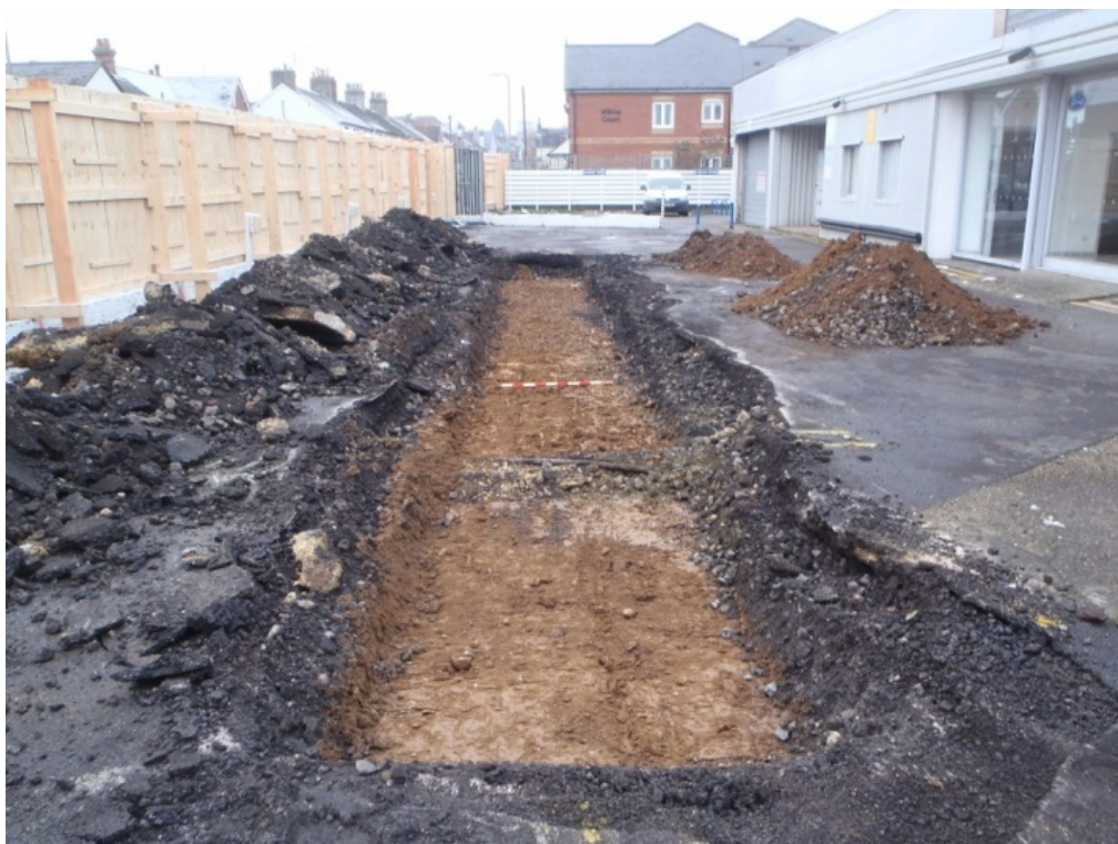
Plate 2: Trench 2: General view to north-west. Scale 1m.
