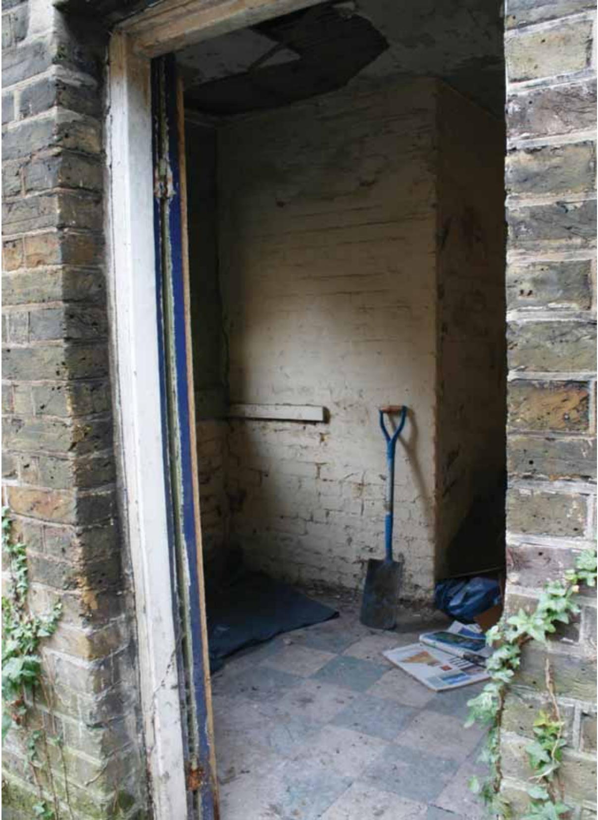
Plate 12: Kitchen of 204, Grange Road, looking east (PCA Archive no. GBR12 D100 (19))
