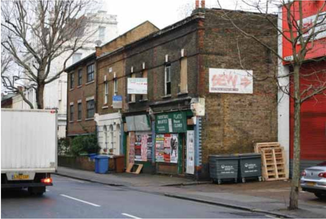
Plate 1: Front (south) elevation of 204 (right) to 206 and Marks Court, Grange Road, looking north-west (PCA Archive no. GBR12 D100 (2))
