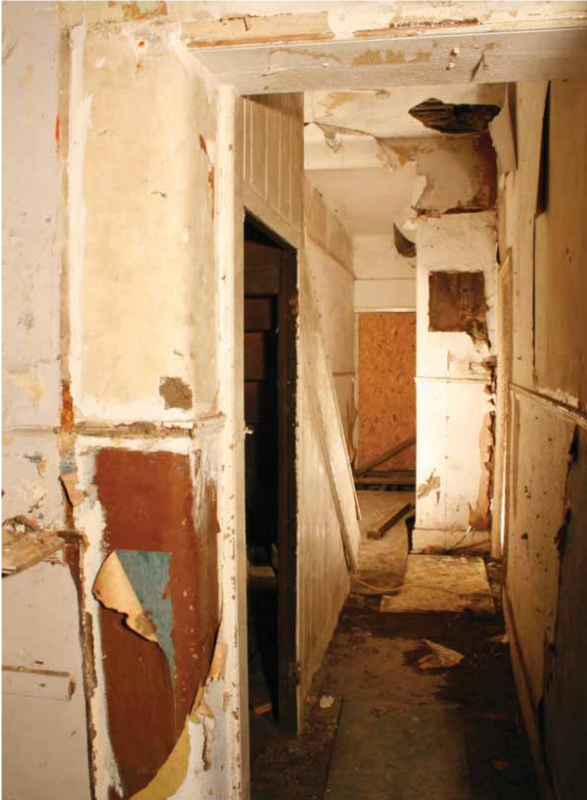
Plate 9: Hall of 204, Grange Road, looking south (PCA Archive no. GBR12 D100 (20))
