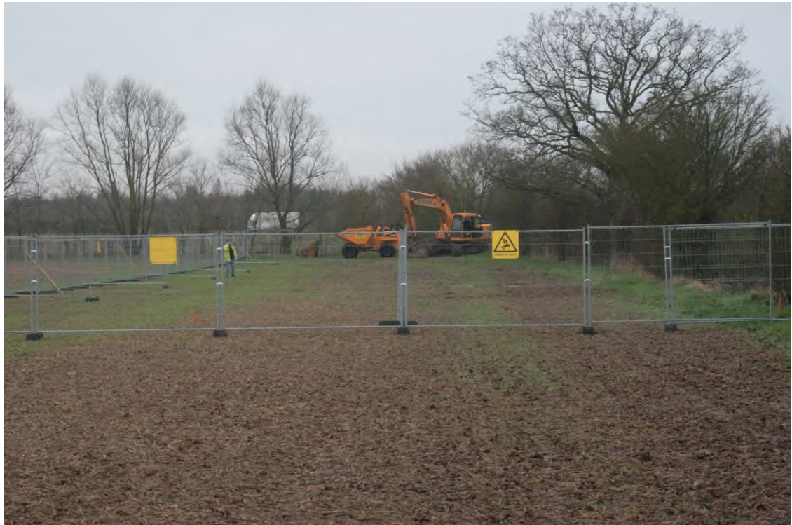
Plate 1: Site prior to stripping operations looking south.
