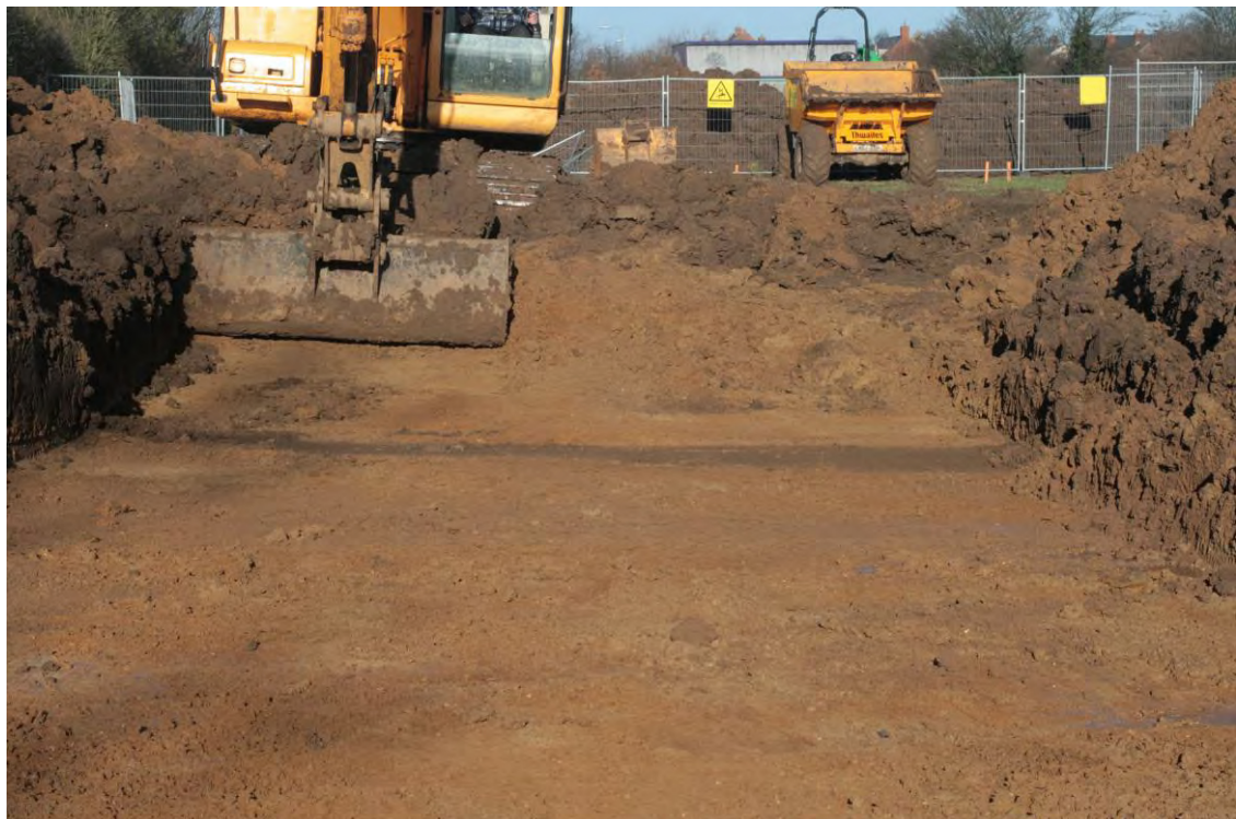
Plate 2: Soil stripping operations showing ditch [1] and hedgeline [3] in foreground.
