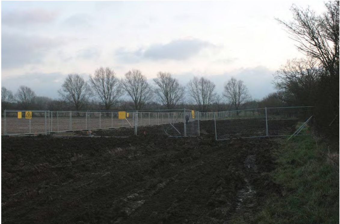
Plate 3: Site following reinstatement of sub- and topsoil.
