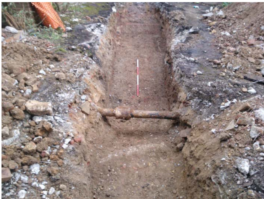
Plate 2: Post-Ex shot of Trench 2 (facing south-west)
