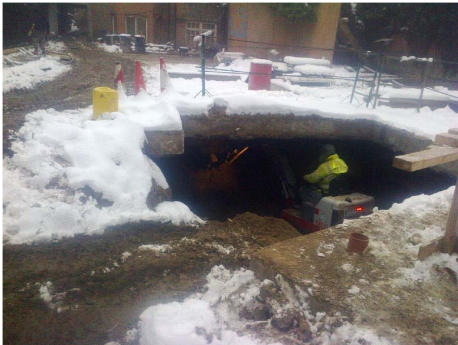
Plate 3: Excavation for basement following casting of slab, view to northeast
