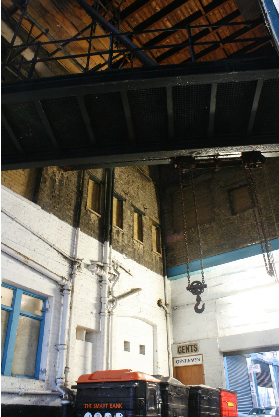
Plate 24: Overhead bridge within passageway, looking north (72FmLa D100 051)
