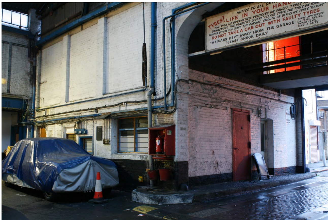
Plate 34: Internal view of the passageway entrance from Farm Lane into the building, looking south-west (72FmLa D100 057)
