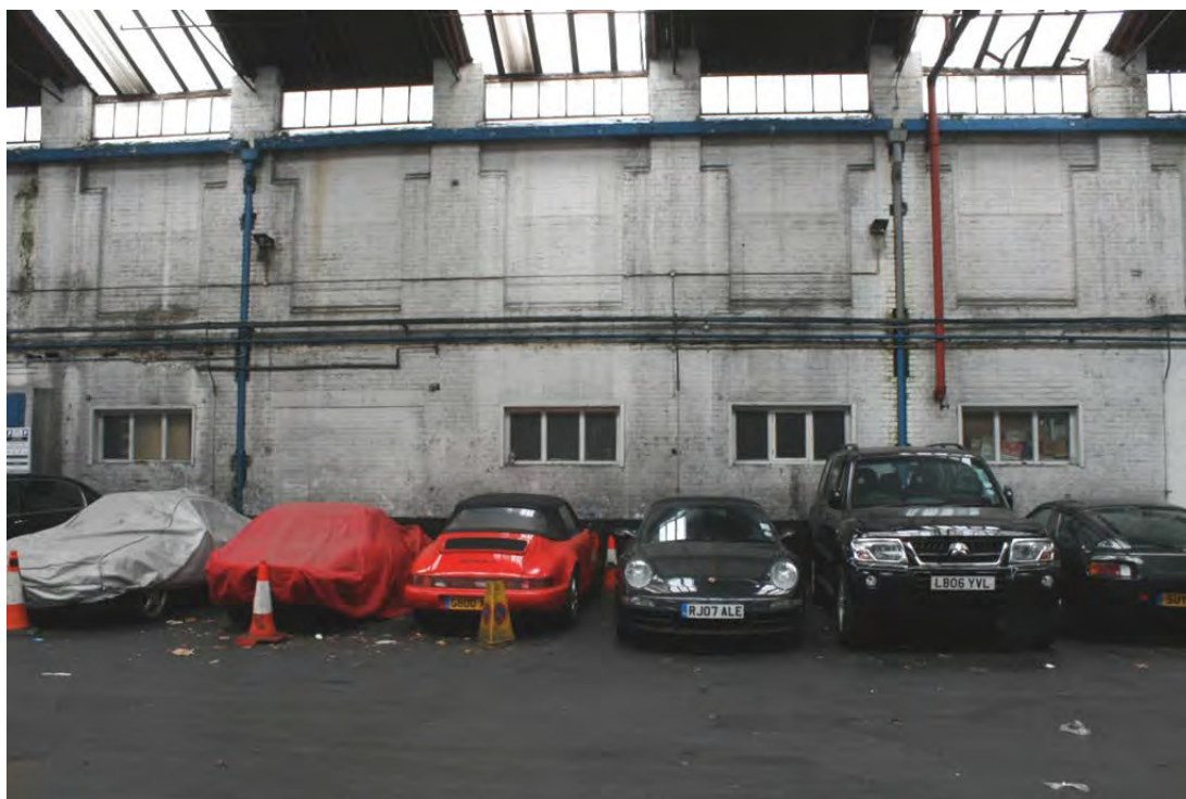
Plate 29: Inserted ground floor windows and blocked double doorway on the north side of building, looking north-west (72FmLa D100 033)
