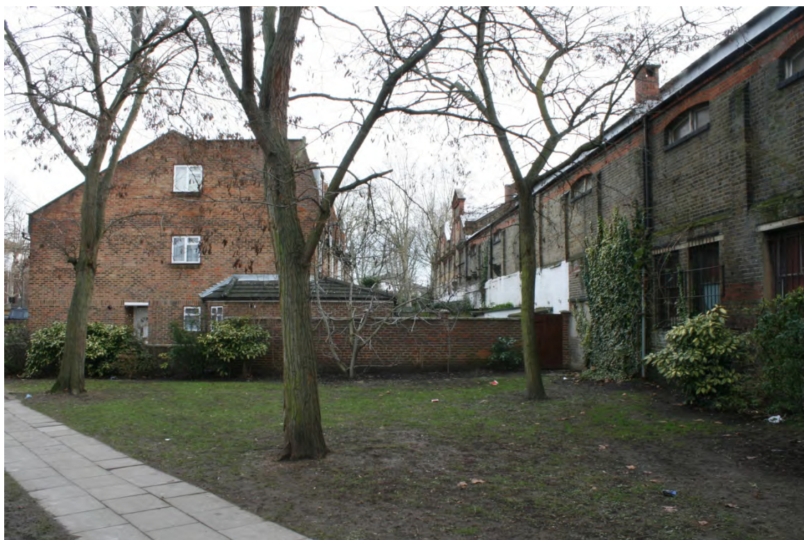
Plate 8: North-east end of long north-west elevation opposite private rear gardens, looking east (72FmLa D100 07a)
