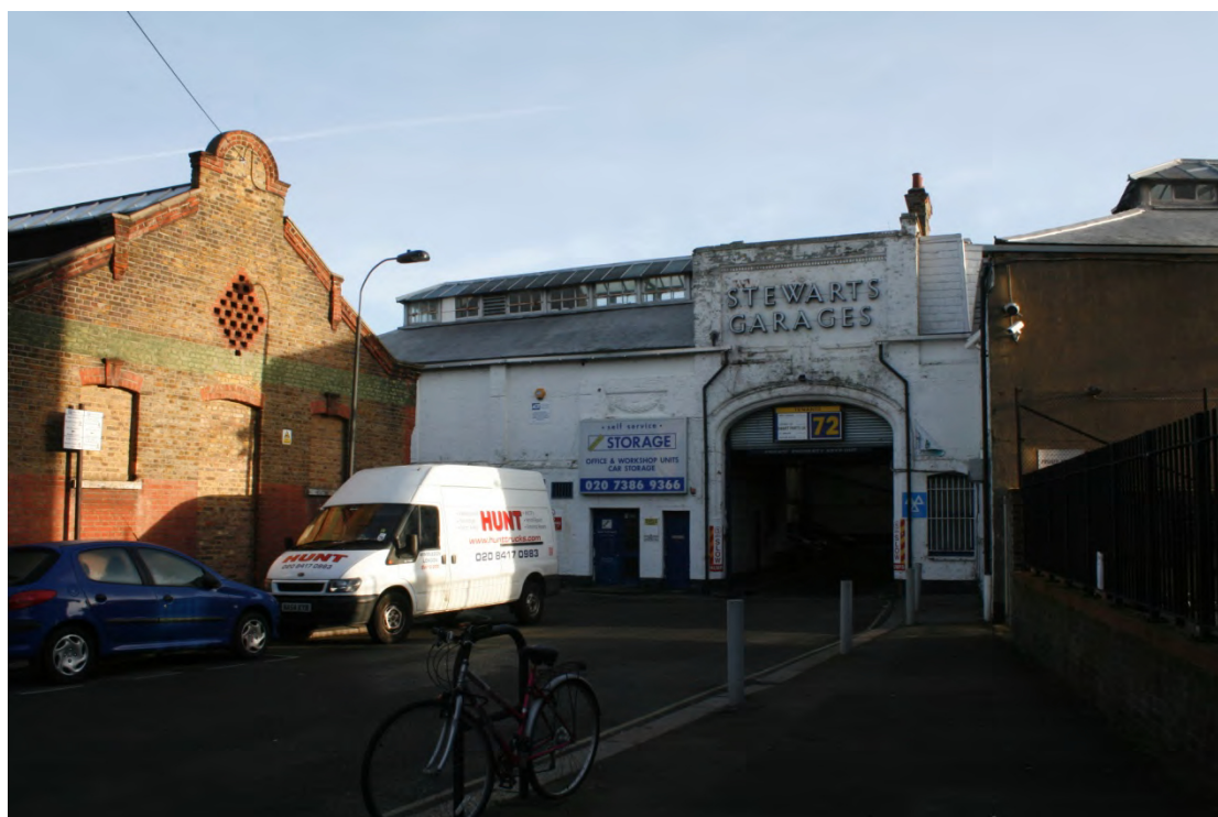
Plate 1: South-west facade with entrance from Farm Lane, looking north-east (72FmLa D100 001)
