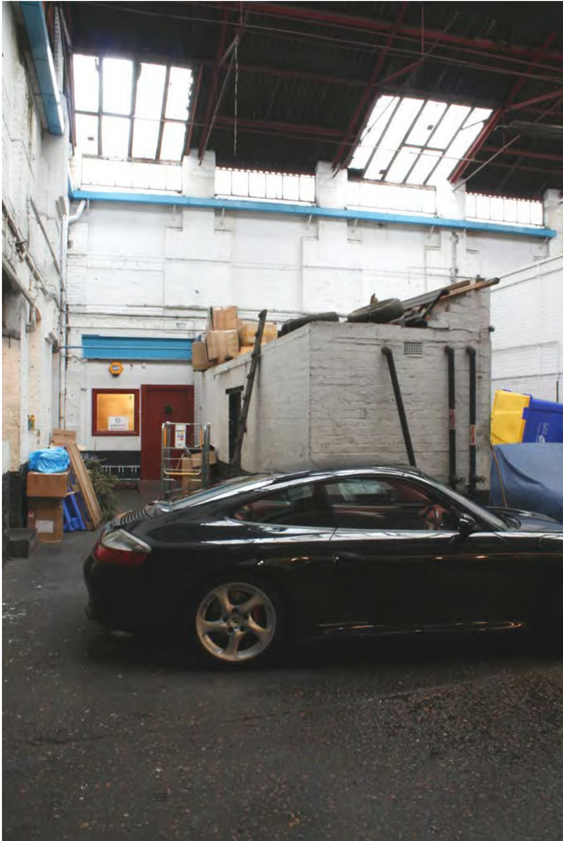
Plate 20: Skylights in the main workshop area of the garage, looking north-west (72FmLa D100 026)
