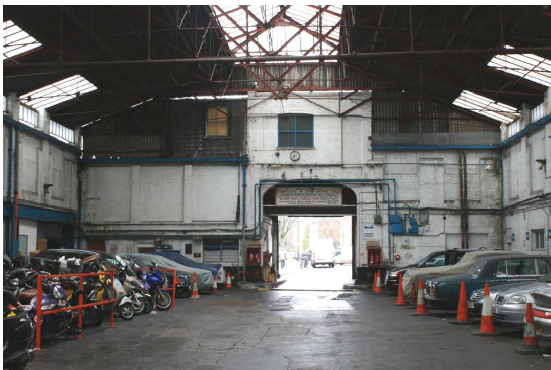
Plate 33: Internal view of the passageway entrance from Farm Lane into the building, looking south-west (72FmLa D100 041)
