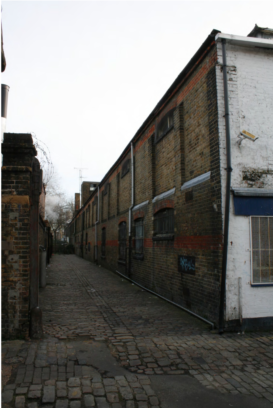
Plate 5: Long north-west elevation (right) and adjacent alleyway, looking north-east (72FmLa D100 04)
