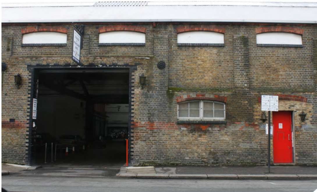
Plate 11: Inserted entrance in north-east elevation from Seagrave Road, looking south-west (72FmLa D100 010)
