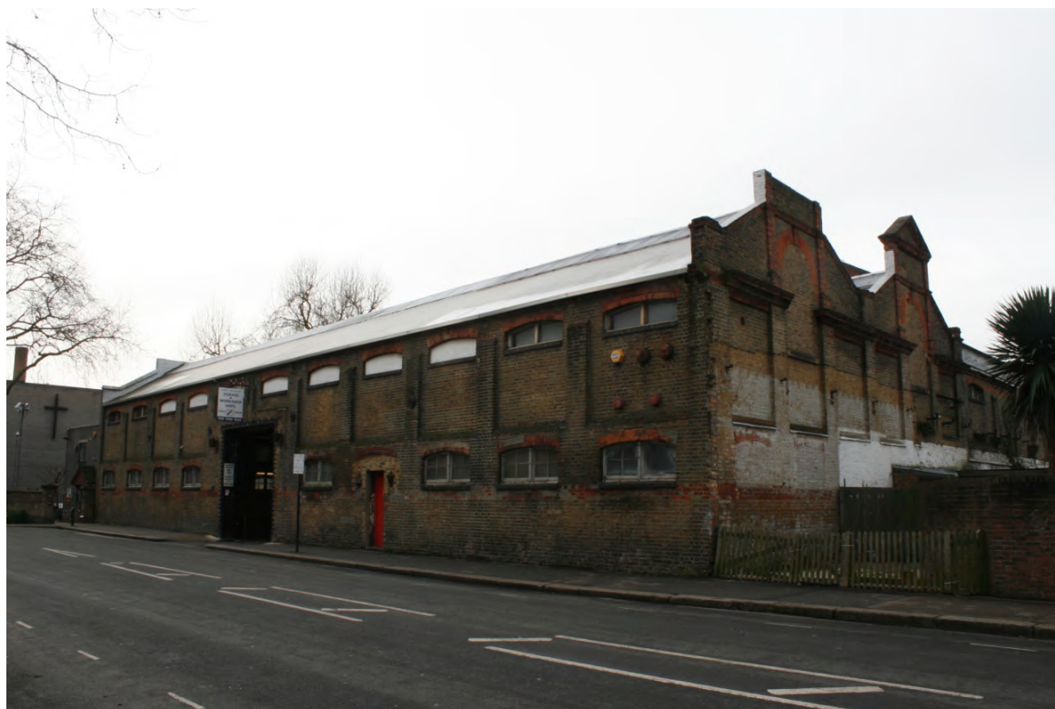
Plate 9: North-west (right) and north-east (left) elevations and Seagrave Road, looking south-west (72FmLa D100 008a)
