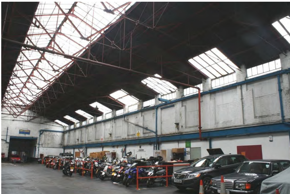
Plate 31: New workshops on the south side of the building, looking east (72FmLa D100 037)
