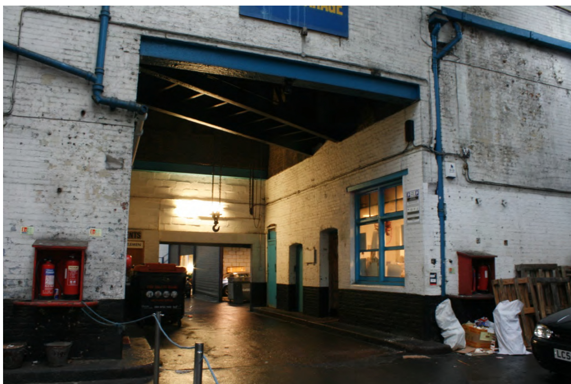
Plate 26: Passageway entrance from the parking area at the south-west end of the building to the main workshop area beyond, looking south-east (72FmLa D100 054)
