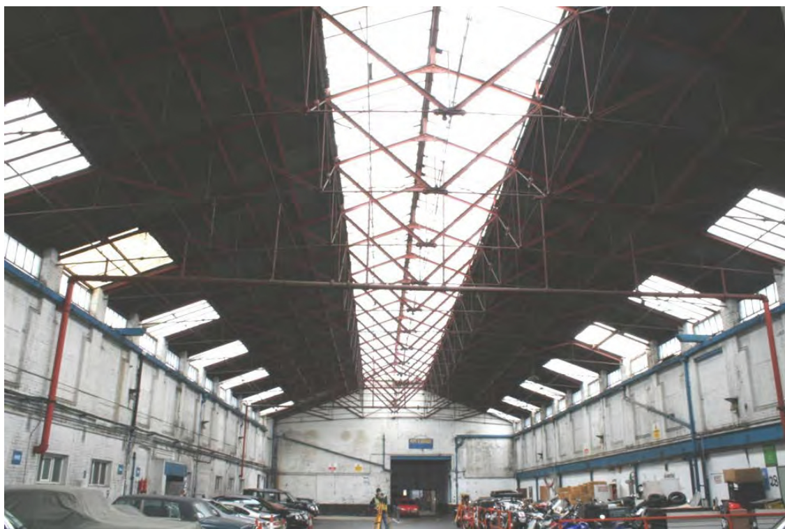
Plate 27: Parking area at the south-west end of the building, looking north-east (72FmLa D100 031a)
