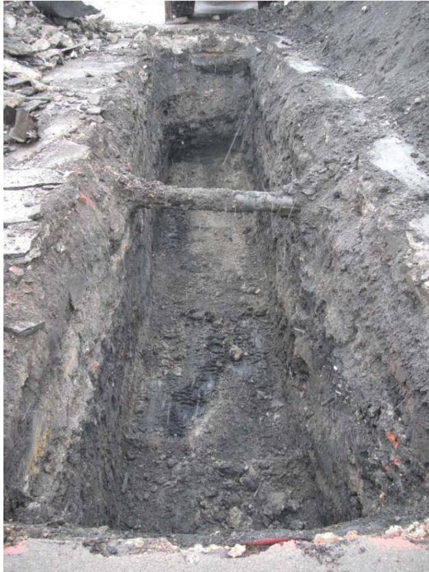
Plate 1: South-West facing view of excavated trench
