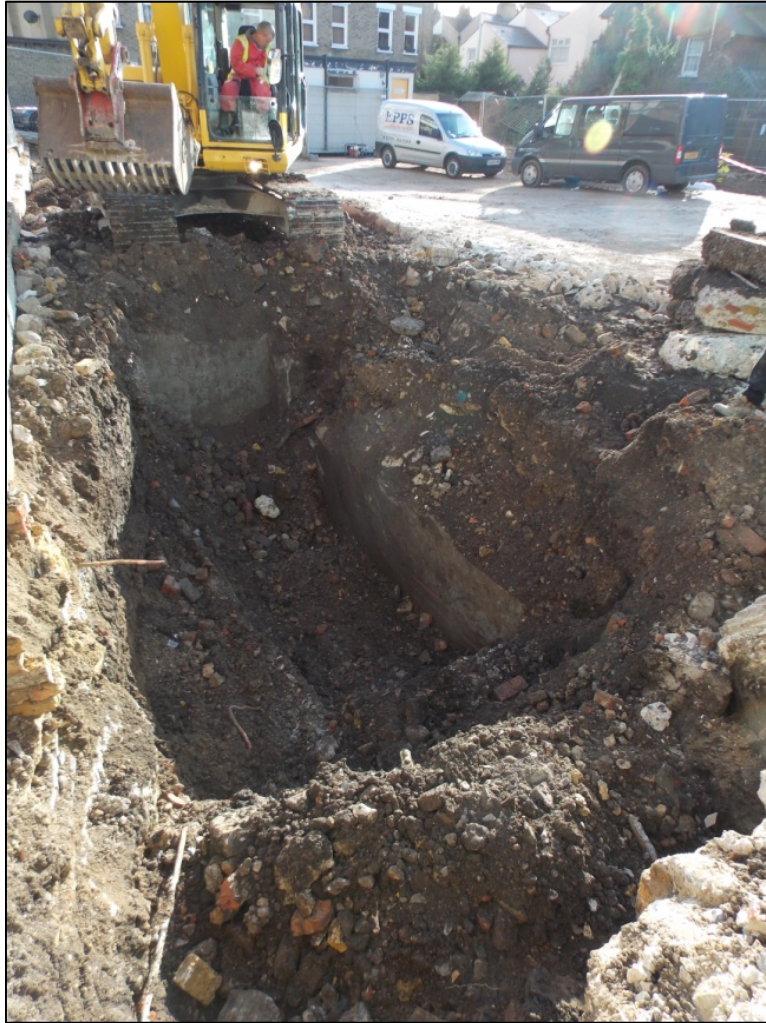
Plate 1 - Basement chamber [8] and backfill [14]
