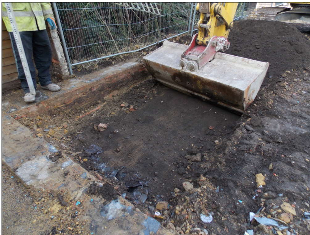
Plate 2 - Excavation of SW corner of building [1]
