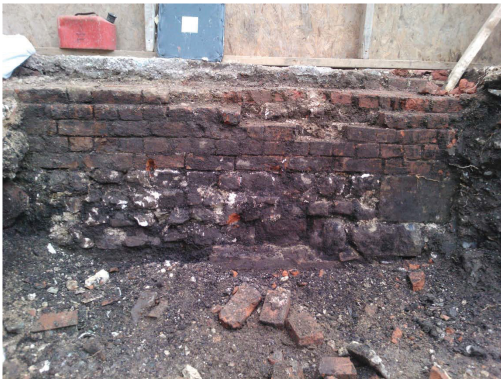
Plate 5: South facing view of wall [14] in Trench 2
