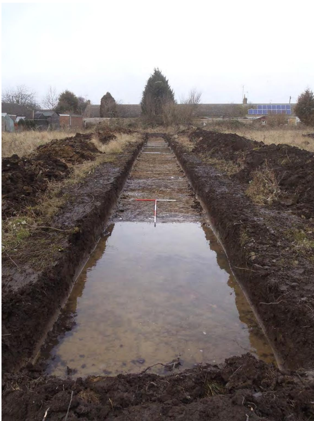
Plate 2: Trench [2], view north-west. The ditch in the foreground was not excavated as it was rapidly covered by rising water after the trench was opened.
