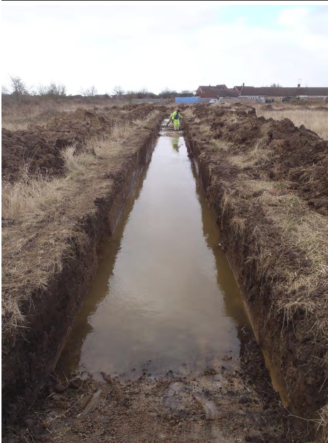
Plate 11: Trench [5], view south-west showing flooding
