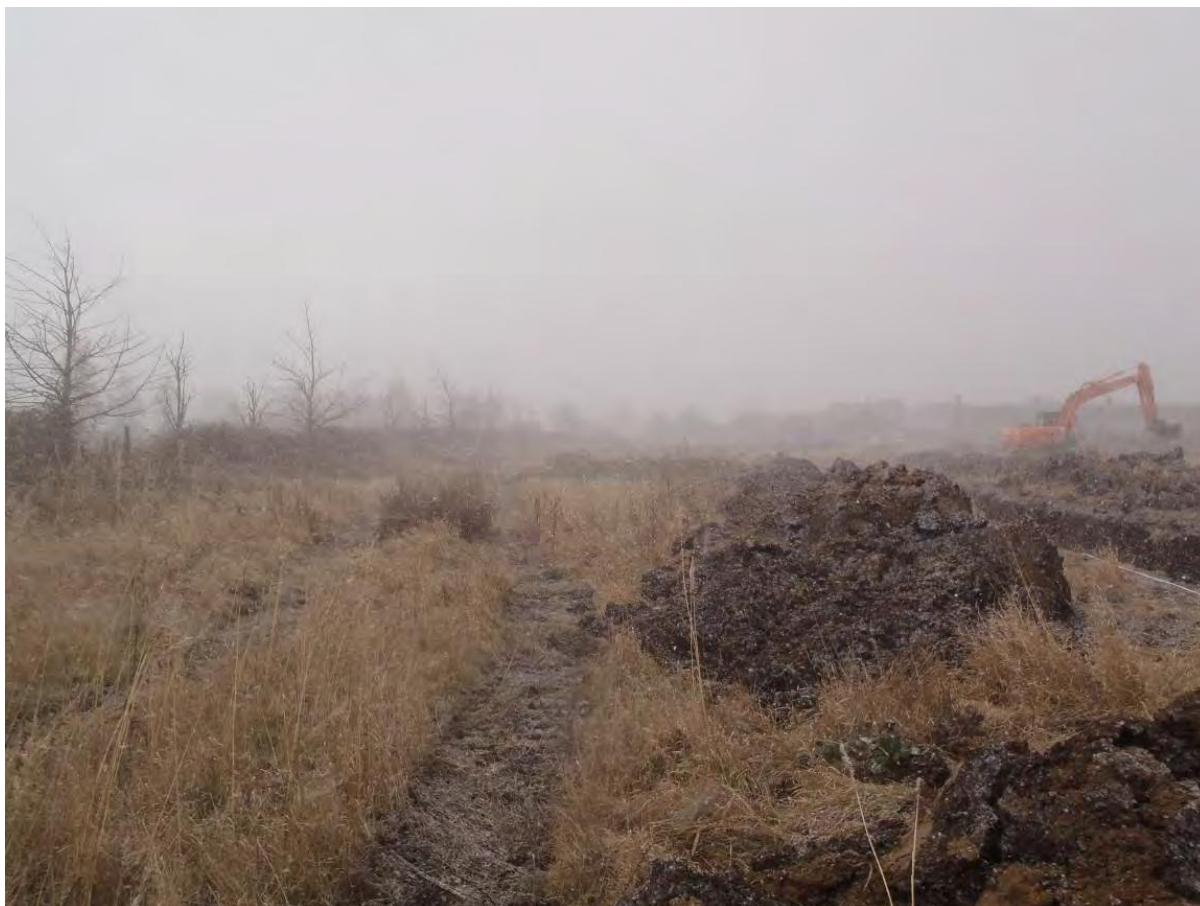
Plate 7: The site, view south-east downslope from north-east
