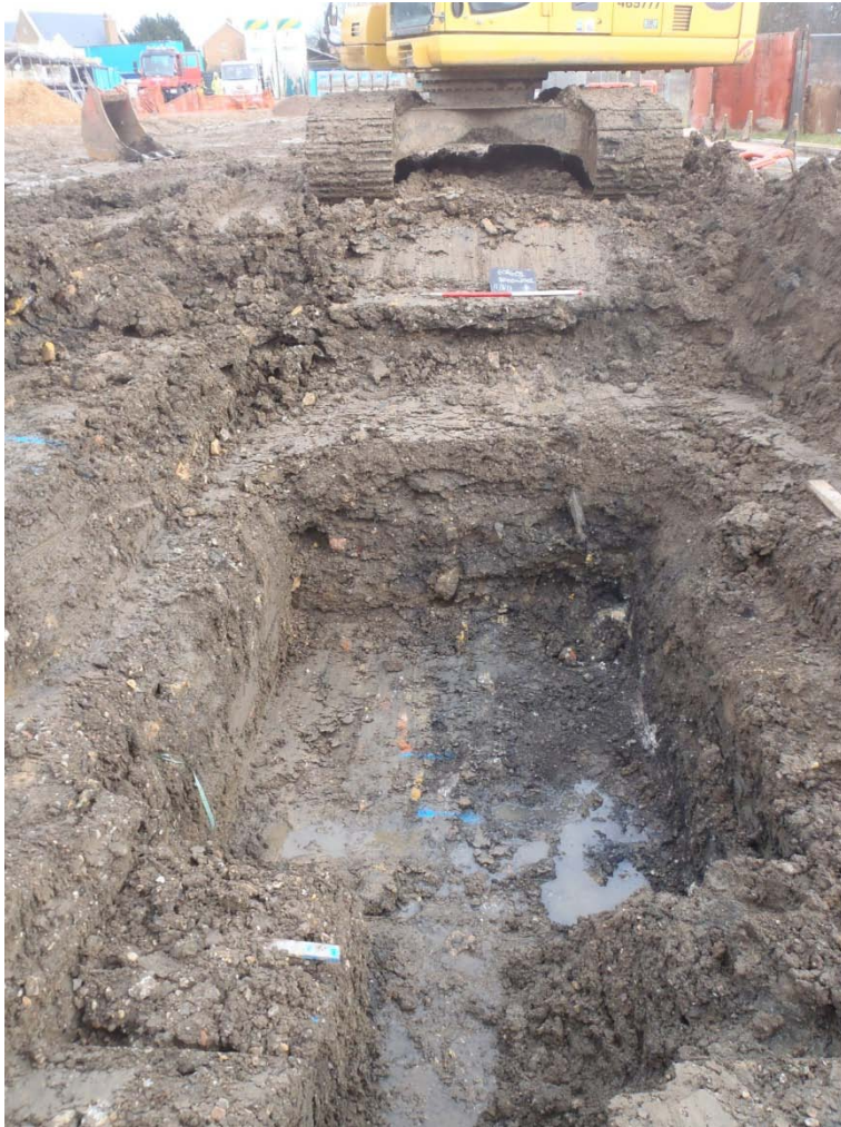
Plate 4: Photo of trench for manholes showing layer [3000], view facing north east.
