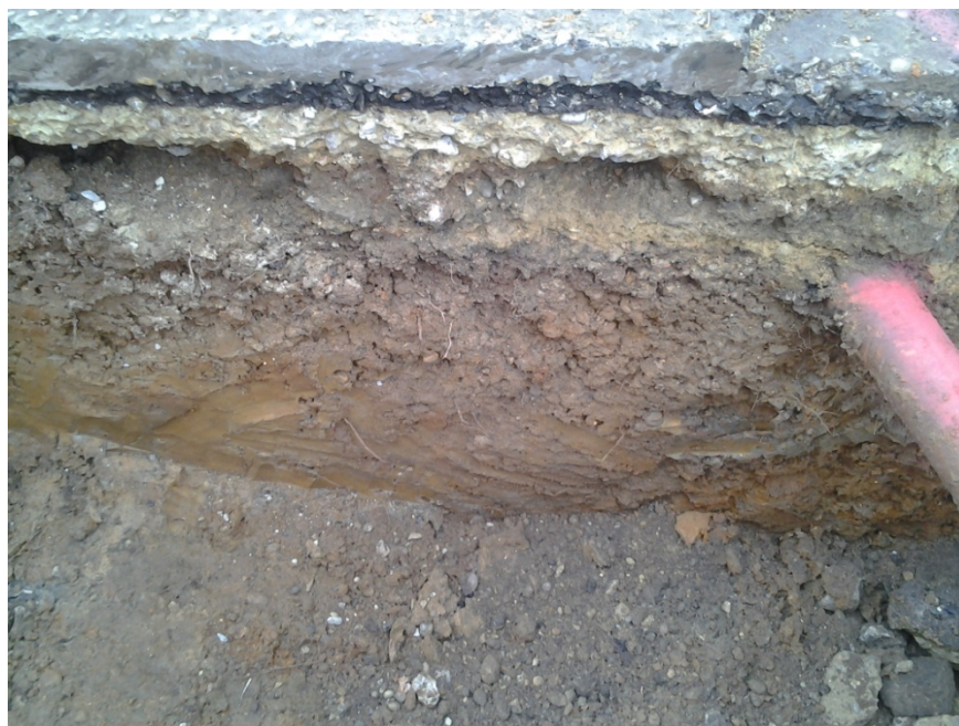
Plate 4: Section through road
