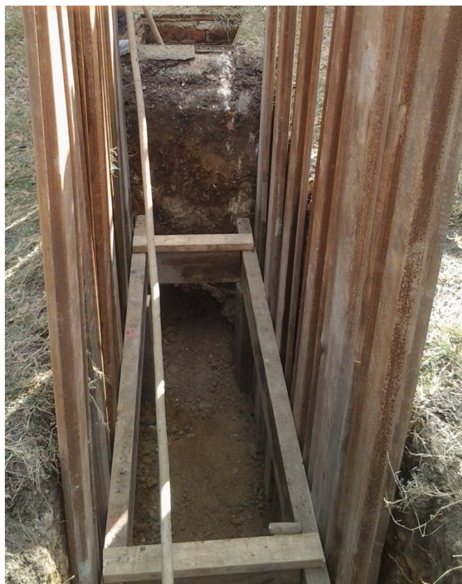
Plate 1: Trench looking east
