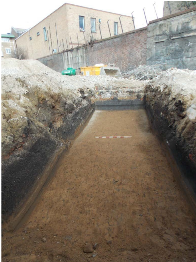
Plate 3: Overview of Trench 3, facing northwest, 1m Scale
