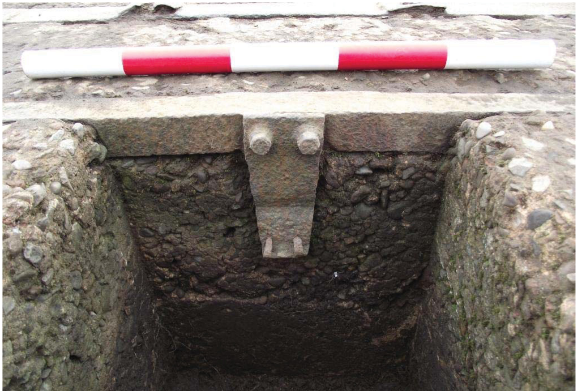
Figure 35. LAA gun pedestal, metal frame, stirrup bracket detail, looking north ( 0.5m scale )
