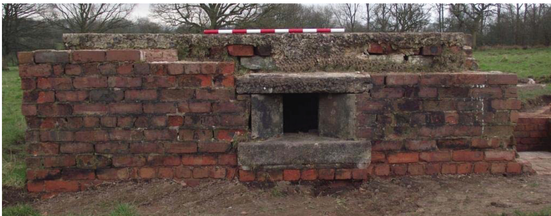
Figure 18. Pillbox, north-west facing elevation (1m scale)
