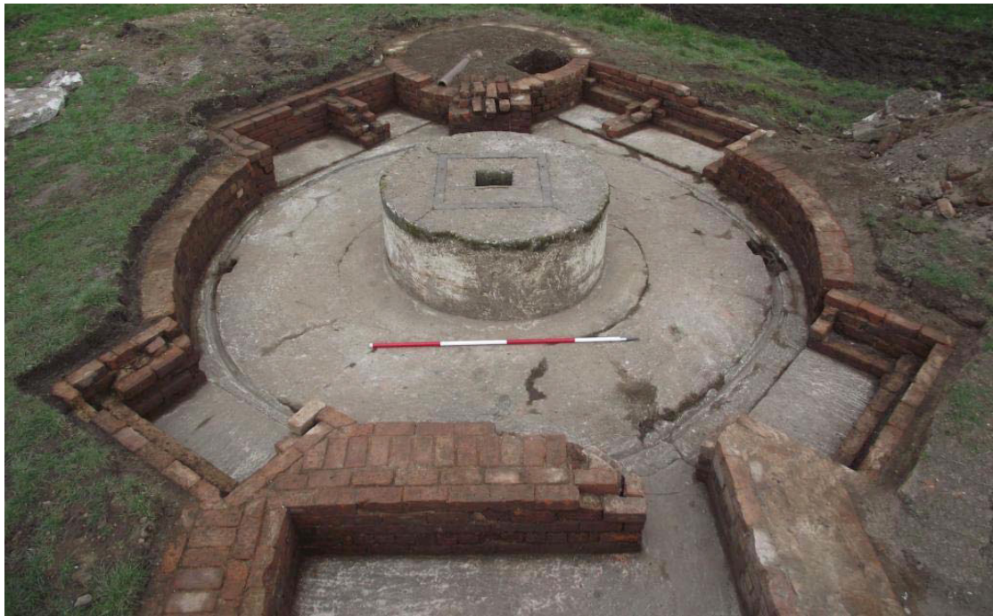
Figure 11. LAA gun emplacement, from pillbox roof, looking south-west (2m scale).
