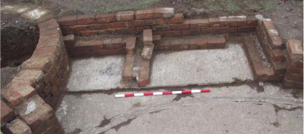
Figure 28. LAA emplacement, south-west ammunition bay, [11], looking WSW (1m scale)
