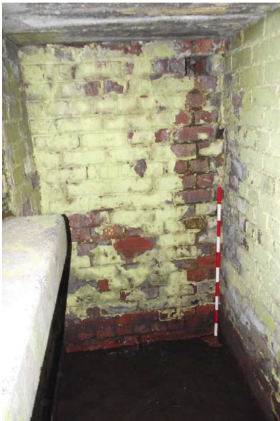
Figure 24. Pillbox, interior, south-west and anti-cochet walls, looking south-west (1m scale)
