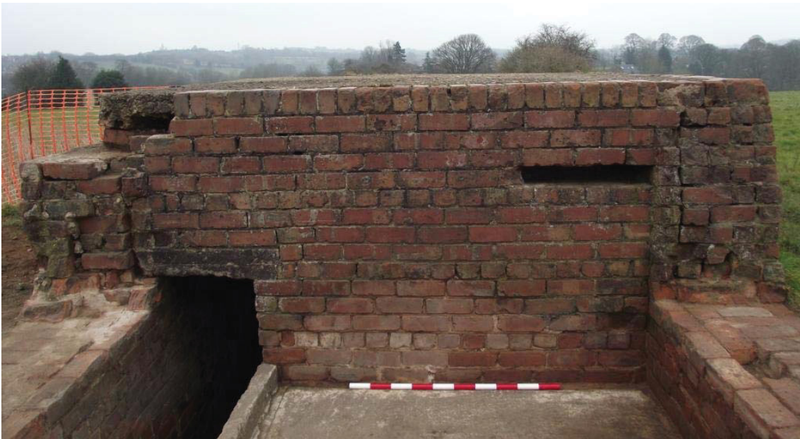
Figure 15. Pillbox, south-west facing elevation, into LMG platform ( 1m scale )
