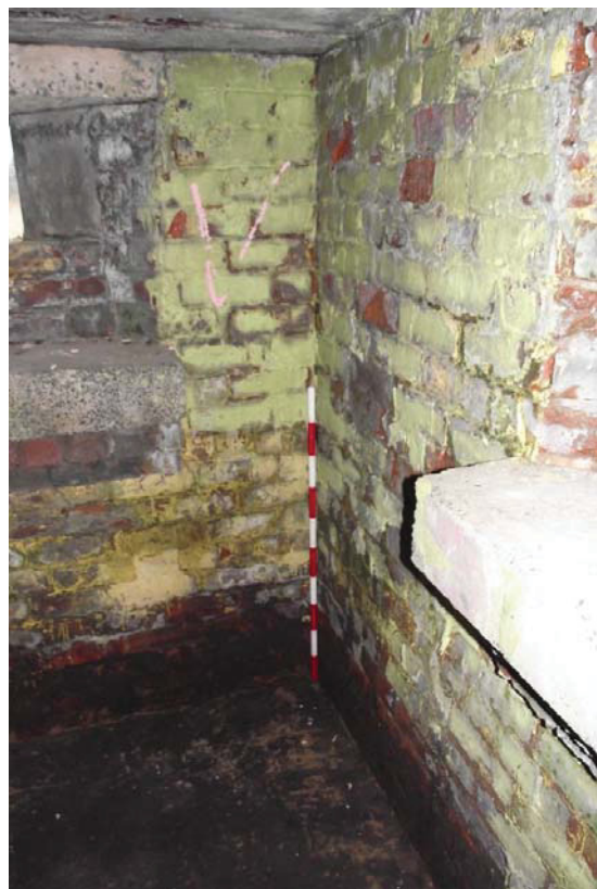
Figure 25. Pillbox, interior, north-east corner, looking north-west (1m scale)
