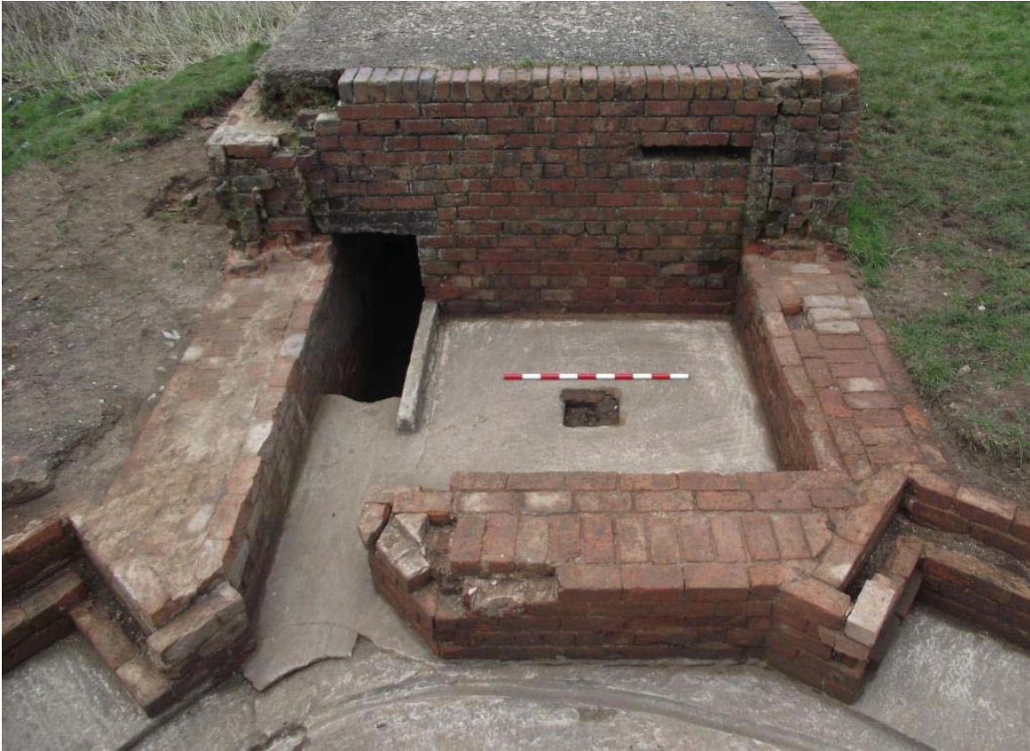
Figure 14. Pillbox and LMG platform, looking north-east ( 1m scale )
