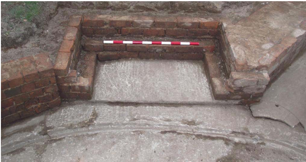
Figure 29. LAA emplacement, north-west ammunition bay, [8], looking NNW (1m scale)
