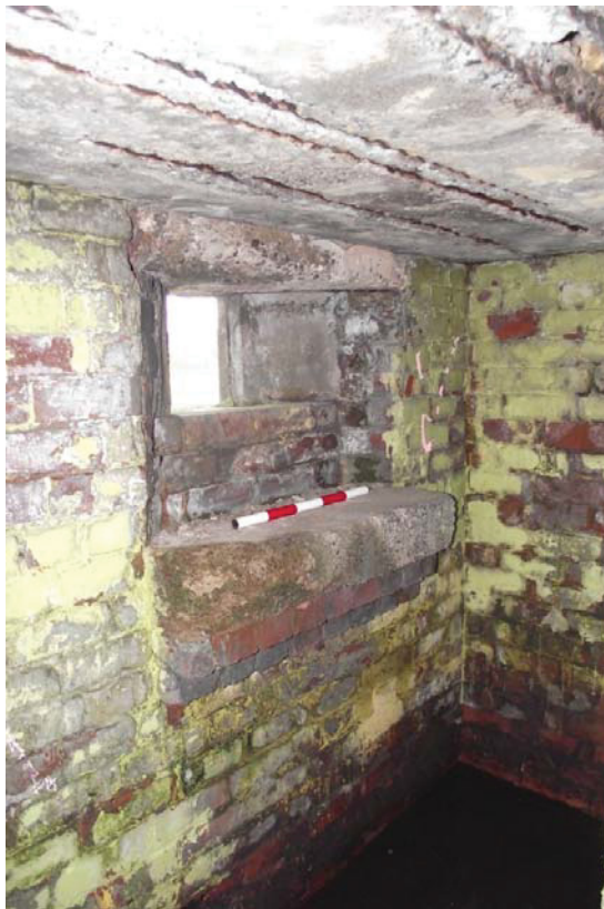
Figure 22. Pillbox, interior, embrasure in north-west wall, looking north (0.5m scale)
