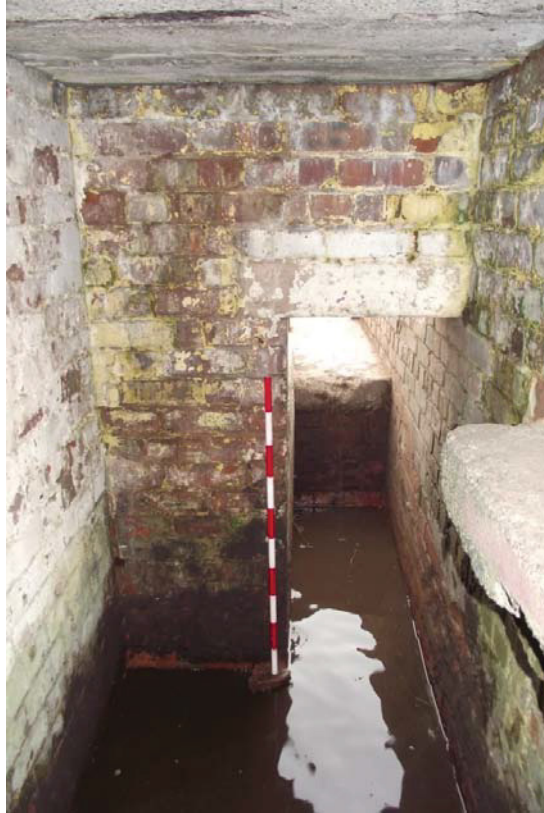
Figure 21. Pillbox, interior, entrance, with anti-ricochet wall to left, looking south-west (1m scale)
