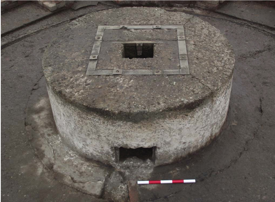
Figure 33. LAA gun pedestal with cabling aperture, looking north-east (0.5m scale)
