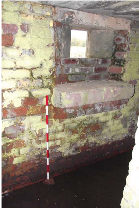
Figure 23. Pillbox, interior, embrasure in south-east wall, looking south-east (1m scale)
