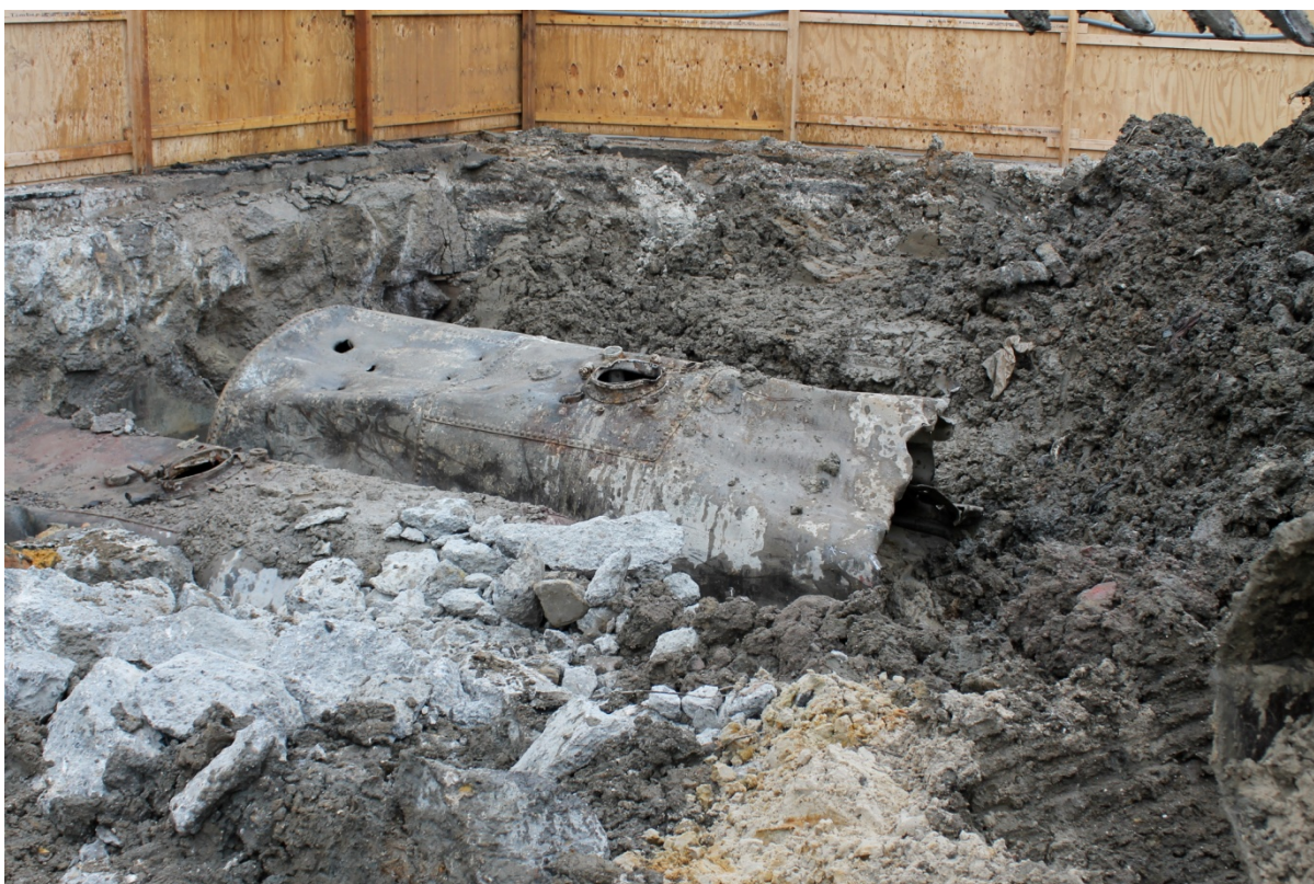
Plate 1: Westernmost tanks in situ
