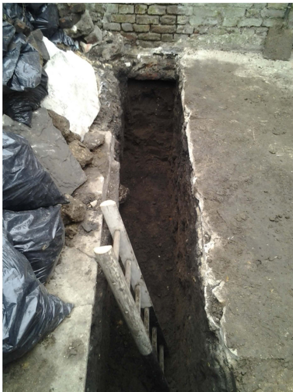
Plate 1: Trench 1 Looking North-West
