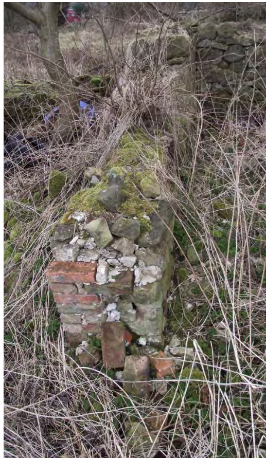
Plate 16. Detail of partition wall in derelict buildings, looking north
