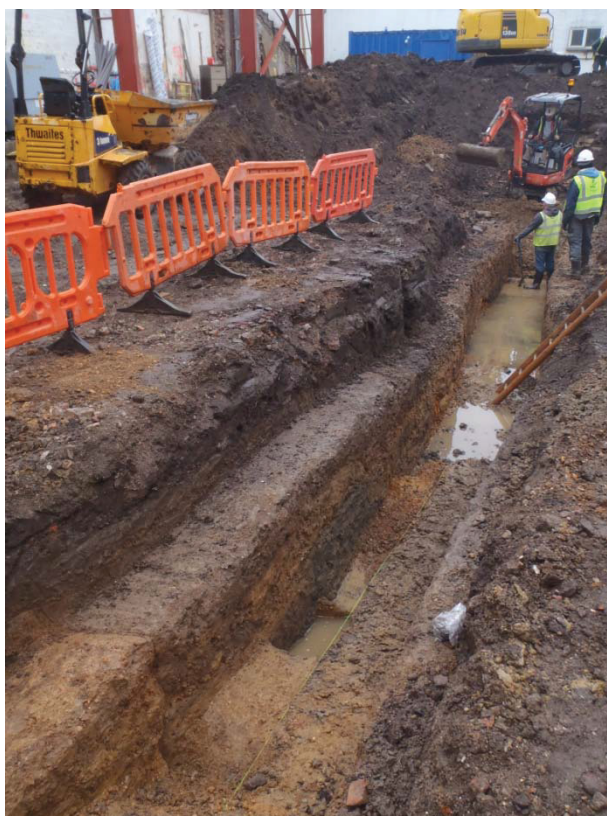
Photograph of Trench 1. Note the upstanding ridge of natural brickearth, [80], in the southern edge of the trench and the intercutting quarry pits to the immediate north. Photograph faces northwest.
