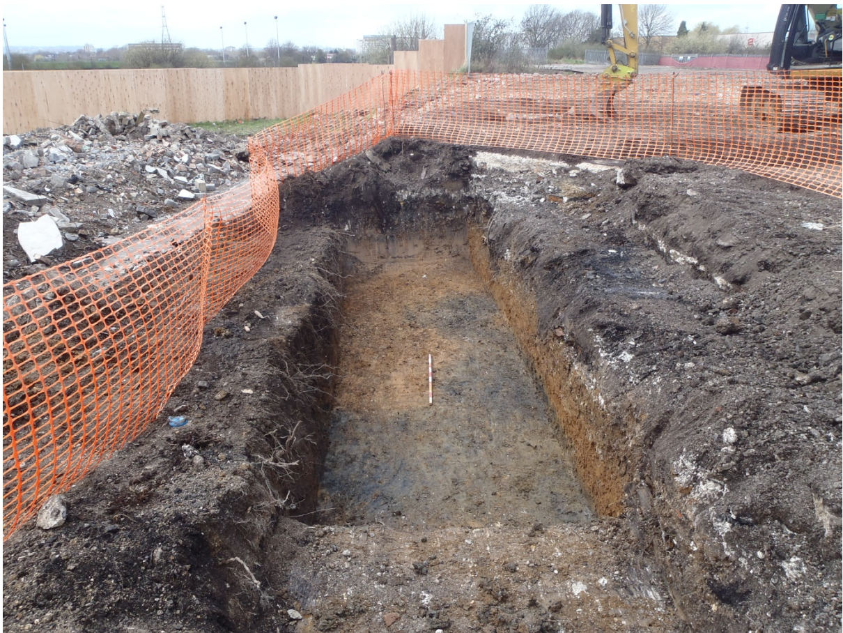
Plate 2: Trench 2 looking west.
