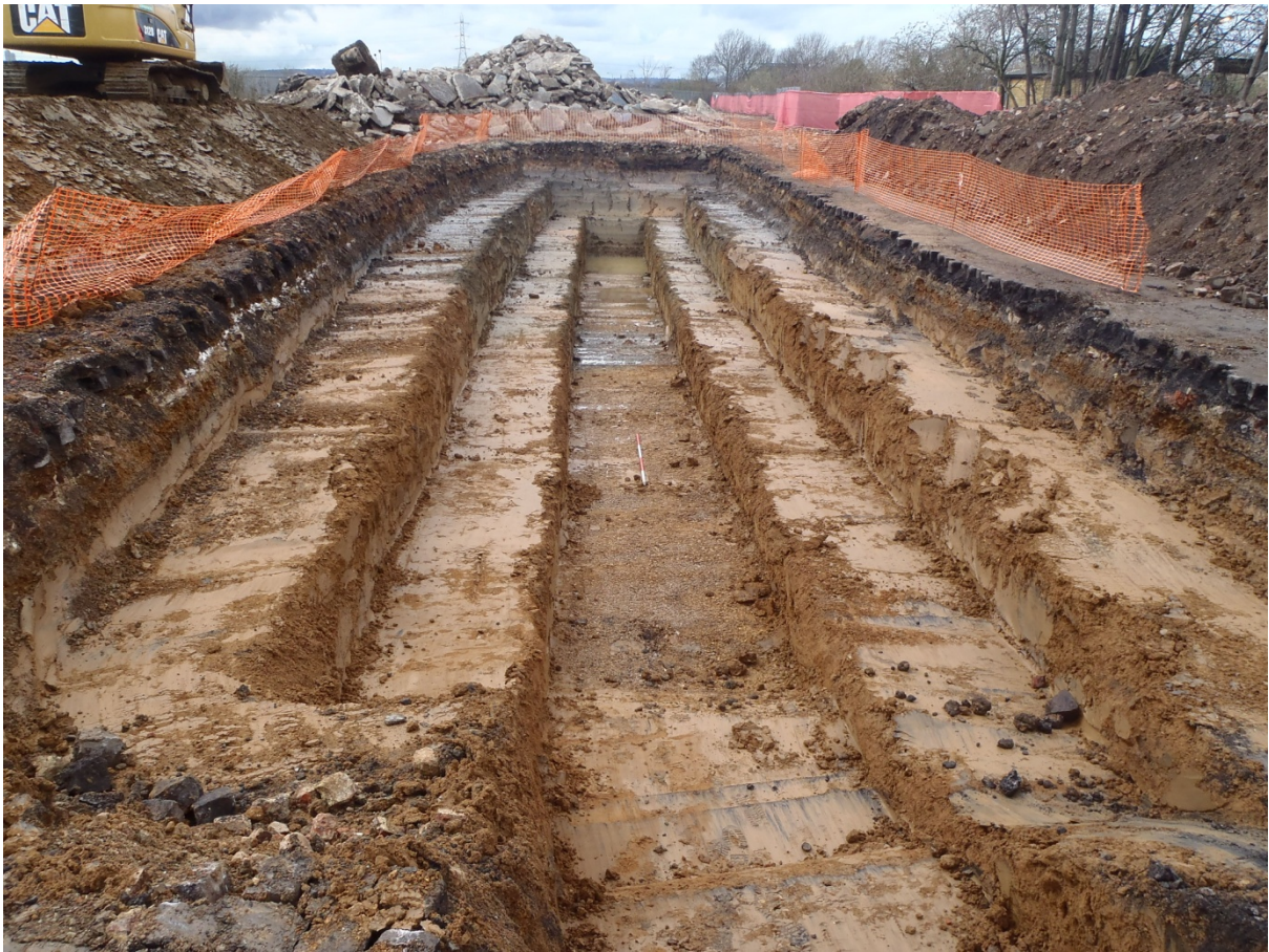
Plate 3: Trench 3, looking west
