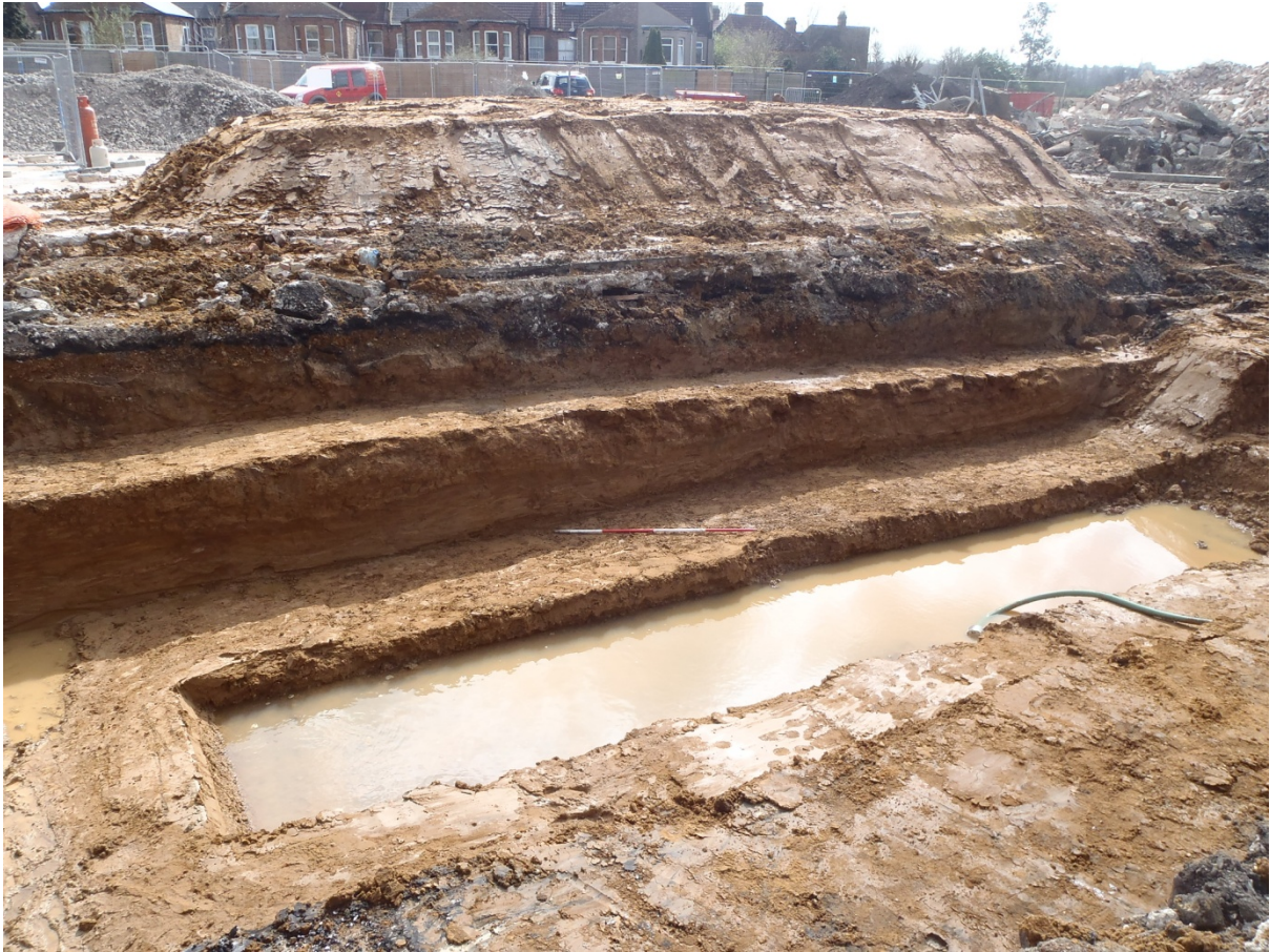
Plate 4: Trench 4 looking southwest showing Sections 3 and 4
