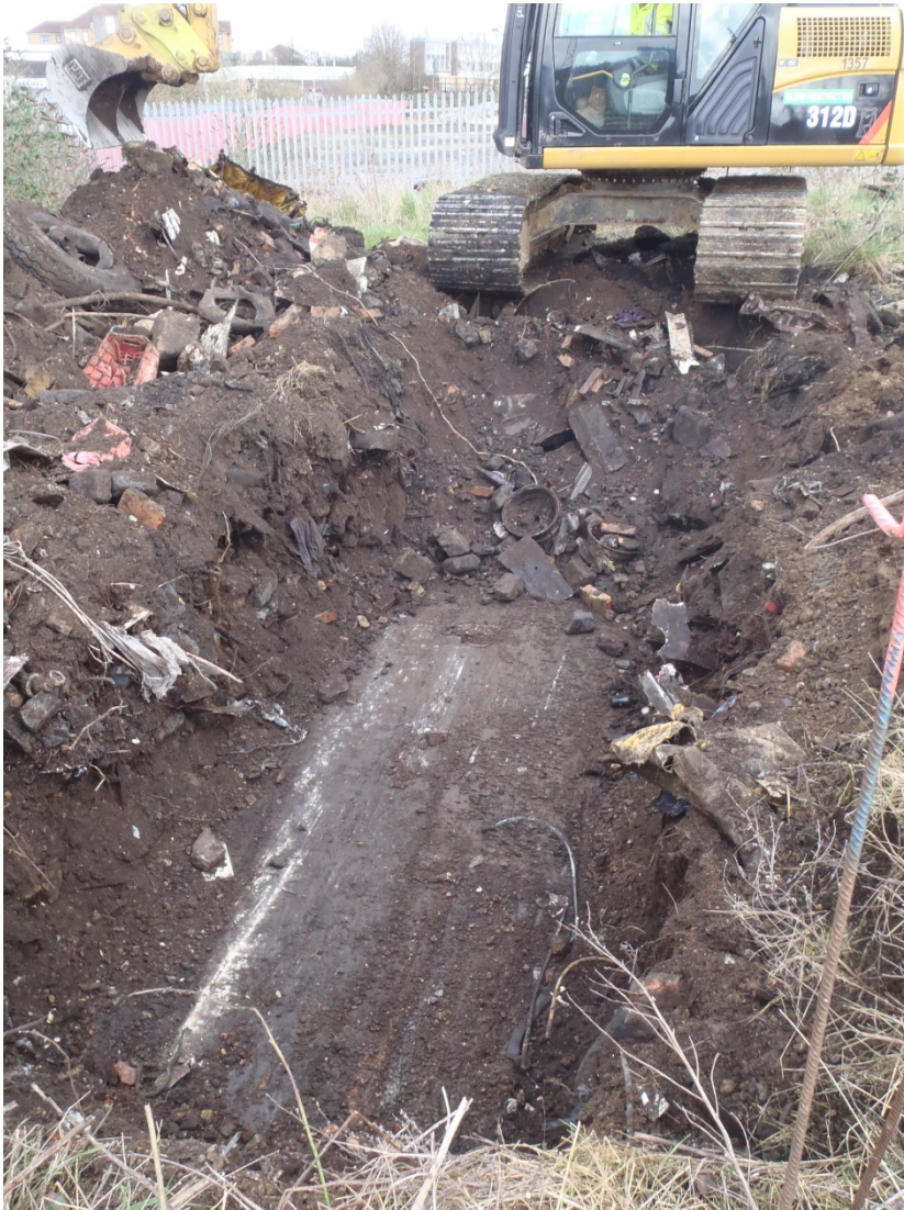
Plate 1: Trench 1 looking east illustrating modern landfill overlying concrete.
