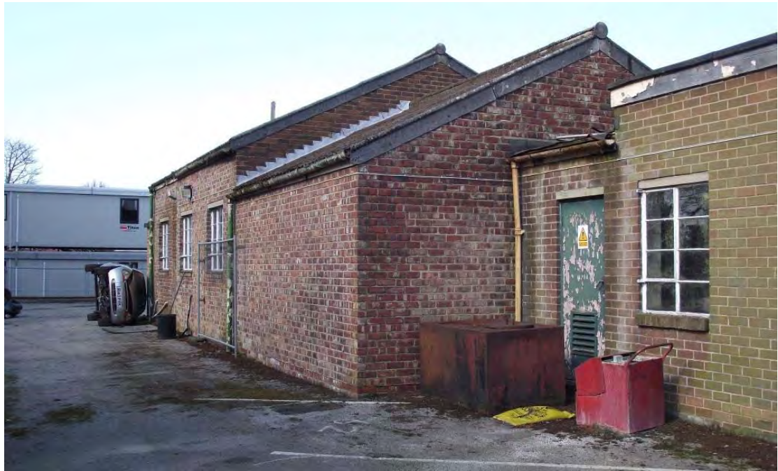
Plate 23. Former Ambulance Station, Workshop/Storage, west elevation (oblique), looking NNE
