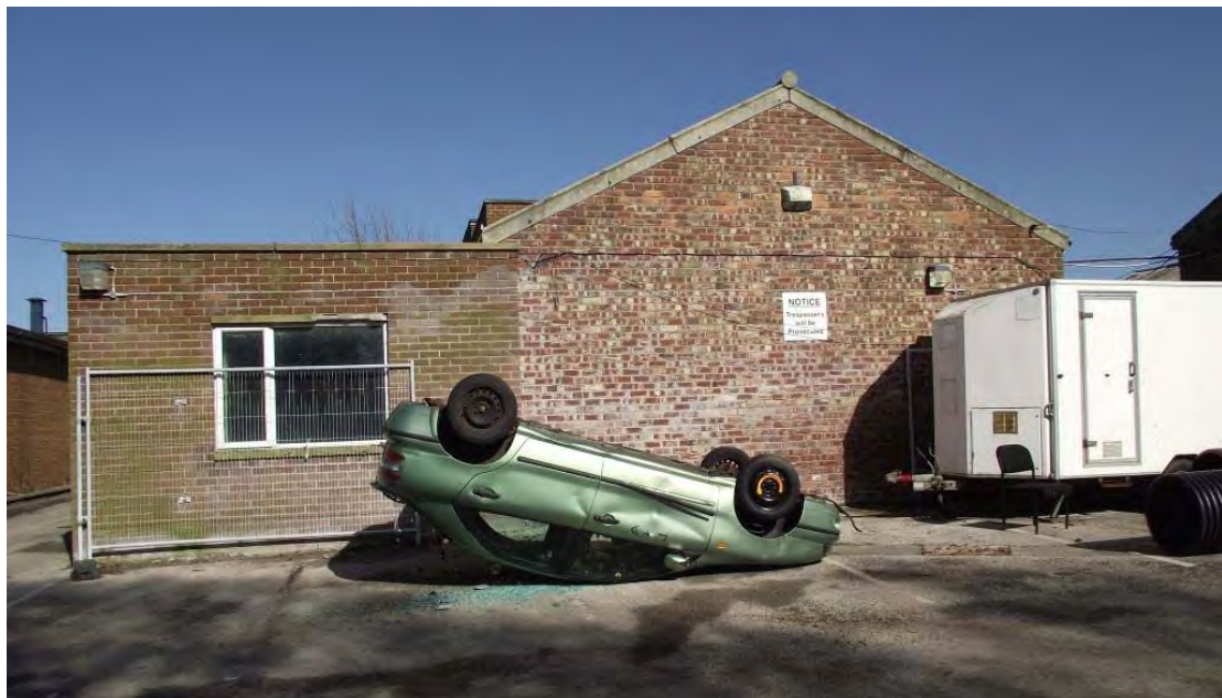
Plate 22. Former Ambulance Station, Garage, west elevation, looking east
