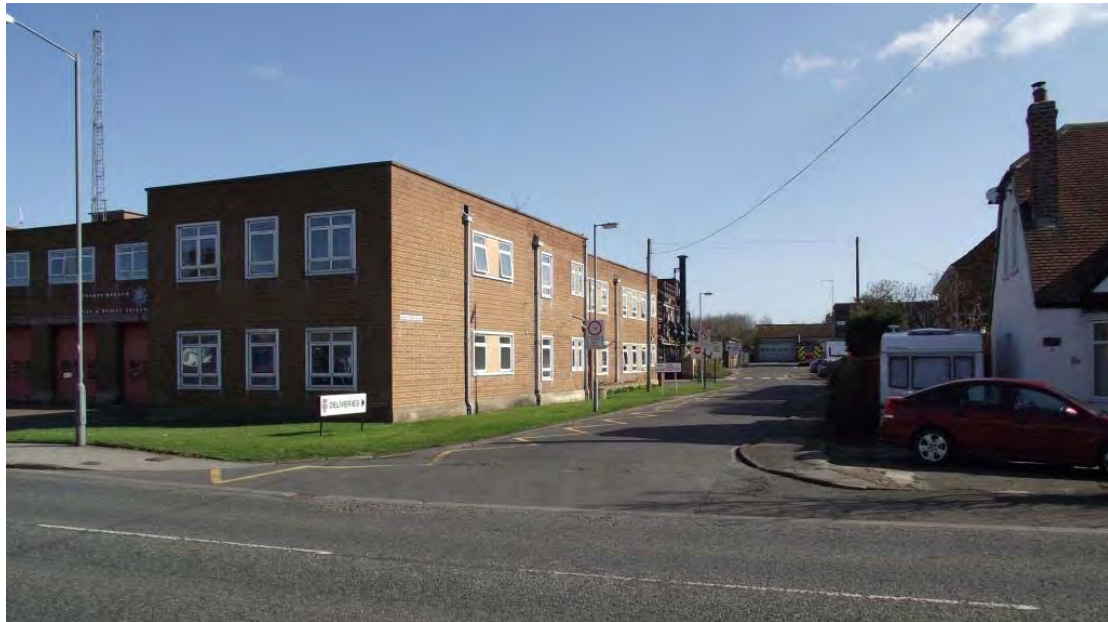
Plate 5. Entrance to study site along High Carr Close, looking south
