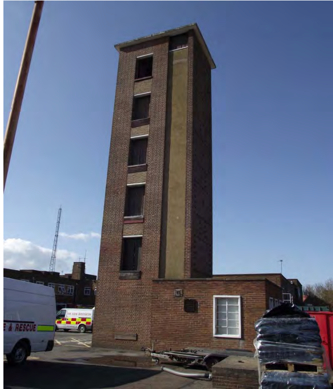
Plate 25. Drill Tower, south elevation, looking NNW
