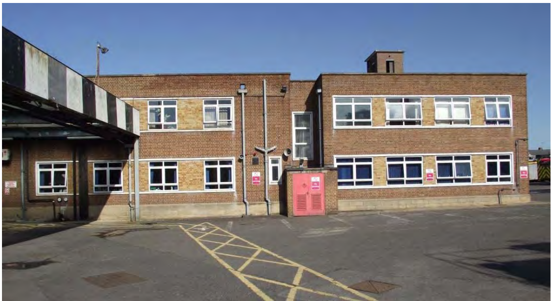
Plate 10. Headquarters Building, Admin Block, west elevation, looking east
