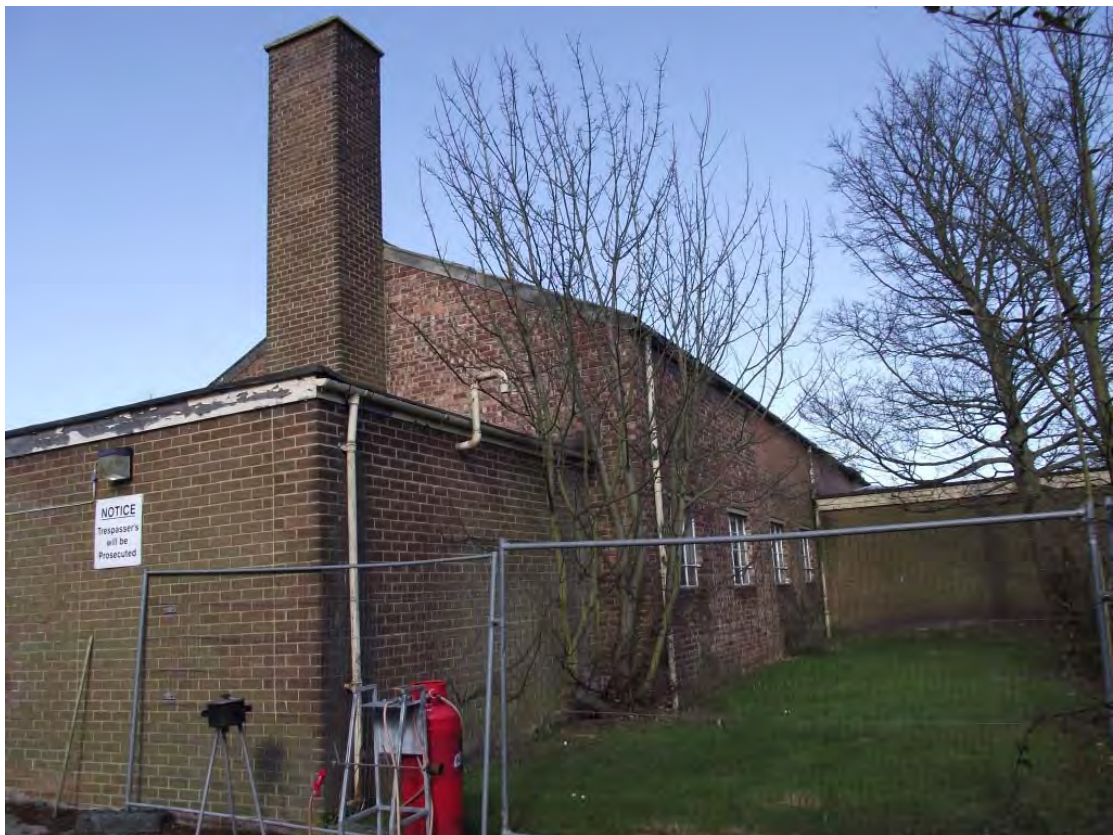
Plate 24. Former Ambulance Station, Garages, south elevation (oblique), looking ENE
