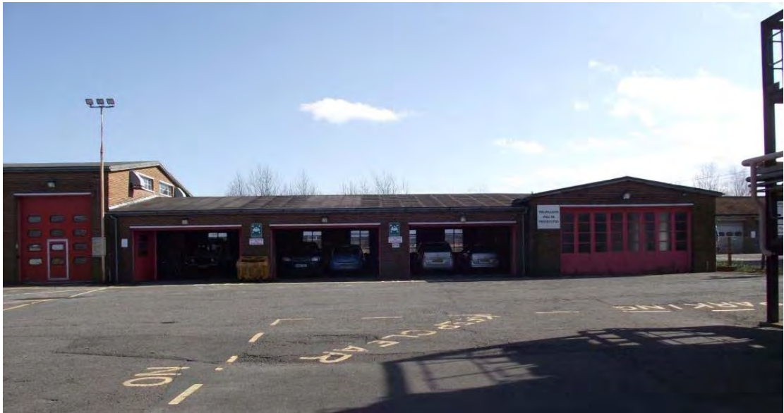
Plate 13. Workshop/Garage Block, western part, north elevation, looking SSE
