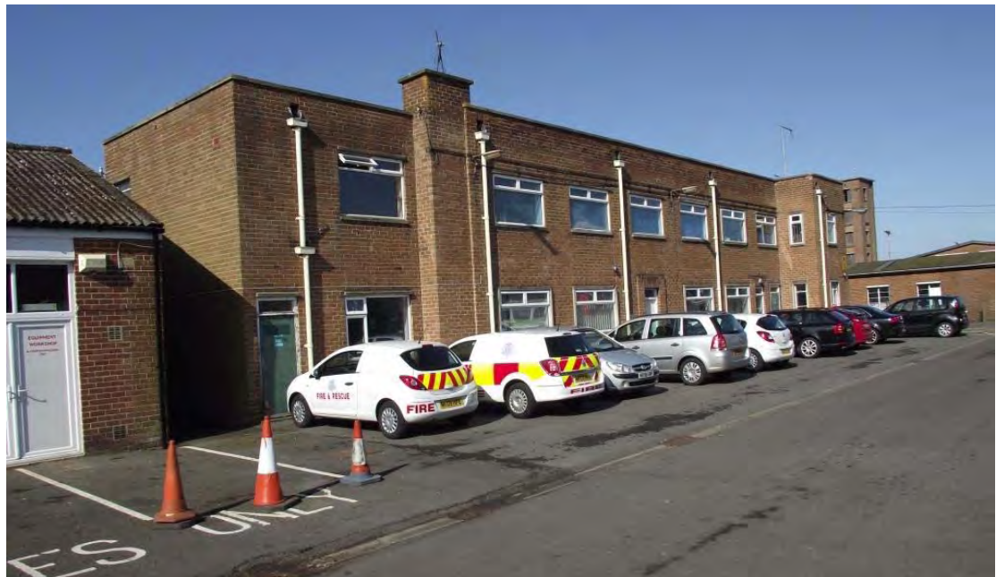
Plate 16. Driver Training Unit, south elevation (oblique), looking north-east
