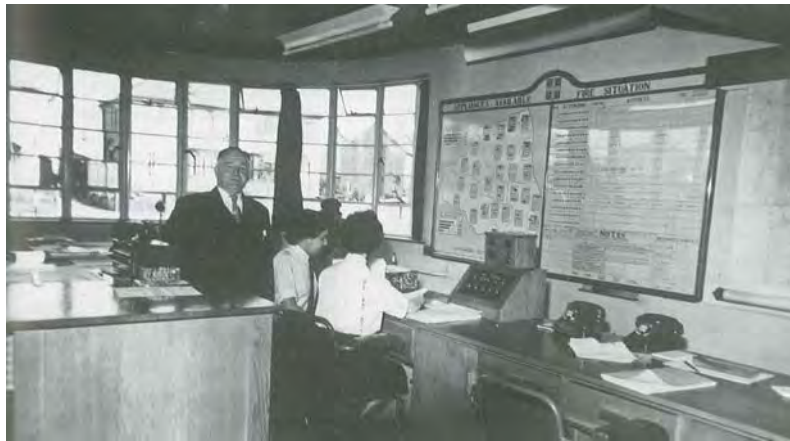
Figure 13. Interior of Control Room, c. 1956, looking north
