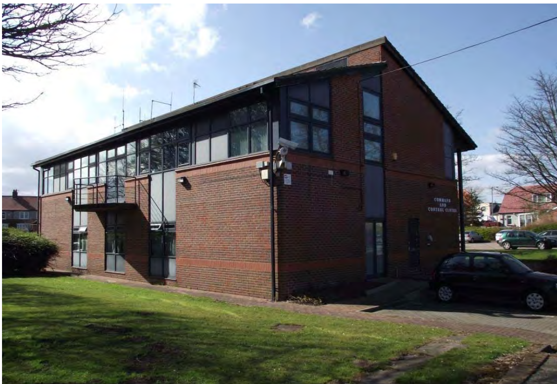
Plate 20. Command and Control Centre, looking north-west
