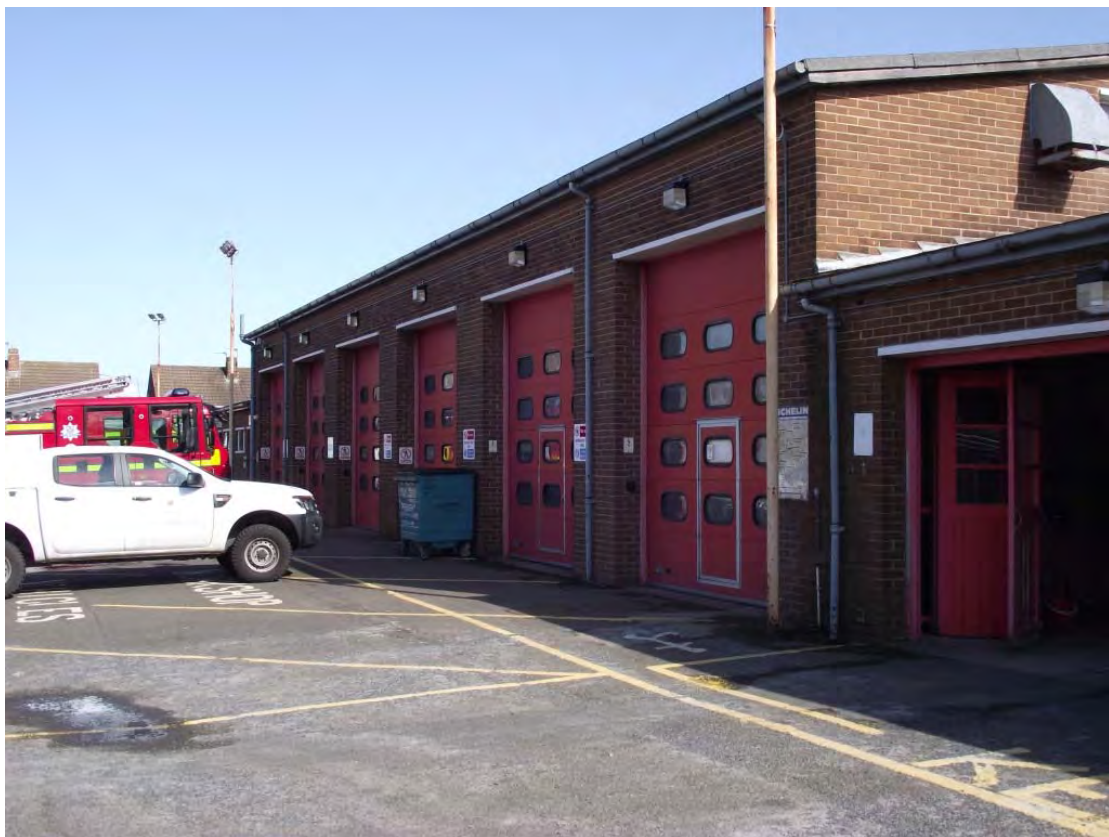
Plate 12. Workshop/Garage Block, central part, north elevation (oblique), looking ESE
