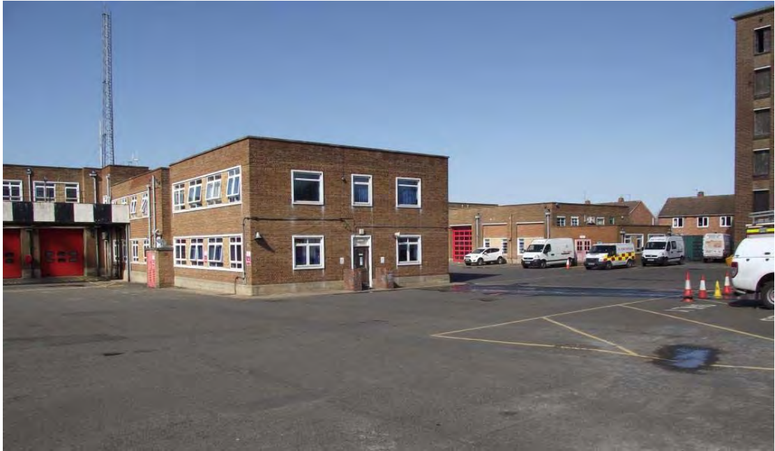
Plate 9. Headquarters Building, Admin Block, looking north-east
