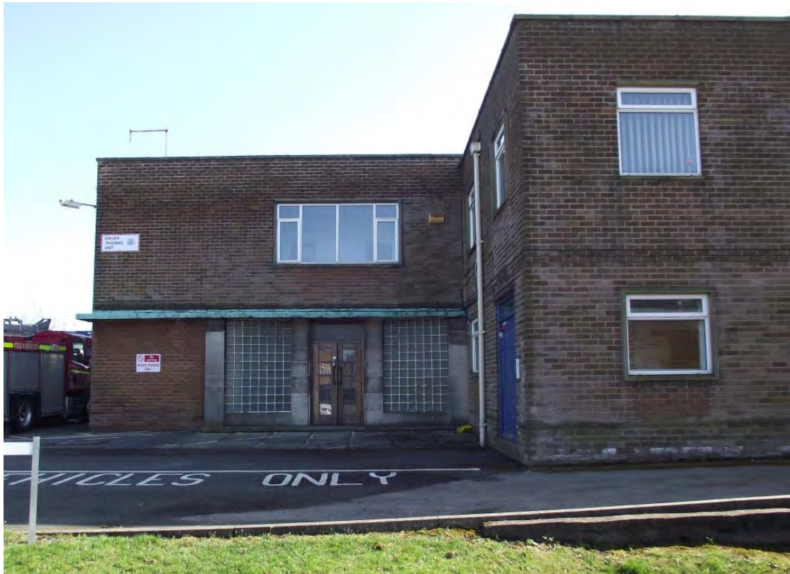
Plate 17. Driver Training Unit, north elevation (eastern part), looking SSE
