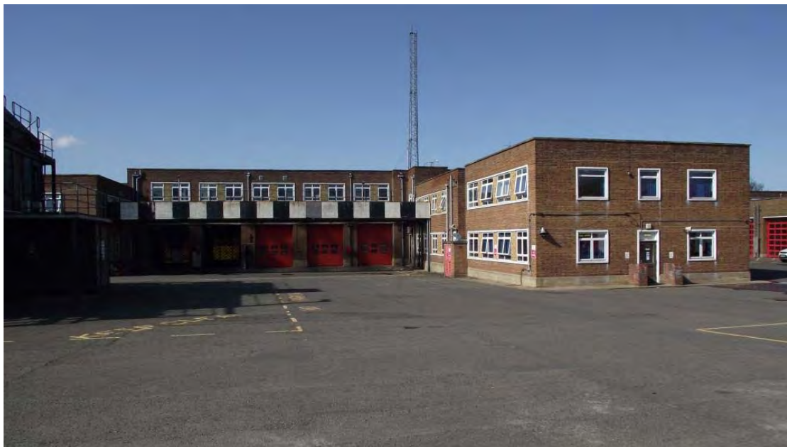
Plate 8. Headquarters Building, Appliance Garages and Admin Block, south elevation, looking north
