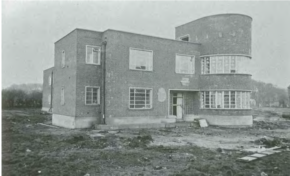
Figure 12. Administration Block/Control Room under construction, c. 1956, looking south-west
