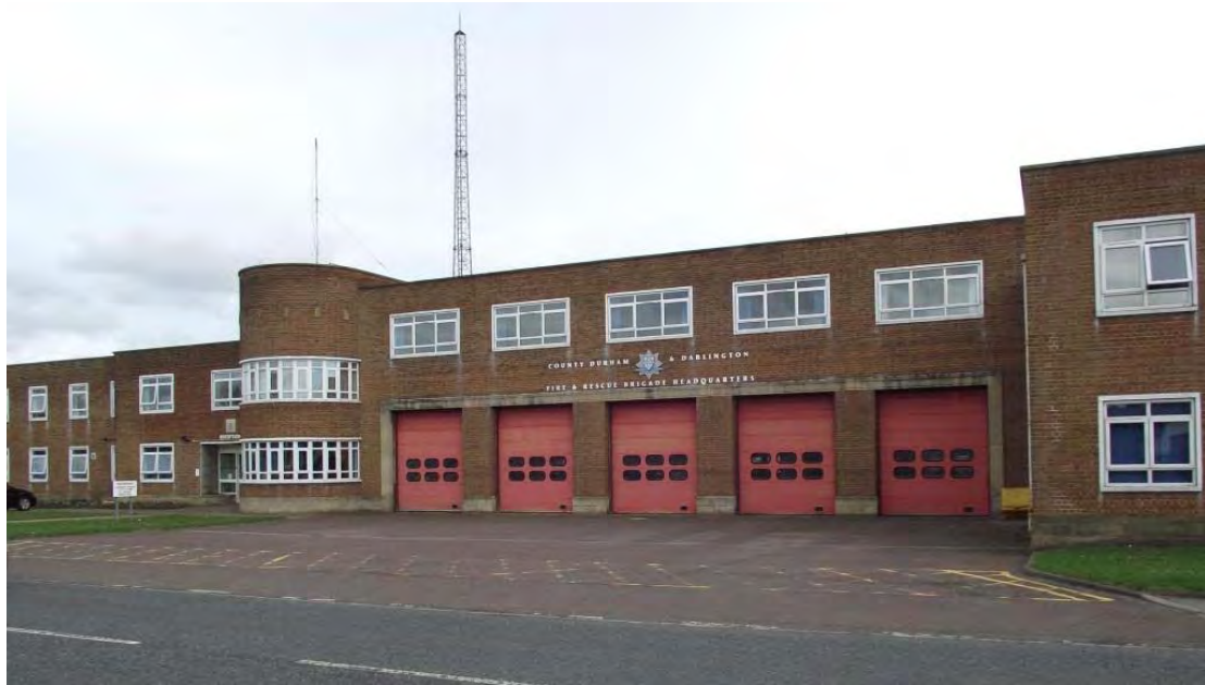
Plate 3. Headquarters Building, Appliance Garages, north elevation, looking SSE
