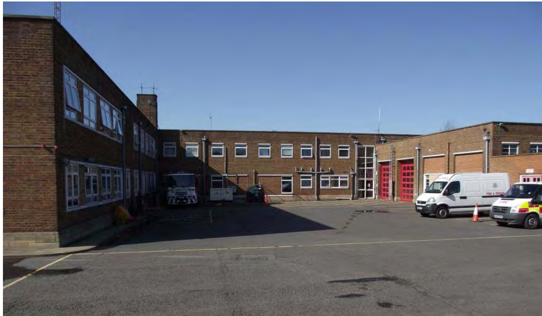
Plate 11. Headquarters Building, Training School, south elevation, looking north
