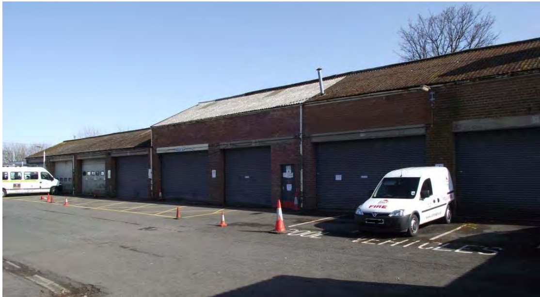
Plate 15. Former Ambulance Station, Garage block, north elevation (oblique), looking ESE
