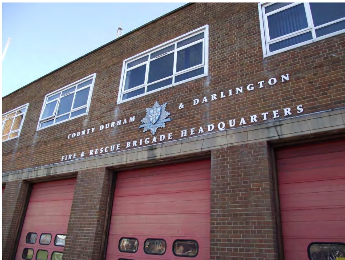
Plate 4. Headquarters Building, north elevation detail, looking SSE
