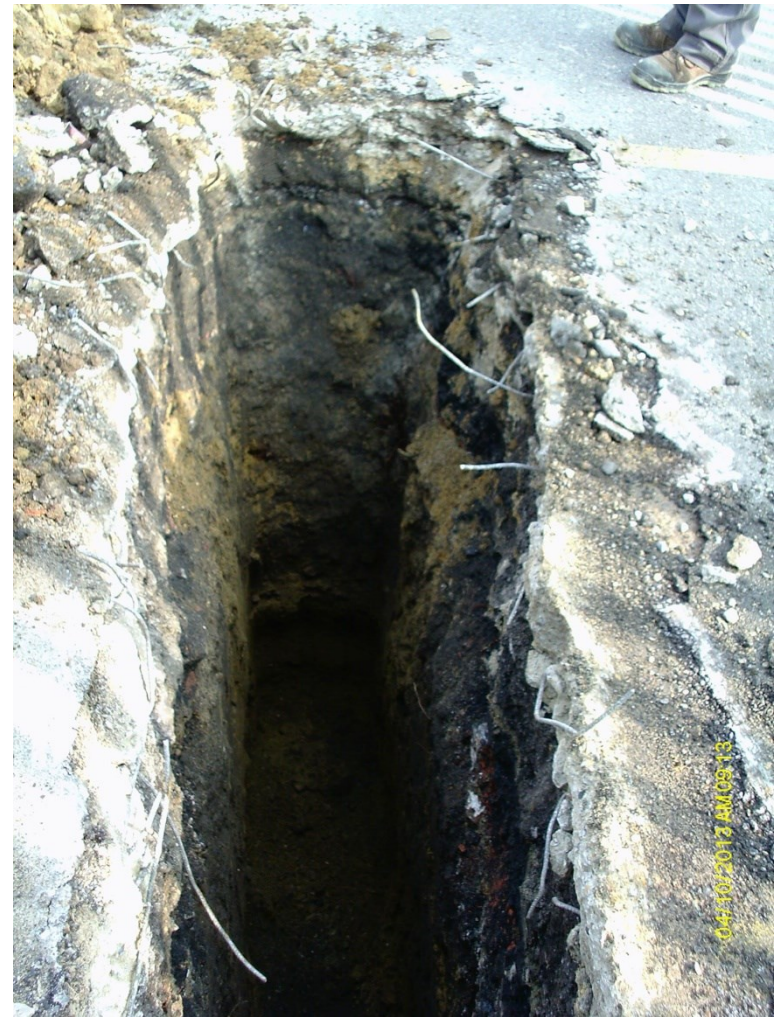
Plate 5: Test pit 3, facing north
