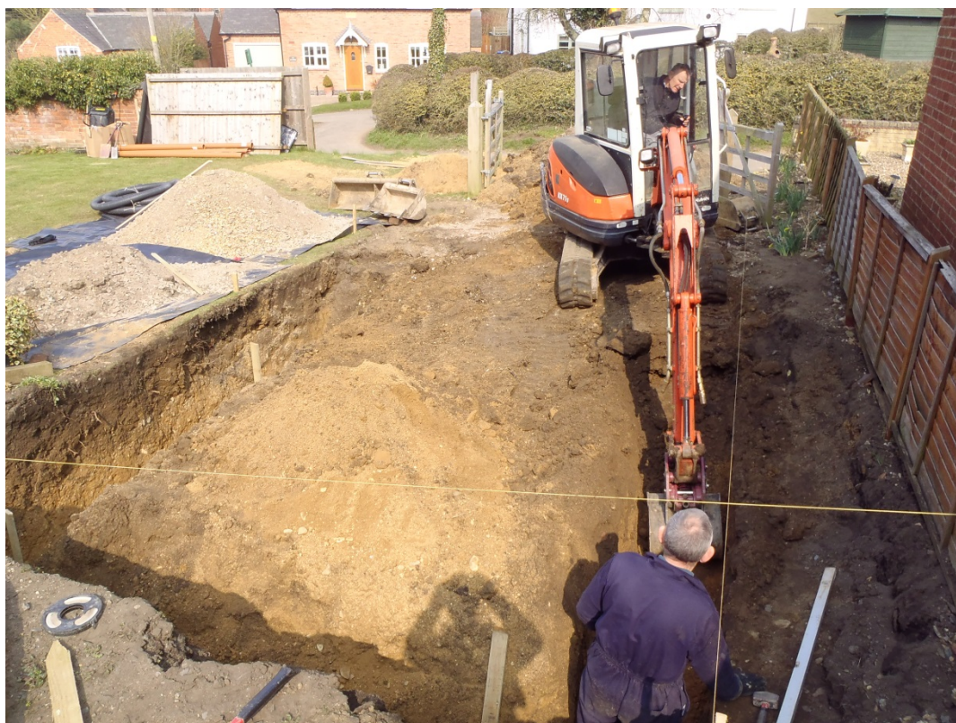
Plate 3, Excavation of footings, looking north-west
