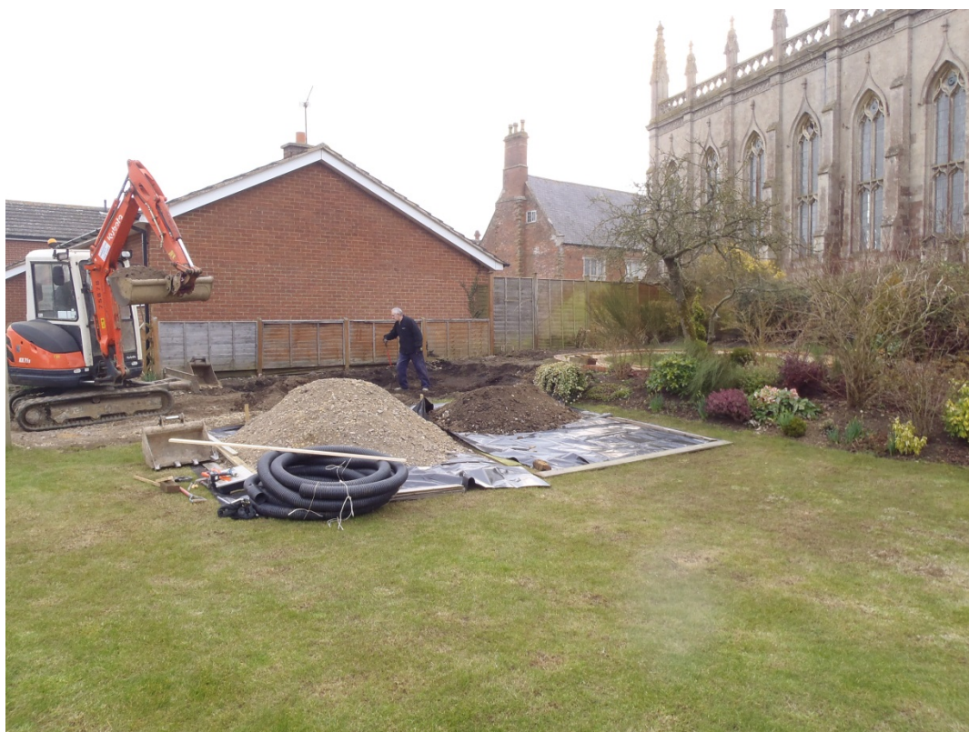
Plate 4, General site view, looking south-east
