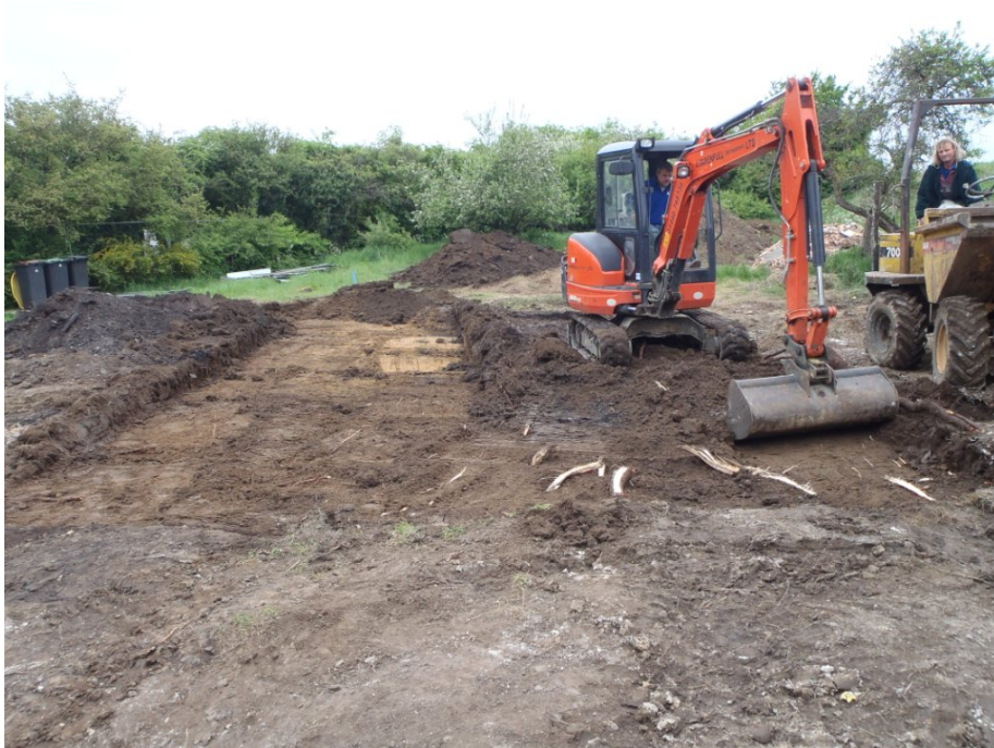
Plate 3: Stripping the footprint of the new building.
