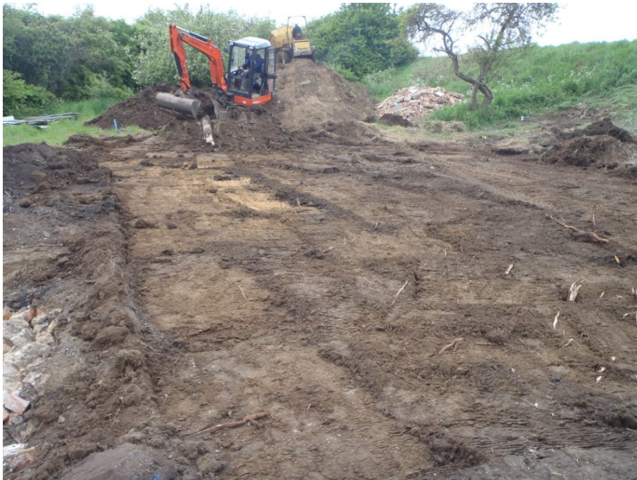
Plate 4: Close-up of area, stripped.
