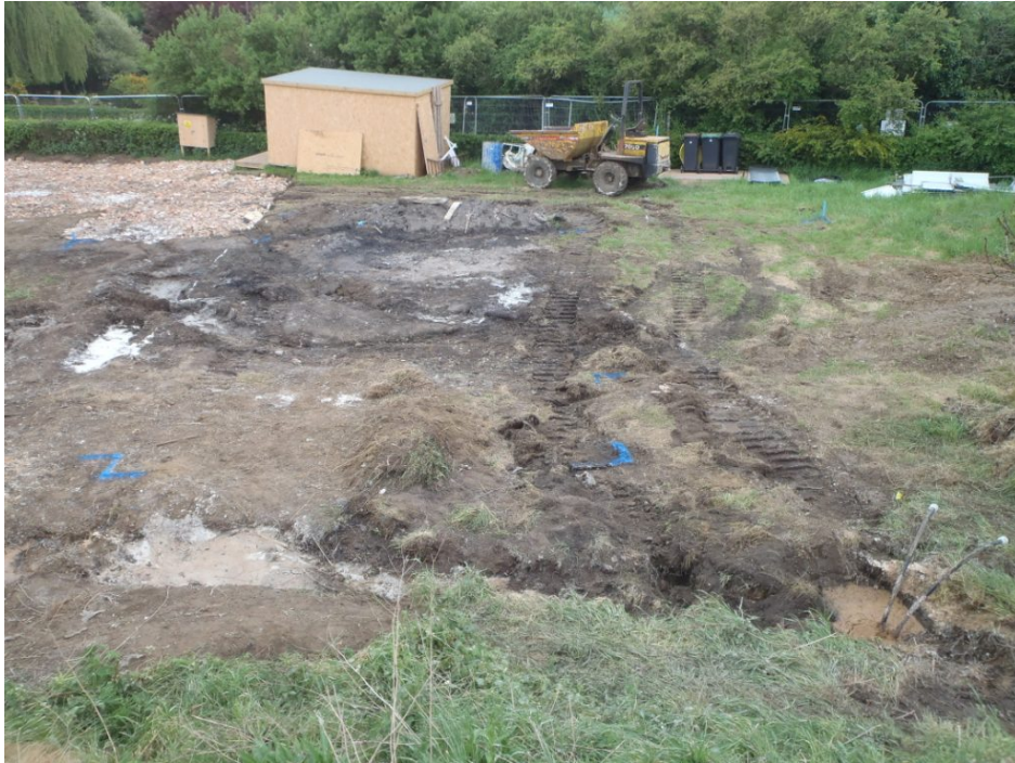
Plate 1: Area of site before commencement of groundworks.
