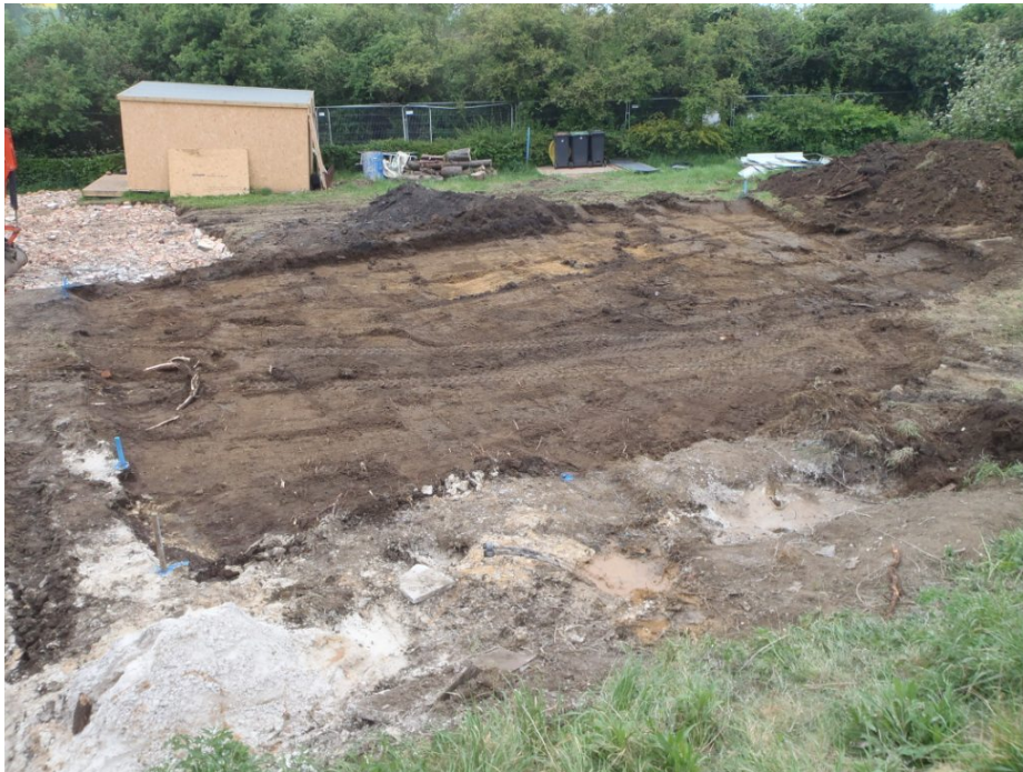
Plate 2: New building footprint, stripped of topsoil.
