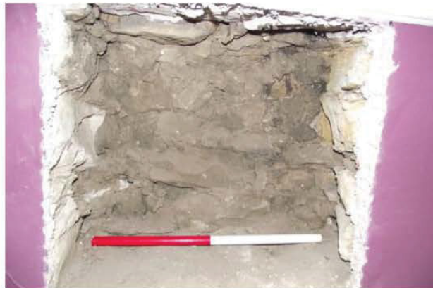
Plate 68: First floor, Bedroom 3, enabling hole in north wall (0.5m scale)
