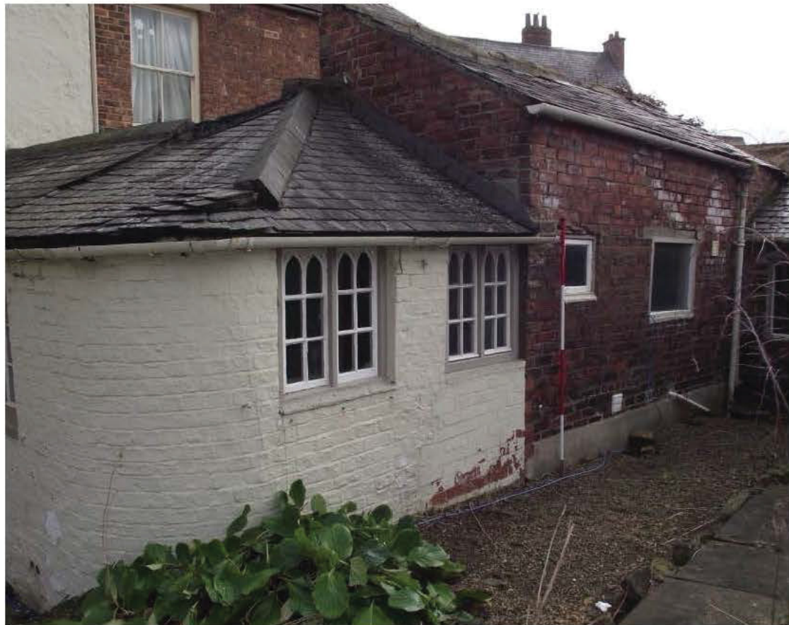
Plate 6: S-shaped extension, west-facing elevation, oblique view, prior to works (2m scale)
