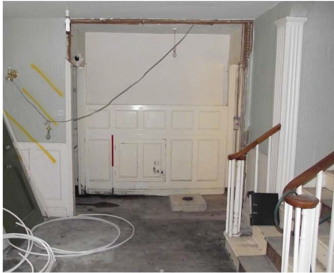
Plate 33: Front element, ground floor, main lobby (1m scale)
