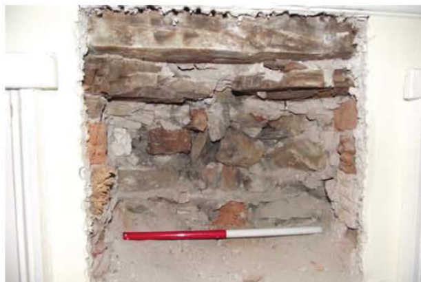
Plate 69: First floor, Bedroom 3, central enabling hole in east wall (0.5m scale)
