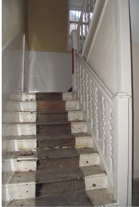
Plate 54: Northern rear element, staircase, rising from ground floor (1m scale)
