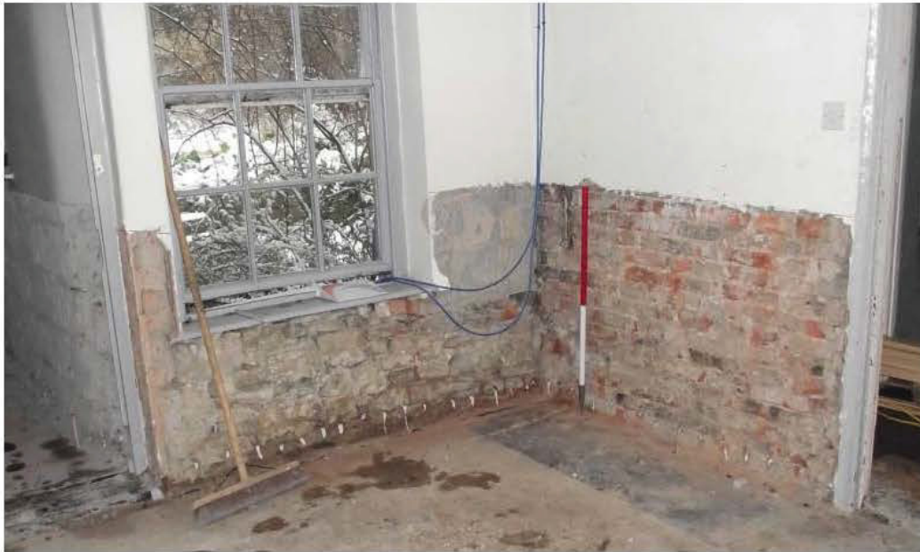
Plate 40: Southern rear element, ground floor, Reception Room 2, exposed masonry in north-west corner (1m scale)
