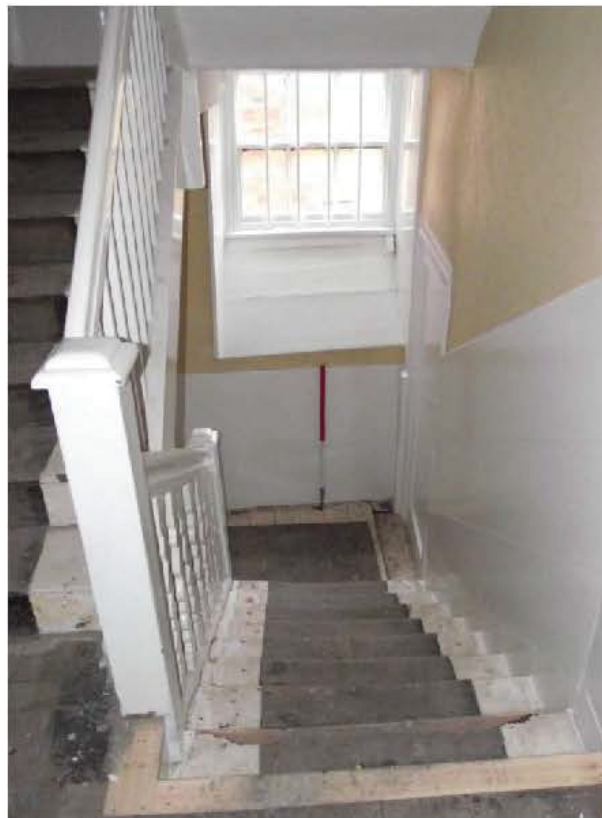
Plate 58: Northern rear element, staircase, from first floor landing (1m scale)
