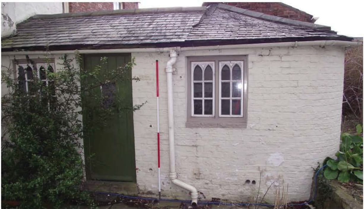
Plate 7: S-shaped extension, north-facing elevation (kitchen range), prior to works (2m scale)
