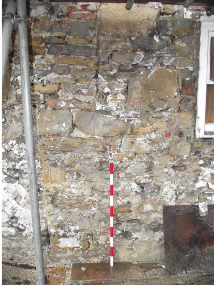
Plate 11: North-facing (side) elevation, sandstone masonry interface (1m scale)
