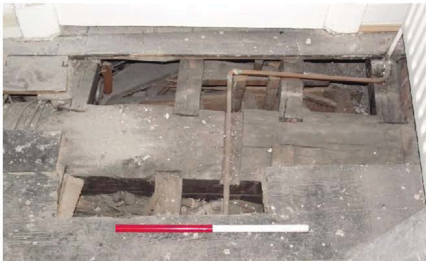
Plate 72: First floor, Bedroom 3, removed floorboards showing timber beam (0.5m scale)
