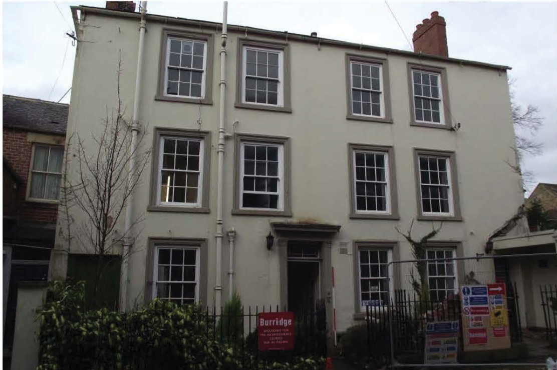
Plate 3: Front element, east-facing (front) elevation, prior to works (2m scale)
