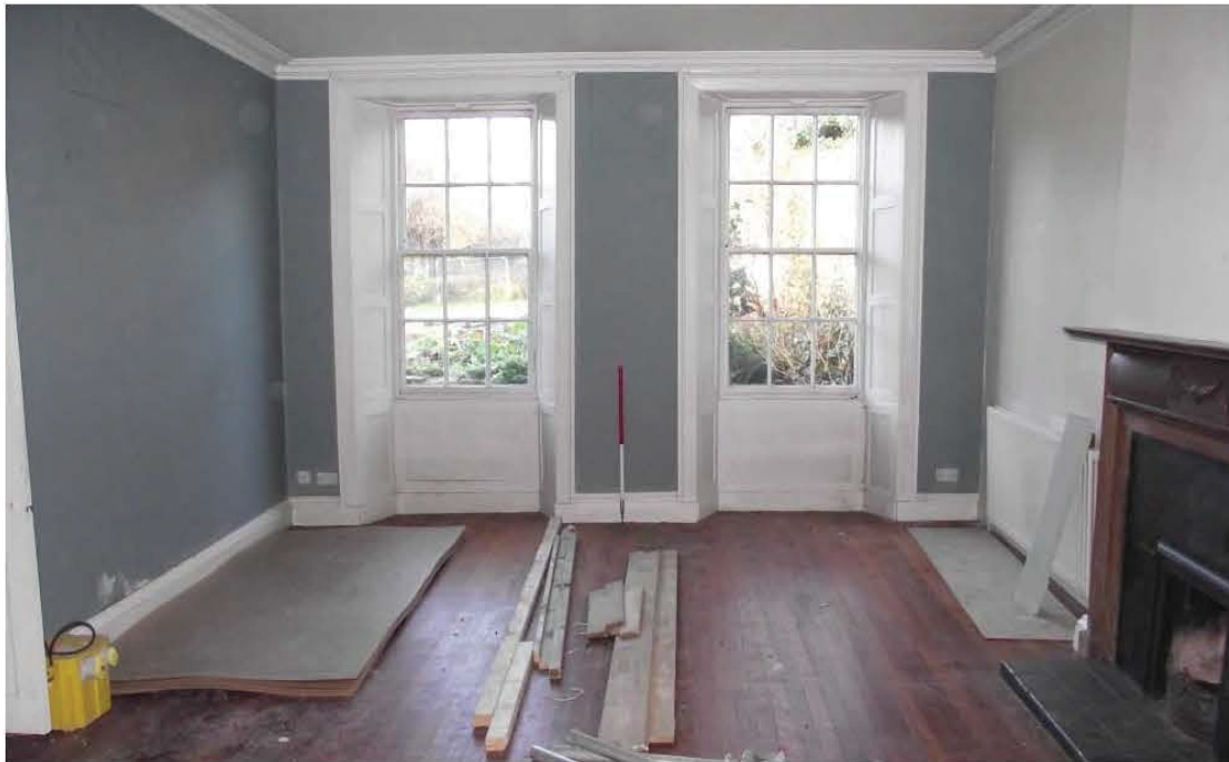
Plate 43: Northern rear element, ground floor, Reception Room 1 (1m scale)
