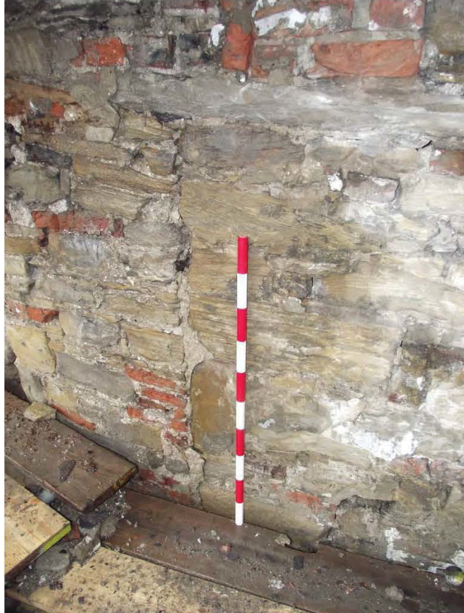
Plate 15: North-facing (side) elevation, masonry interface (1m scale)
