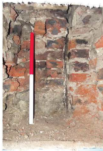
Plate 48: Reception Room 1, westernmost enabling hole in south wall, detail (0.5m scale)
