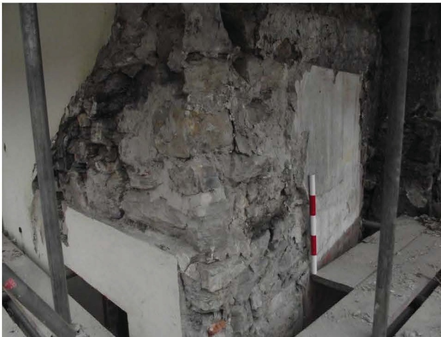
Plate 12: North-eastern corner of building, sandstone masonry above doorway (0.5m scale)
