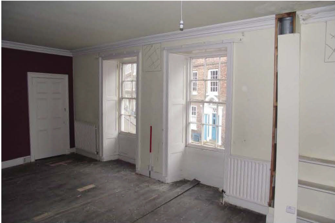
Plate 65: Front element, first floor, Bedroom 3, eastern part (1m scale)
