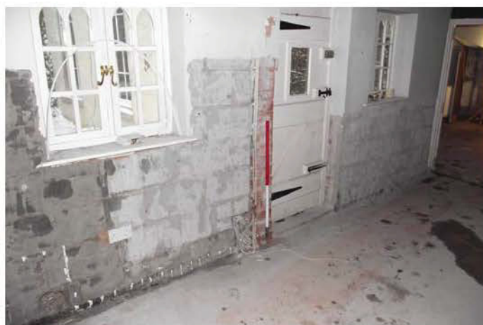
Plate 53: S-shaped rear extension, kitchen range, north wall (1m scale)
