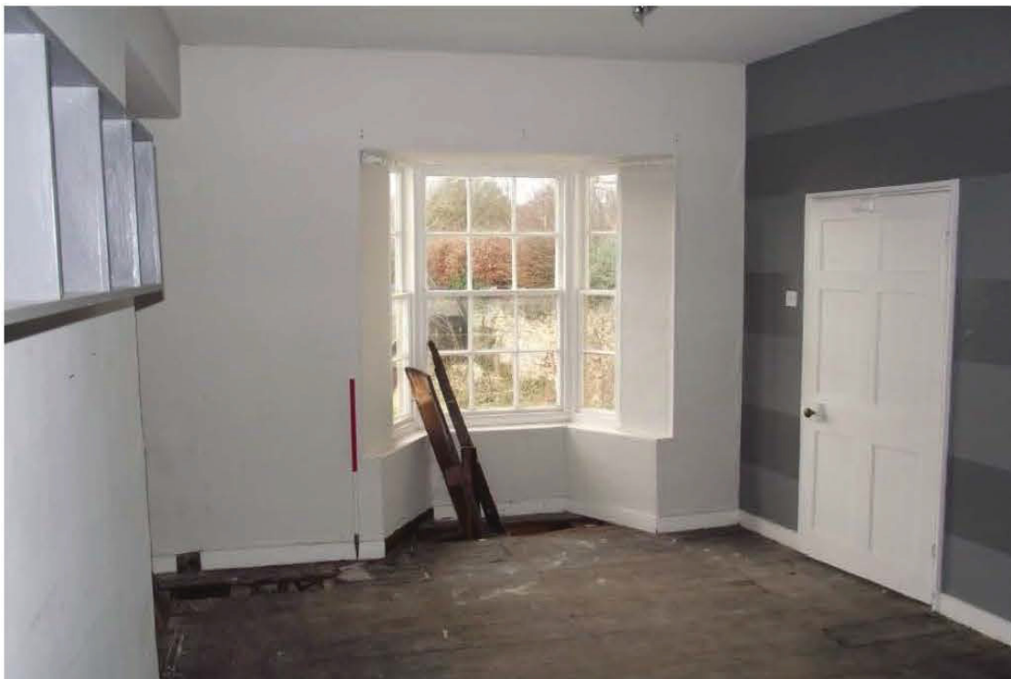
Plate 64: Southern rear element, first floor, Bedroom 2, western part (1m scale)
