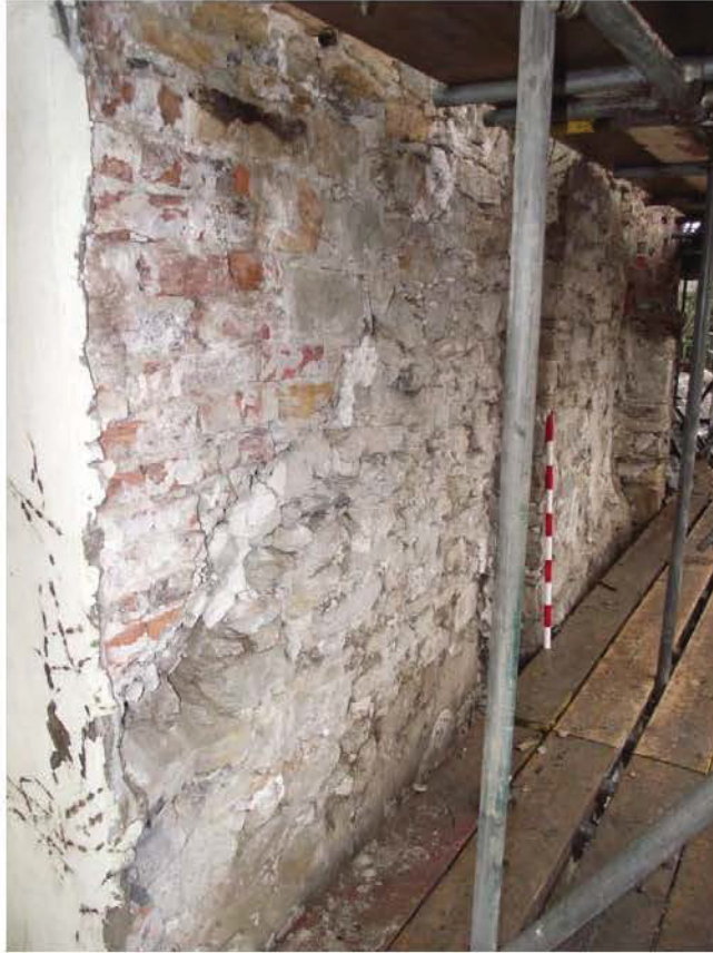
Plate 13: North-facing (side) elevation, brick/sandstone masonry interface (1m scale)
