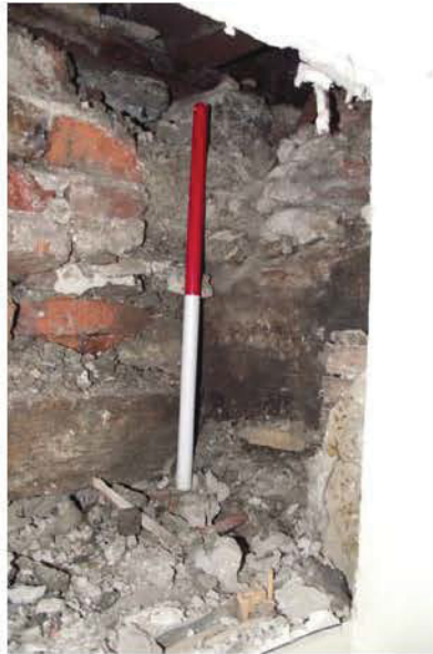
Plate 70: First floor, Bedroom 3, southern enabling hole in east wall (0.5m scale)
