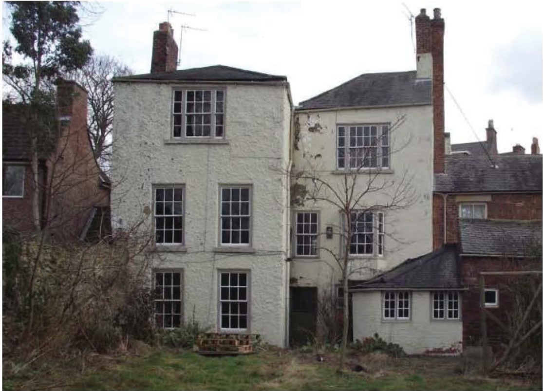
Plate 5: Rear elements, west-facing (rear) elevation, prior to works (view, no scale)
