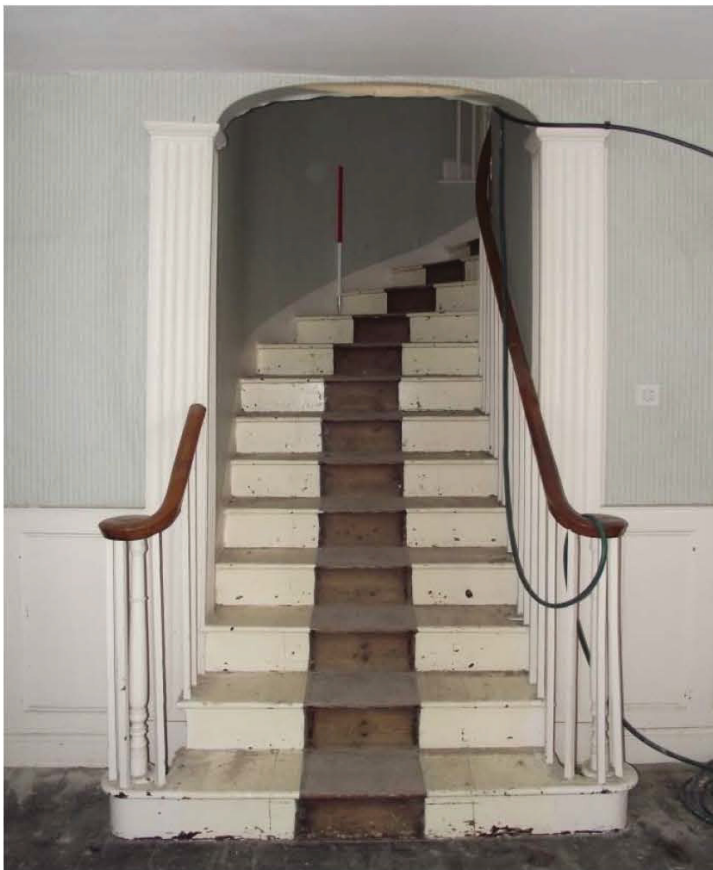
Plate 34: Front element, ground floor, staircase from main lobby (1m scale)
