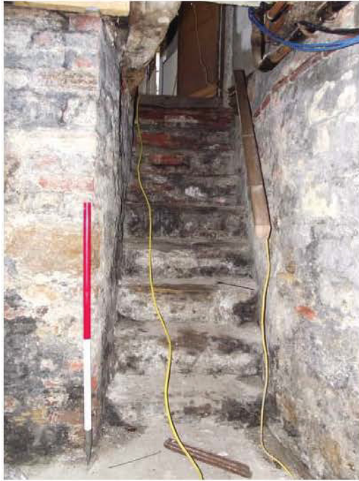
Plate 30: Cellar, access steps (1m scale)
