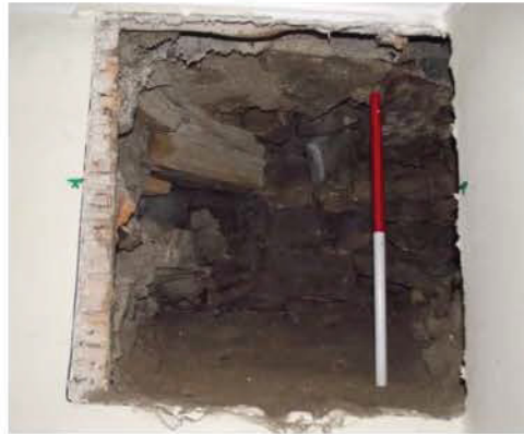
Plate 46: Reception Room 1, easternmost enabling hole in north wall, detail (0.5m scale)
