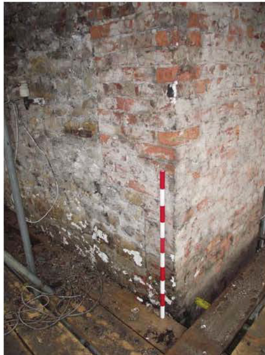
Plate 20: North-facing (side) elevation, northern element, brickwork façade on earlier masonry (1m scale)
