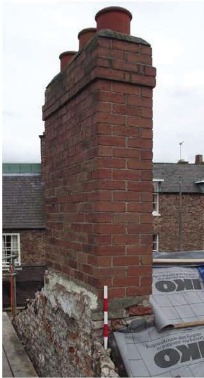
Plate 26: North-facing (side) elevation, front element, chimney stack on roofline (0.5m scale)
