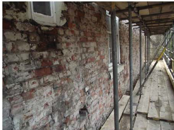
Plate 21: North-facing (side) elevation, northern element, upper brickwork (view, no scale)
