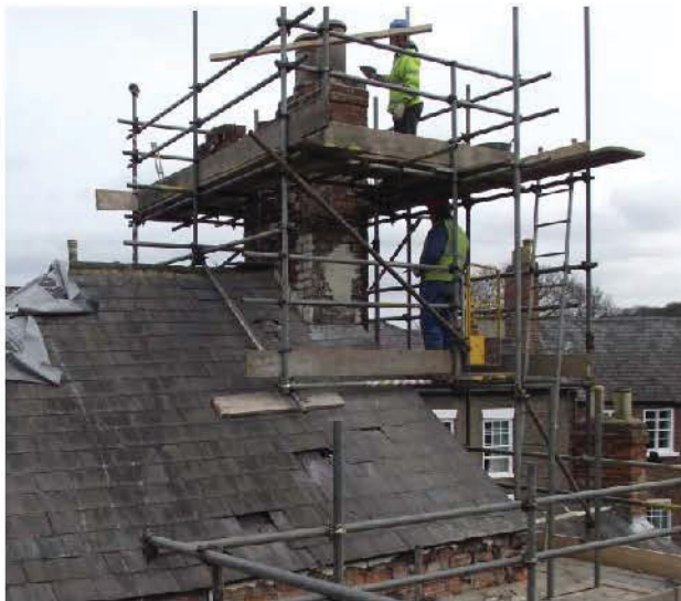
Plate 28: Southern rear element, chimney stack in south-facing elevation (view, no scale)
