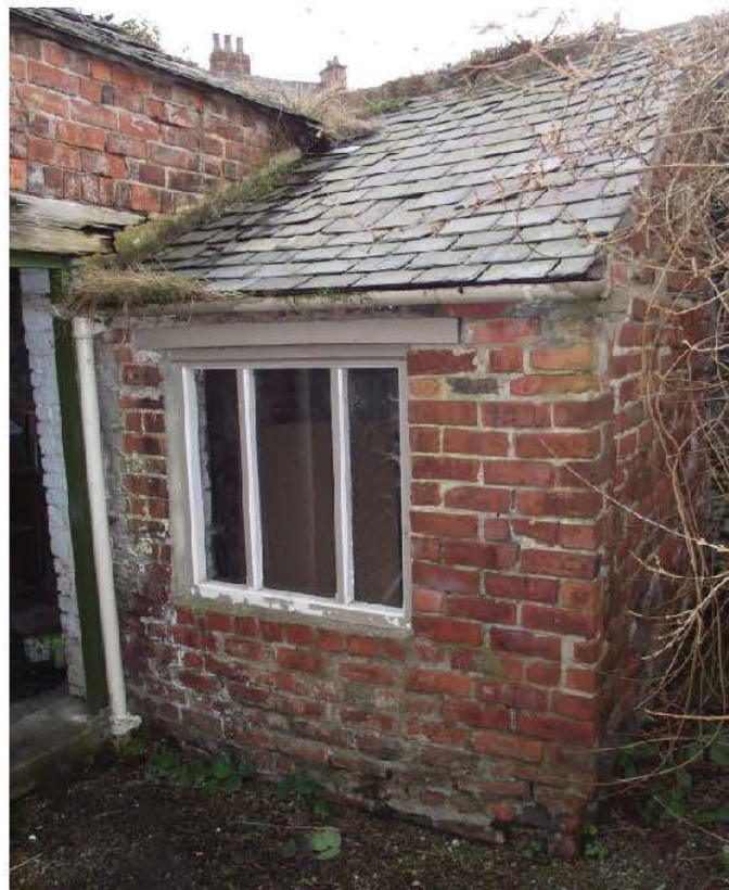
Plate 8: S-shaped extension, north-facing elevation (outbuilding), prior to works (view, no scale)
