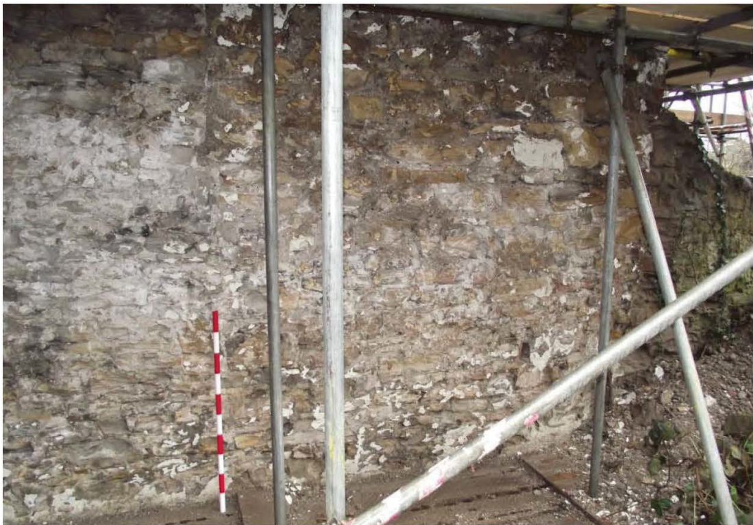
Plate 16: North-facing (side) elevation, sandstone masonry at western extent of rear element (1m scale)
