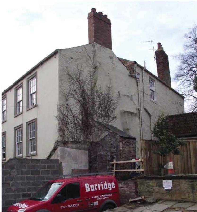
Plate 4: North-facing (side) elevation, oblique view, prior to works (view, no scale)
