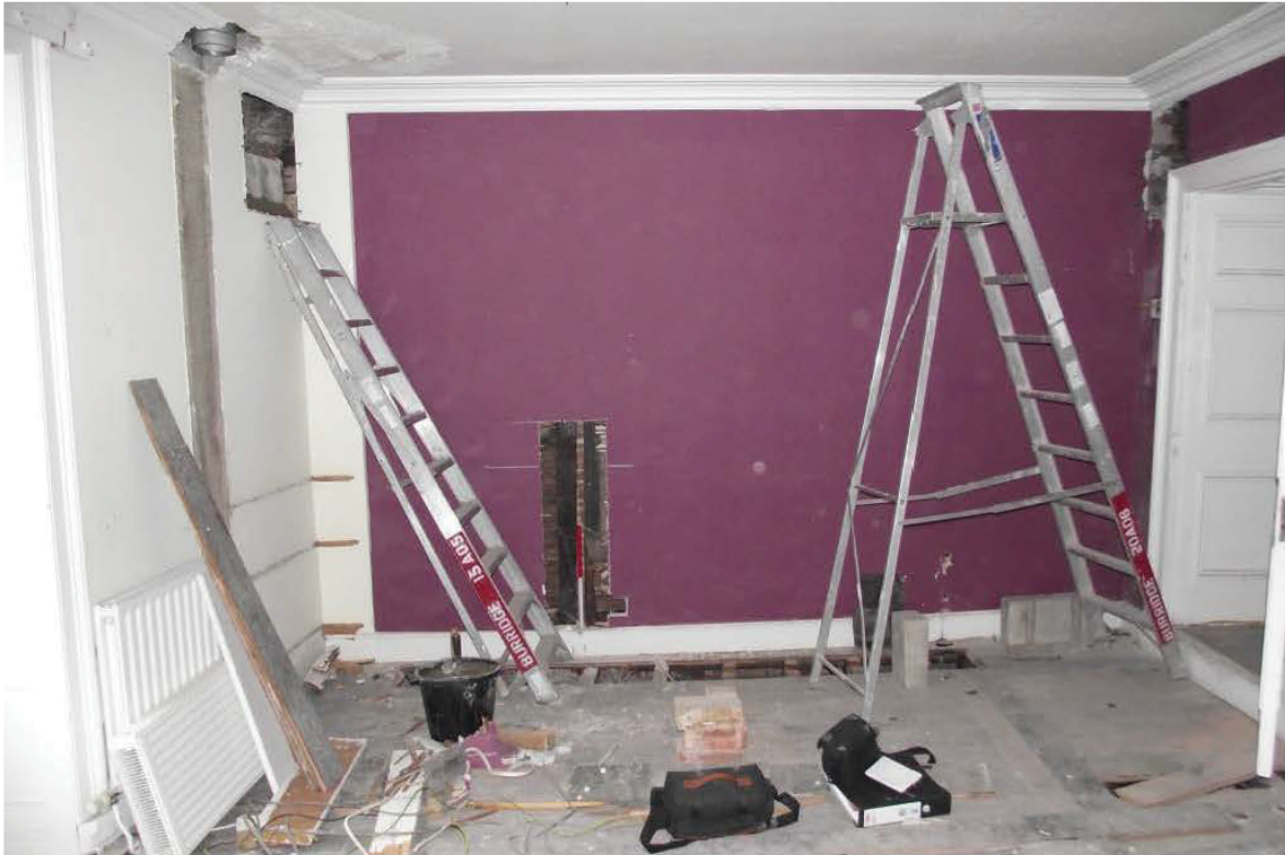
Plate 67: Front element, first floor, Bedroom 3, south end, during works (1m scale)
