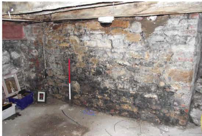
Plate 31: Cellar, west wall (1m scale)
