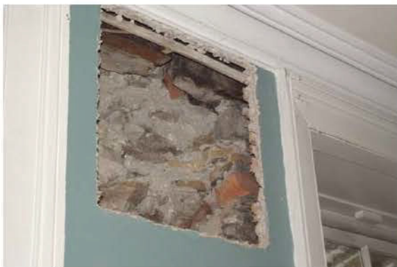
Plate 47: Reception Room 1, enabling hole in west wall, detail (view, no scale)
