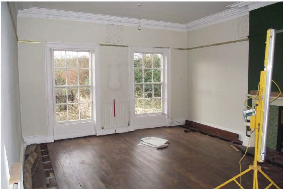
Plate 60: Northern rear element, first floor, Bedroom 1 (1m scale)
