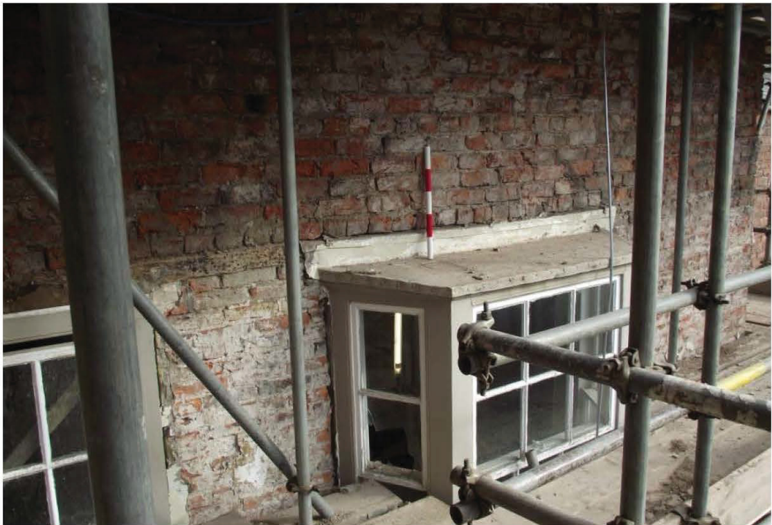
Plate 25: West-facing (rear) elevation, southern element, brickwork detail above window (0.5m scale)
