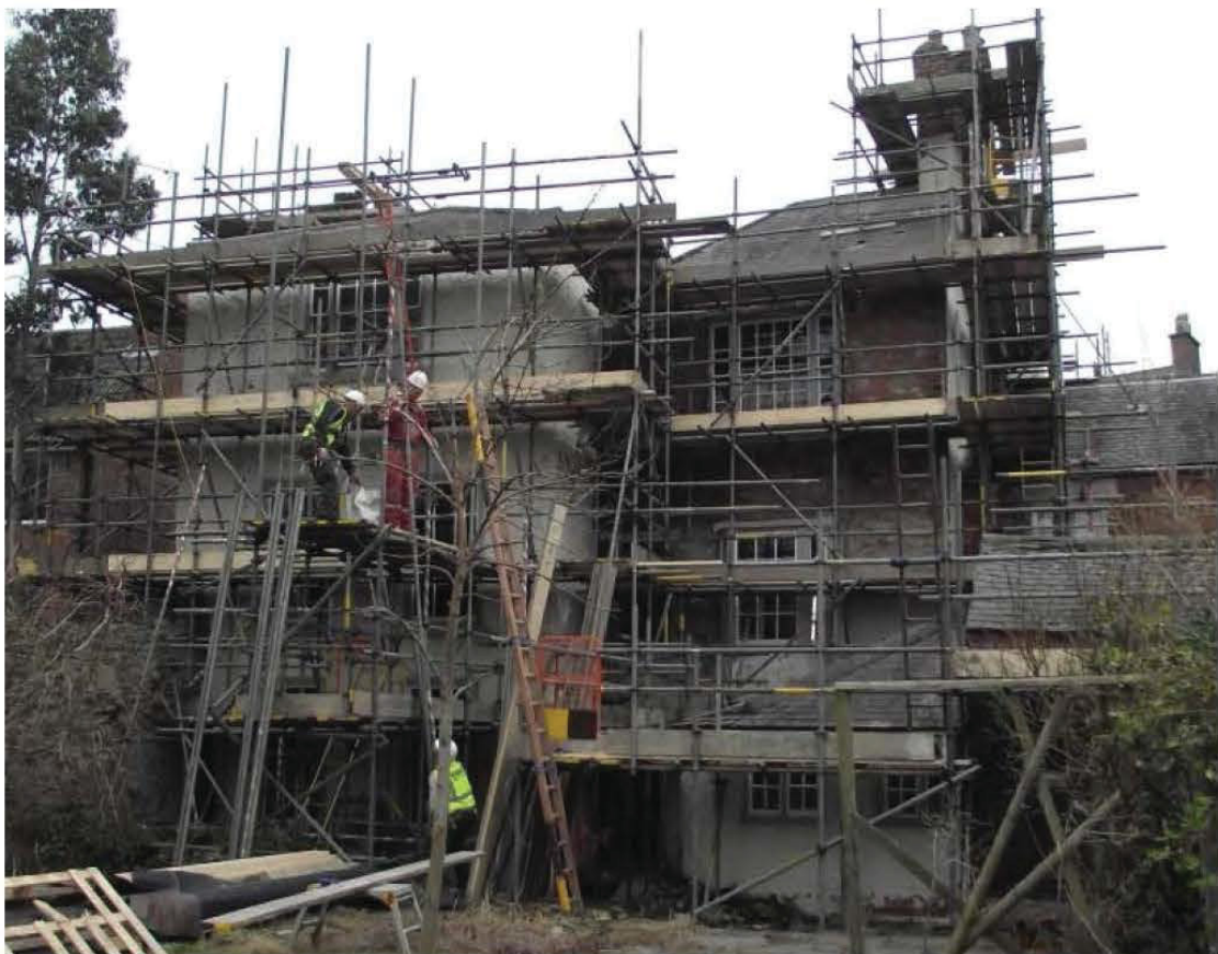
Plate 10: Rear elements, west-facing (rear) elevation, during works (view, no scale)
