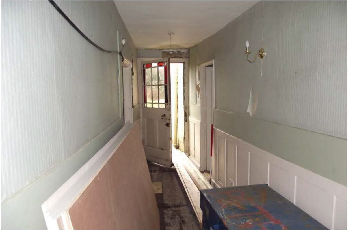
Plate 38: Southern rear element, ground floor, central hallway (1m scale)
