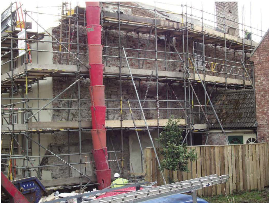
Plate 9: North-facing (side) elevation, during works (view, no scale)
