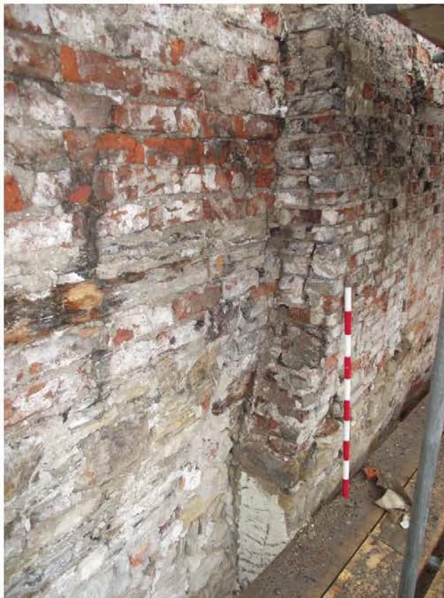
Plate 14: North-facing (side) elevation, projecting chimney masonry (1m scale)
