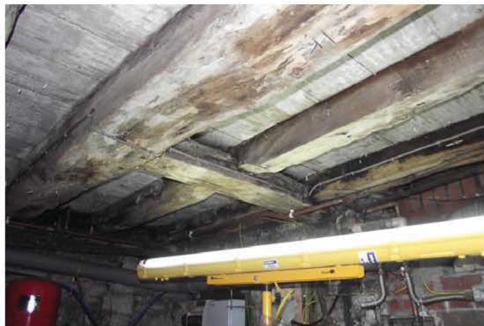
Plate 32: Cellar, ceiling (floor timbers above) (view, no scale)
