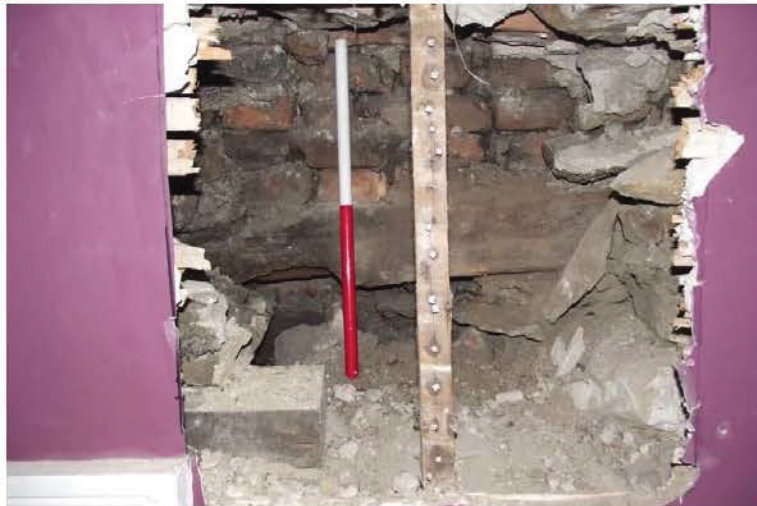
Plate 71: First floor, Bedroom 3, central enabling hole in west wall (0.5m scale)
