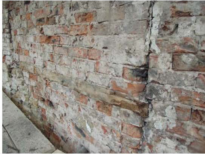
Plate 19: North-facing (side) elevation, northern element, brickwork incorporating timber (view, no scale)
