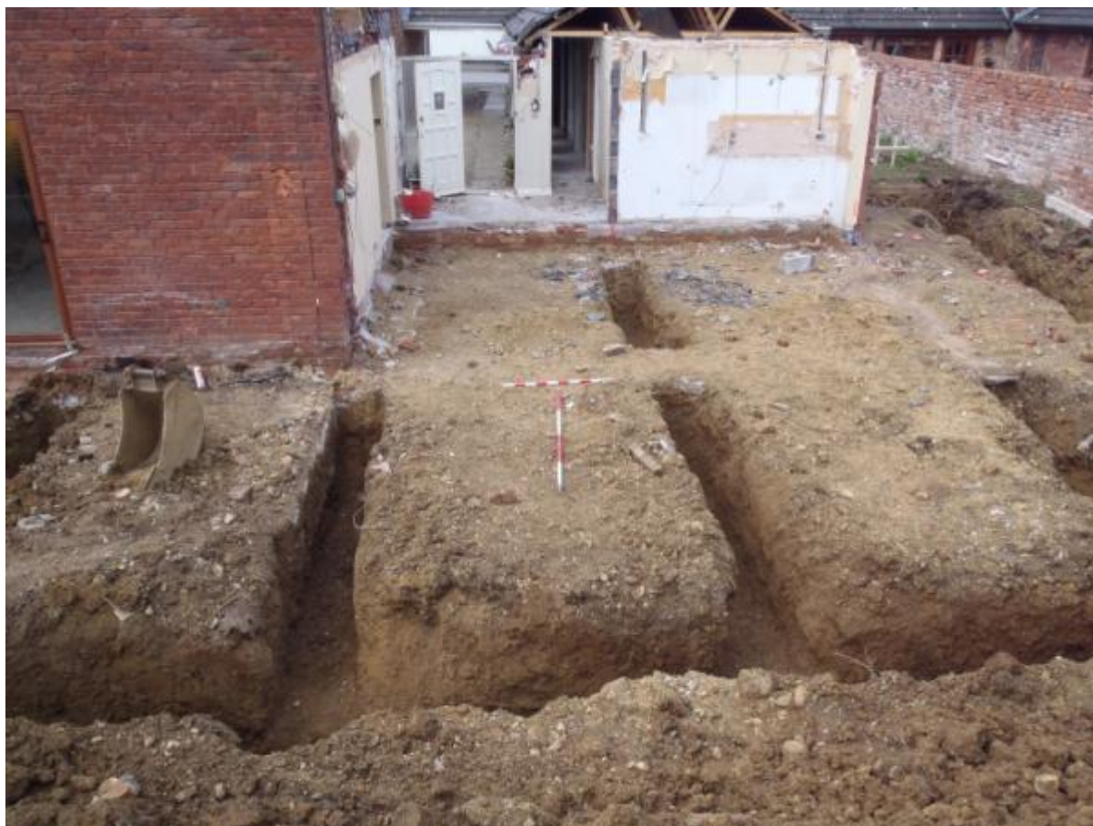
Plate 2: General view of excavated foundations, facing east (Scales 2 & 1m)
