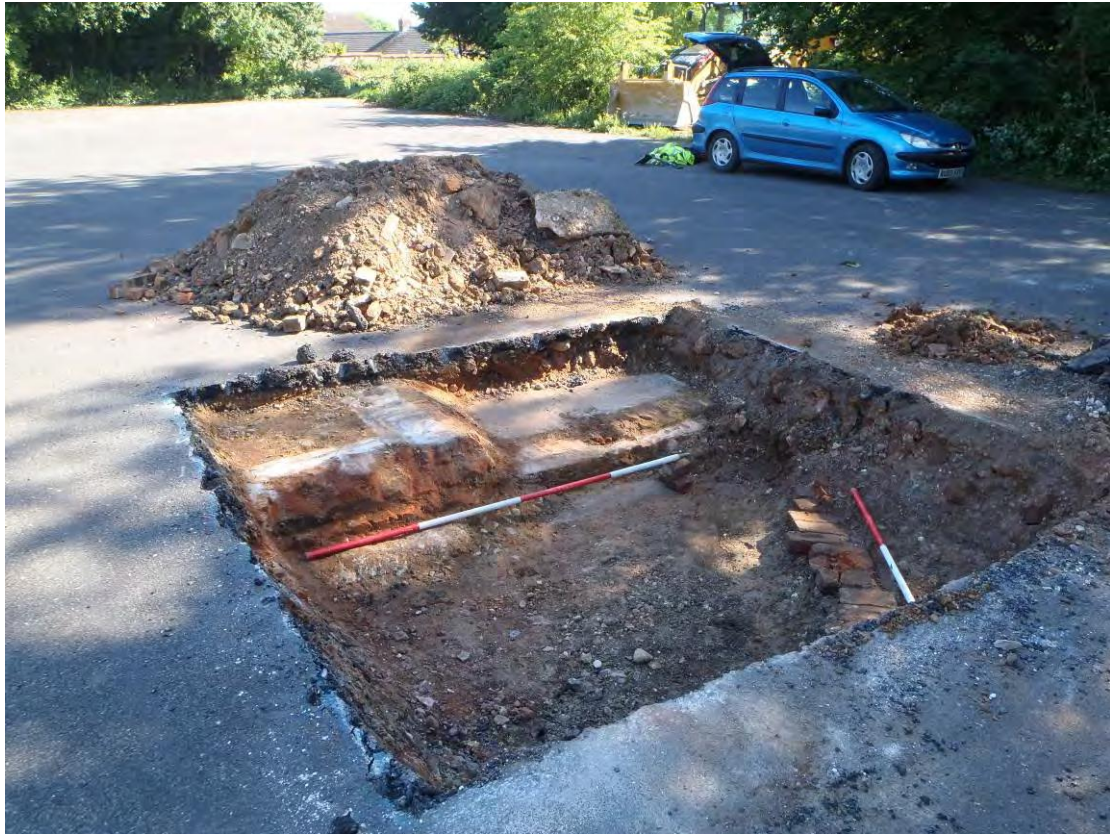
5: Trench 3, view north-east showing (from left to right) Walls (10), (7) and (12) of Victorian Hyde House
