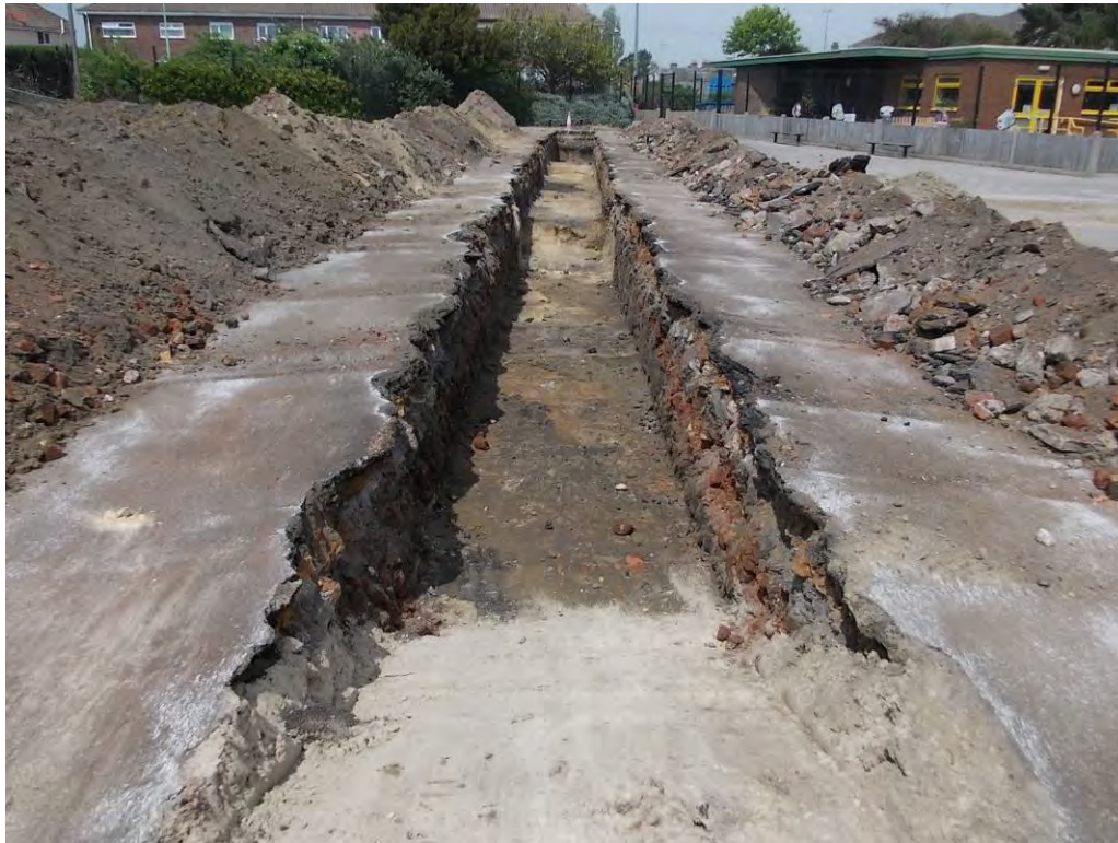
Plate 7: Trench 4: view north with large Quarry Pit [15] in foreground.
