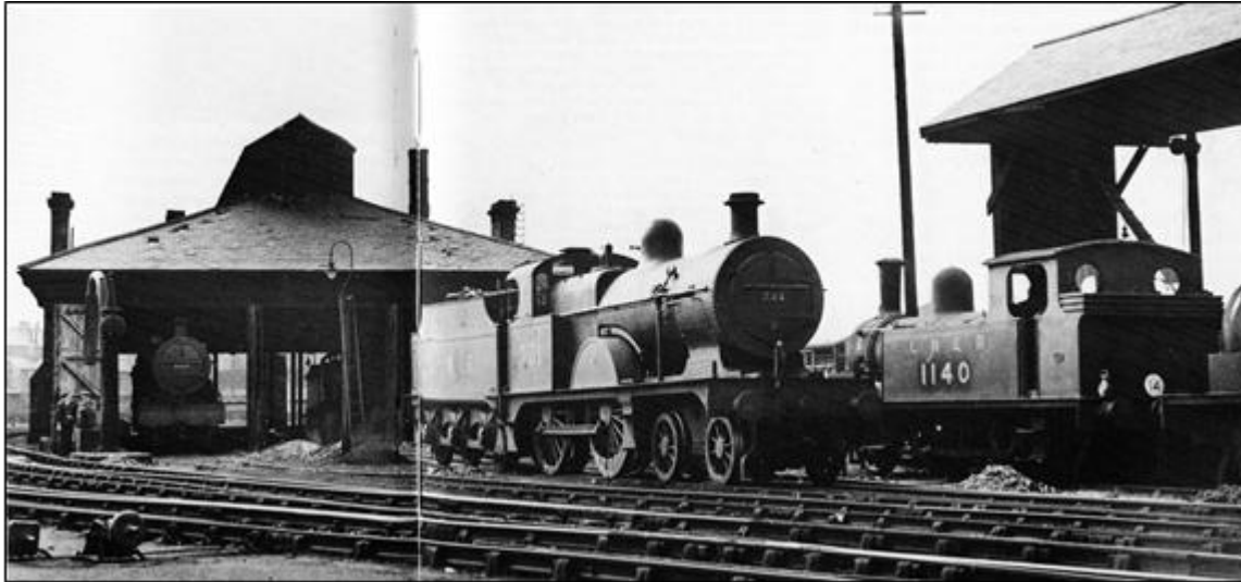
Plate 10-1 Photograph (taken after c. 1923) of the 1841 Engine Shed, showing clerestory roof (Hoole 1983, 71)
