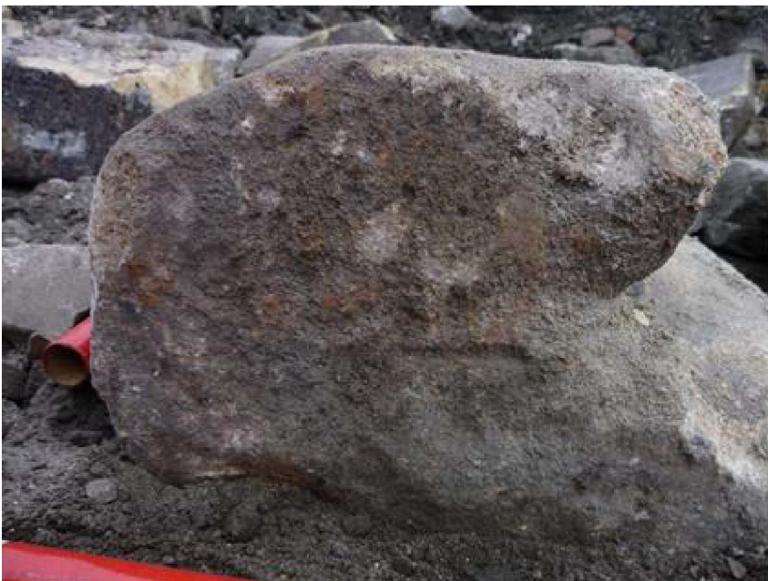
Plate 8-10 Possible mason's mark on end of rebated window sill from RH3
