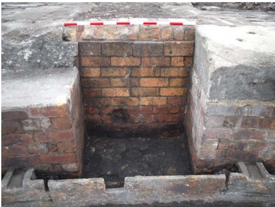
Plate 5-36 RH3, turntable well access pit [783], looking south-west (scale 1m)
