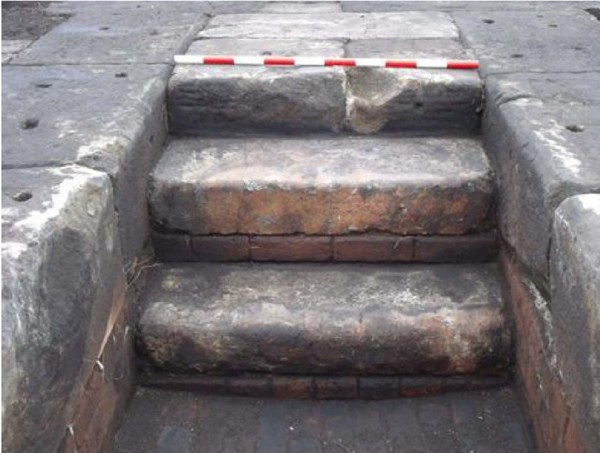
Plate 5-21 RH2, detail of stone steps in inspection pit [529], looking NNE towards central turntable (scale 1m)
