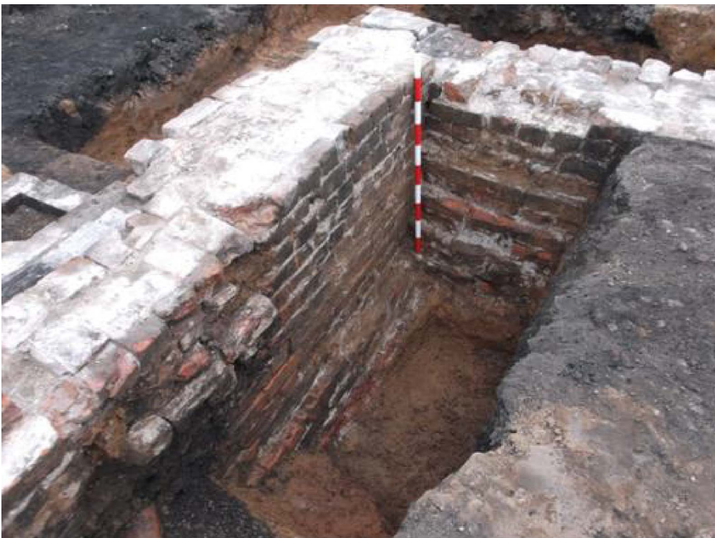
Plate 5-2 Detail of 1841 Engine Shed external wall footings [945], south-west corner, looking south-west (scale 1m)
