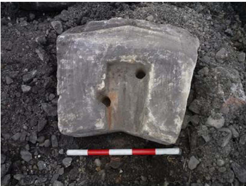
Plate 8-16 Roof (rafter) support coping stone from RH2 (scale 0.50m)
