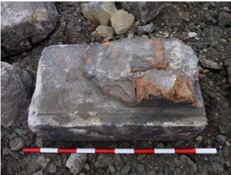
Plate 8-2 Underside of coping stone from RH2, with remnants of brickwork attached (scale 1m)
