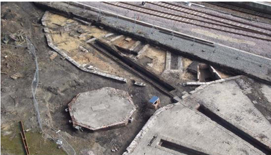
Plate 5-12 RH1 and RH2 and octagonal building [897], overview (from access platform), looking south-east
