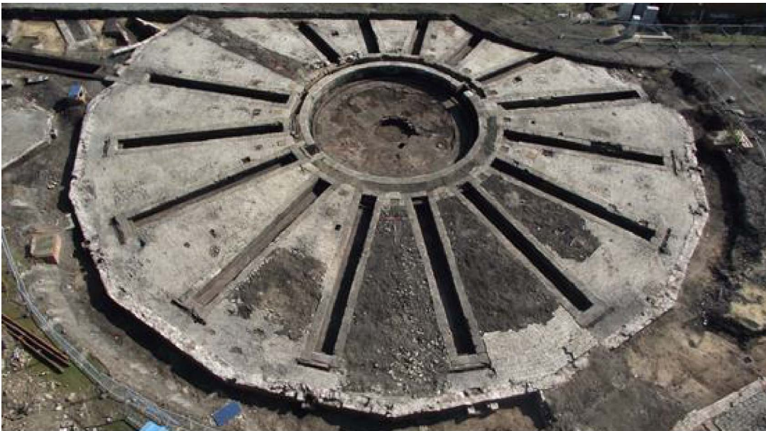
Plate 5-14 RH2, overview (from access platform), looking south-east
