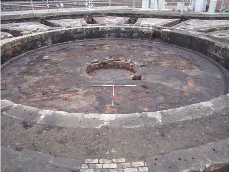
Plate 5-15 RH2, turntable well, looking south-east (scales 2 x 2m)
