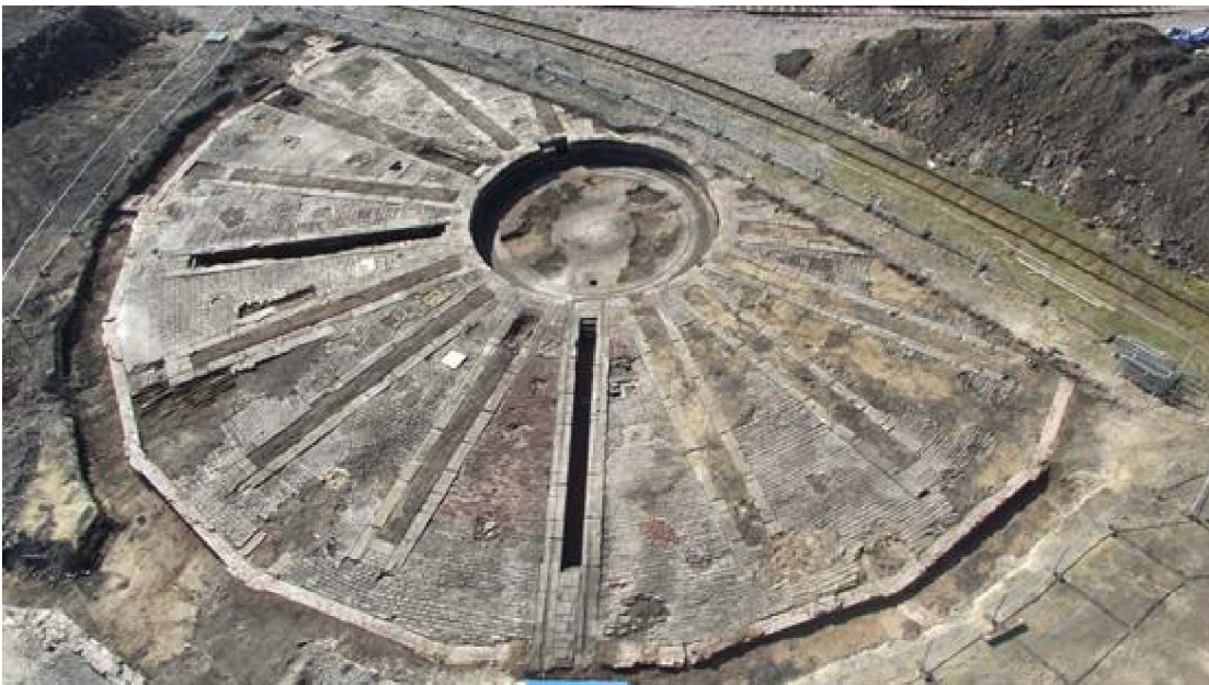
Plate 5-28 RH3, overview (from access platform), looking south-west
