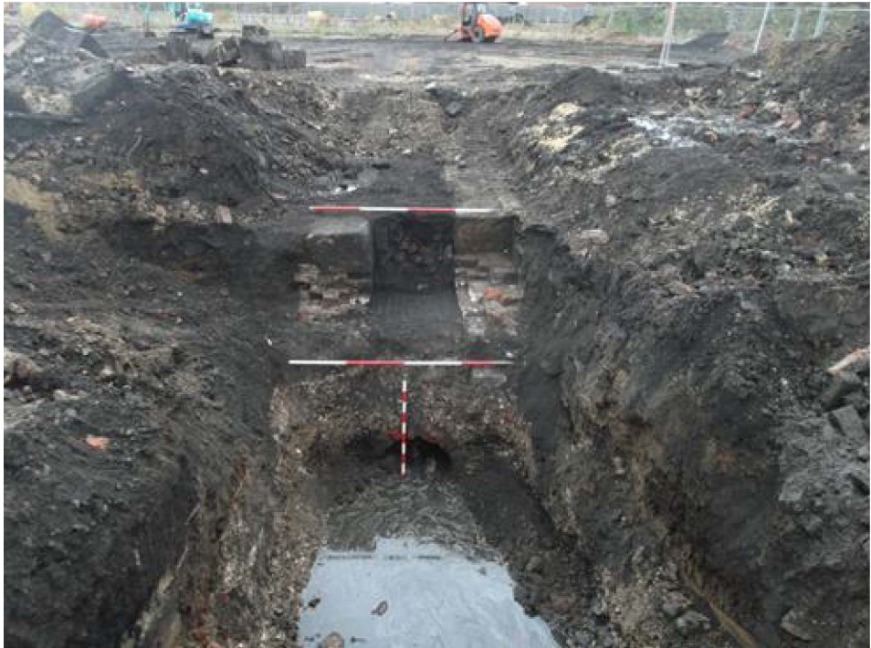
Plate 5-39 RH3, external inspection pit [1238] with culvert [1240] below, looking southwest (scales 2 x 2m, 1 x 1m)
