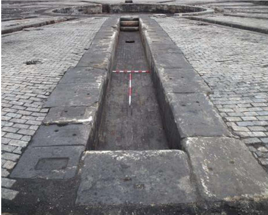
Plate 5-19 RH2, inspection pit [529], looking NNE towards central turntable (scales 2m and 1m)
