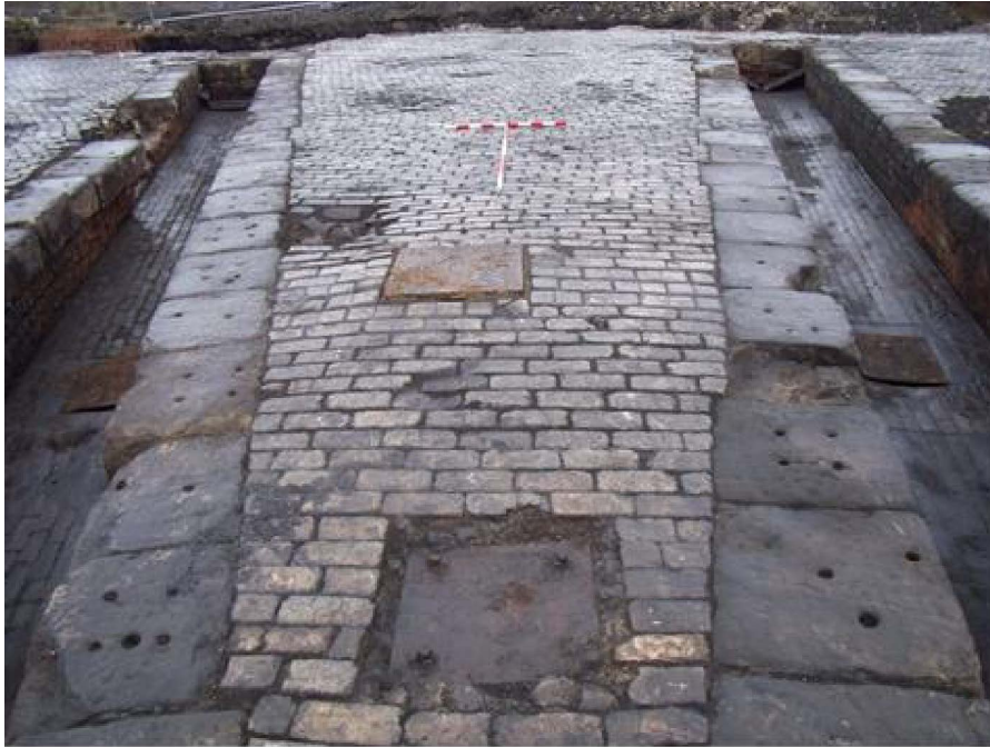
Plate 5-23 RH2, scoria brick floor surface detail [733], with stone pad for roof support [746] and manhole [747], looking south-west (scales 2m and 1m)
