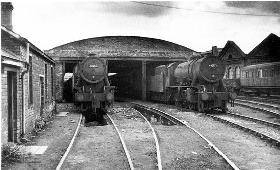
Plate 10-2 Photograph (taken mid-20th century) of the 1841 Engine Shed, showing arched brick roof (Rose 1994, 21)
