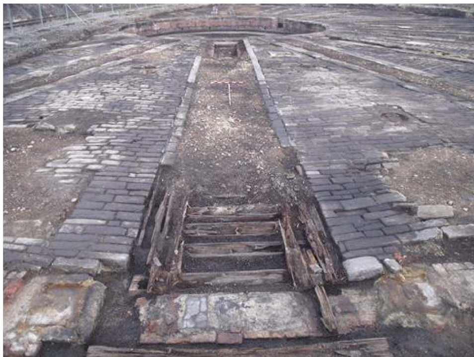
Plate 5-40 RH3, inspection pit [653] show timber track elements [798], looking north (scales 2m and 1m)
