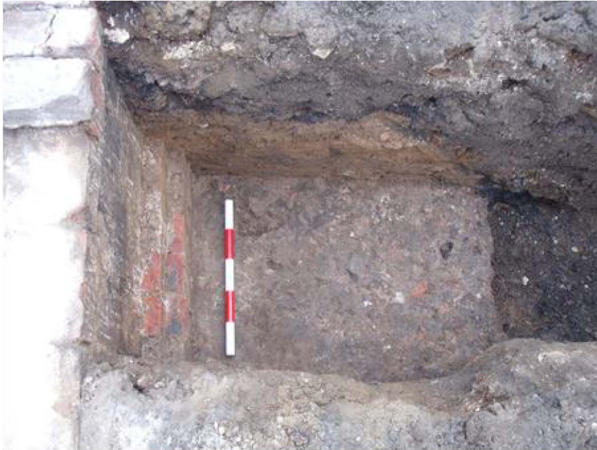
Plate 5-29 RH3, concrete slab footing [863] for external wall [708], looking east (scale 1m)
