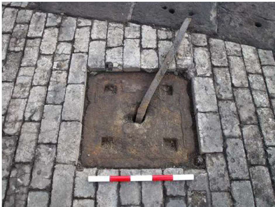
Plate 5-24 RH2, stone support pad [746], looking east (scale 0.5m)
