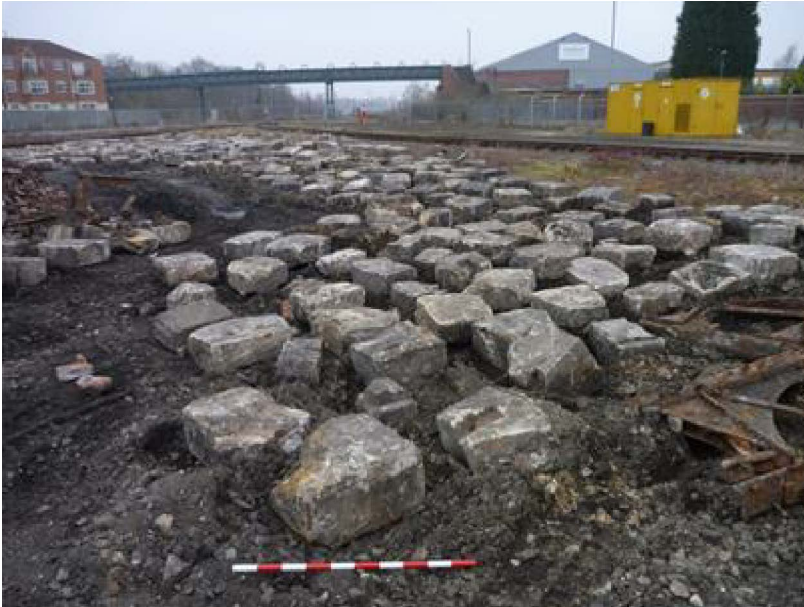
Plate 8-1 General view of stonework from RH2 (scale 1m)
