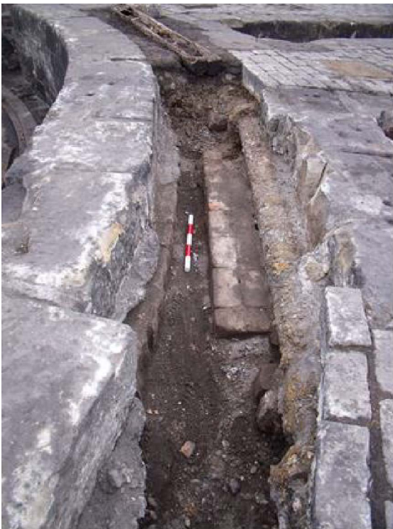
Plate 5-22RH2, service trench with cast iron water pipe, shows original length of inspection pit, looking WNW (scale 0.5m)
