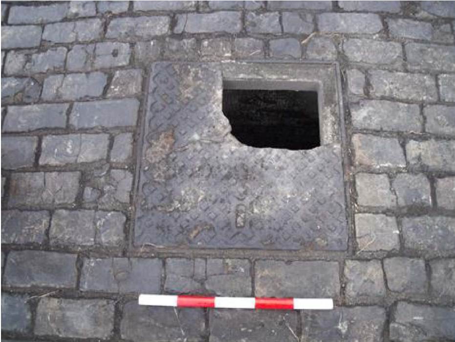
Plate 5-25 RH2, detail of manhole [747], looking south-west (scale 0.5m)
