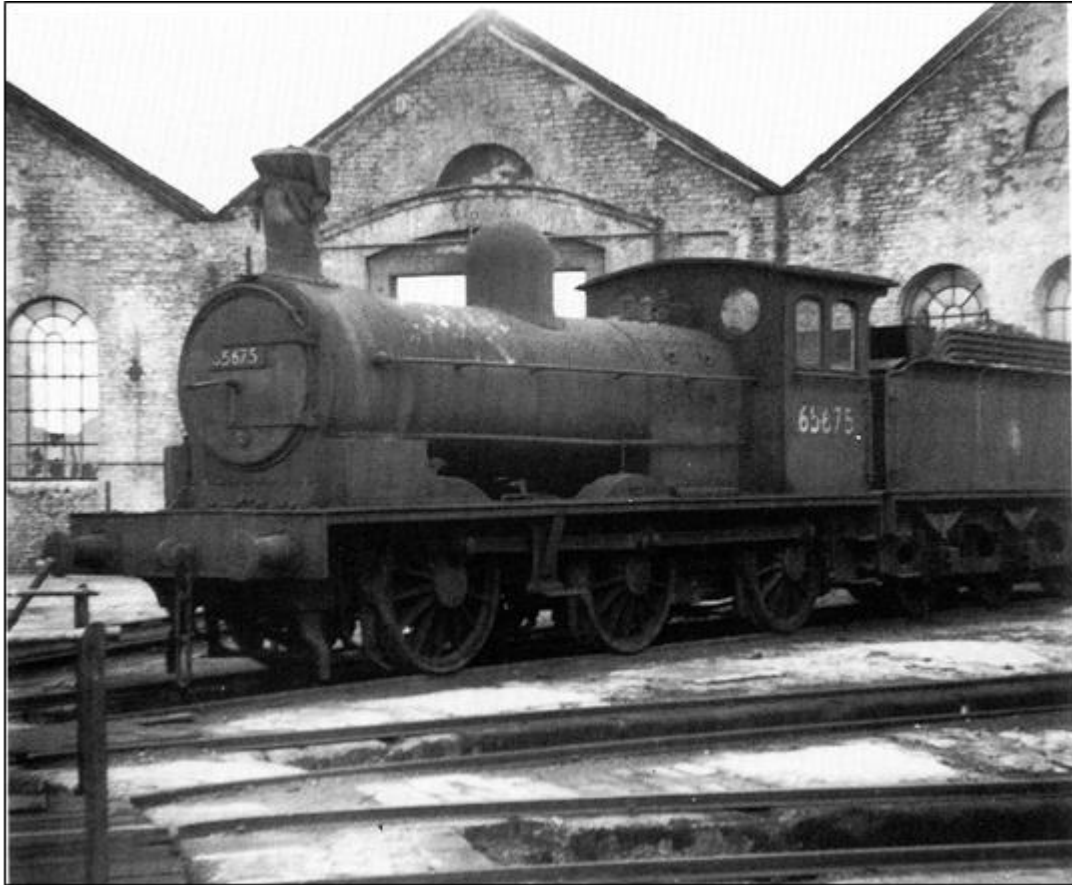
Plate 10-9 Photograph (taken mid-20th century) showing interior of RH3 interior, with detail of squared entrance with segmental arch in rearground (Rose 1994, 80)
