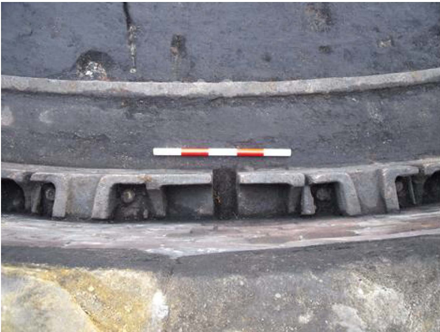
Plate 5-34 RH3, detail of perimeter track [778] and locking mechanism [779] (scale 0.5m)
