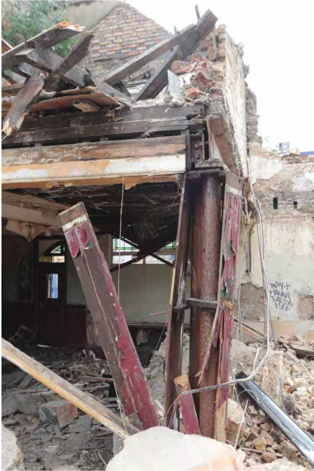
Plate 30 Iron column and beam in Bar Area GF1, looking south
