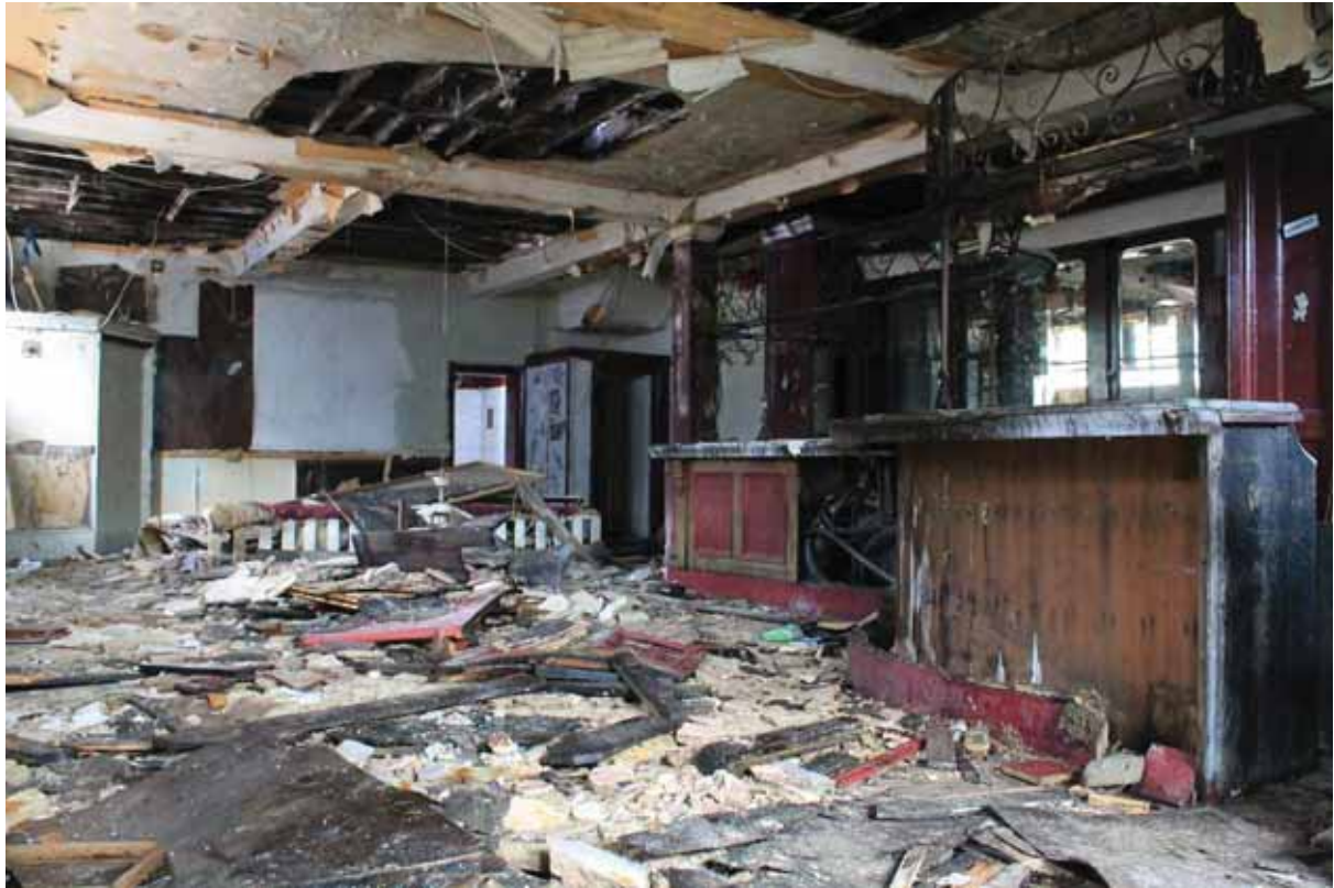
Plate 13 Bar Area GF1, looking west
