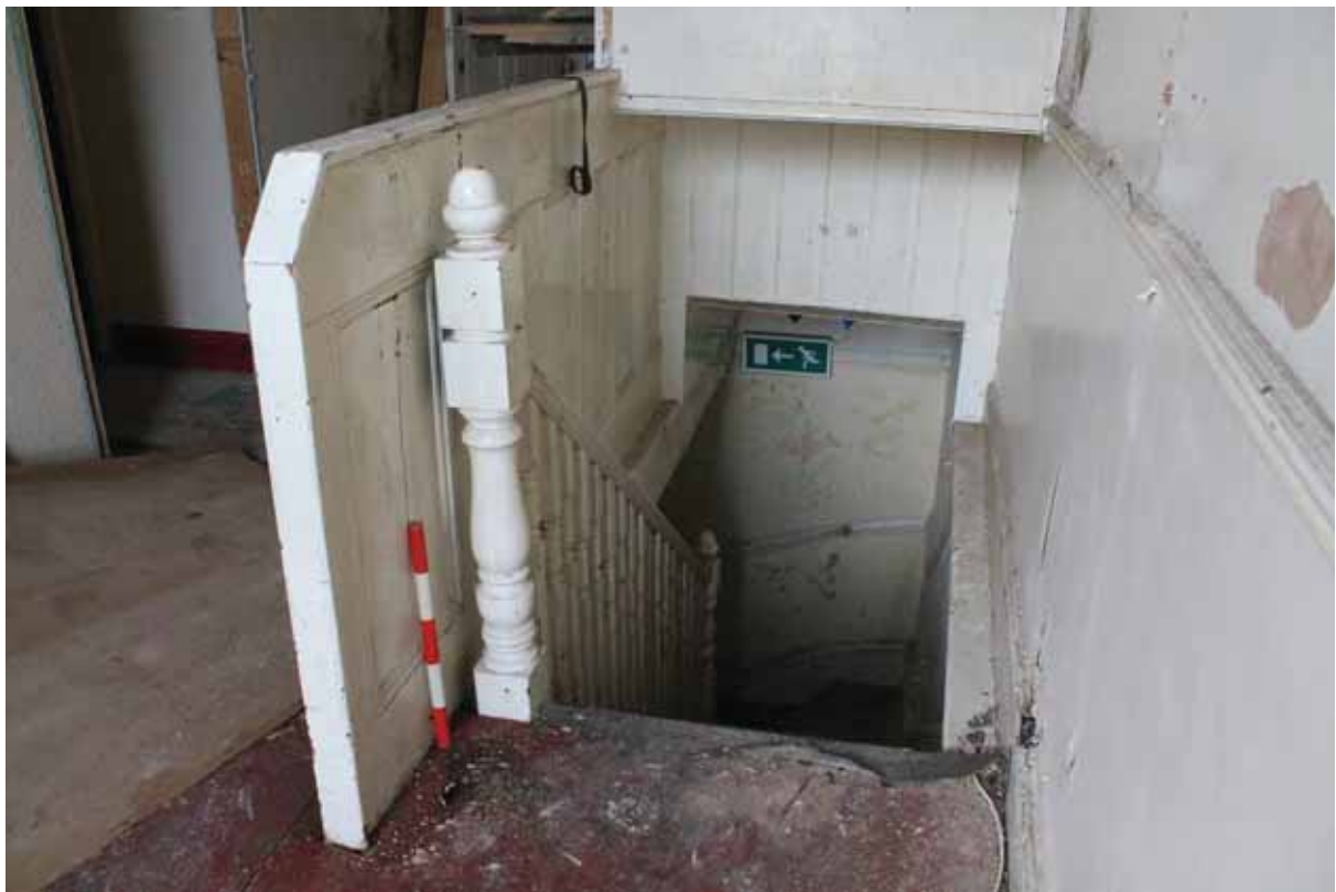
Plate 23 Staircase, balustrade and first floor landing, looking west
