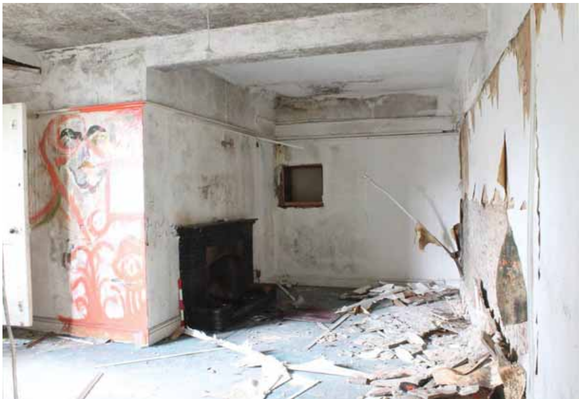
Plate 21 Room GF5, looking south
