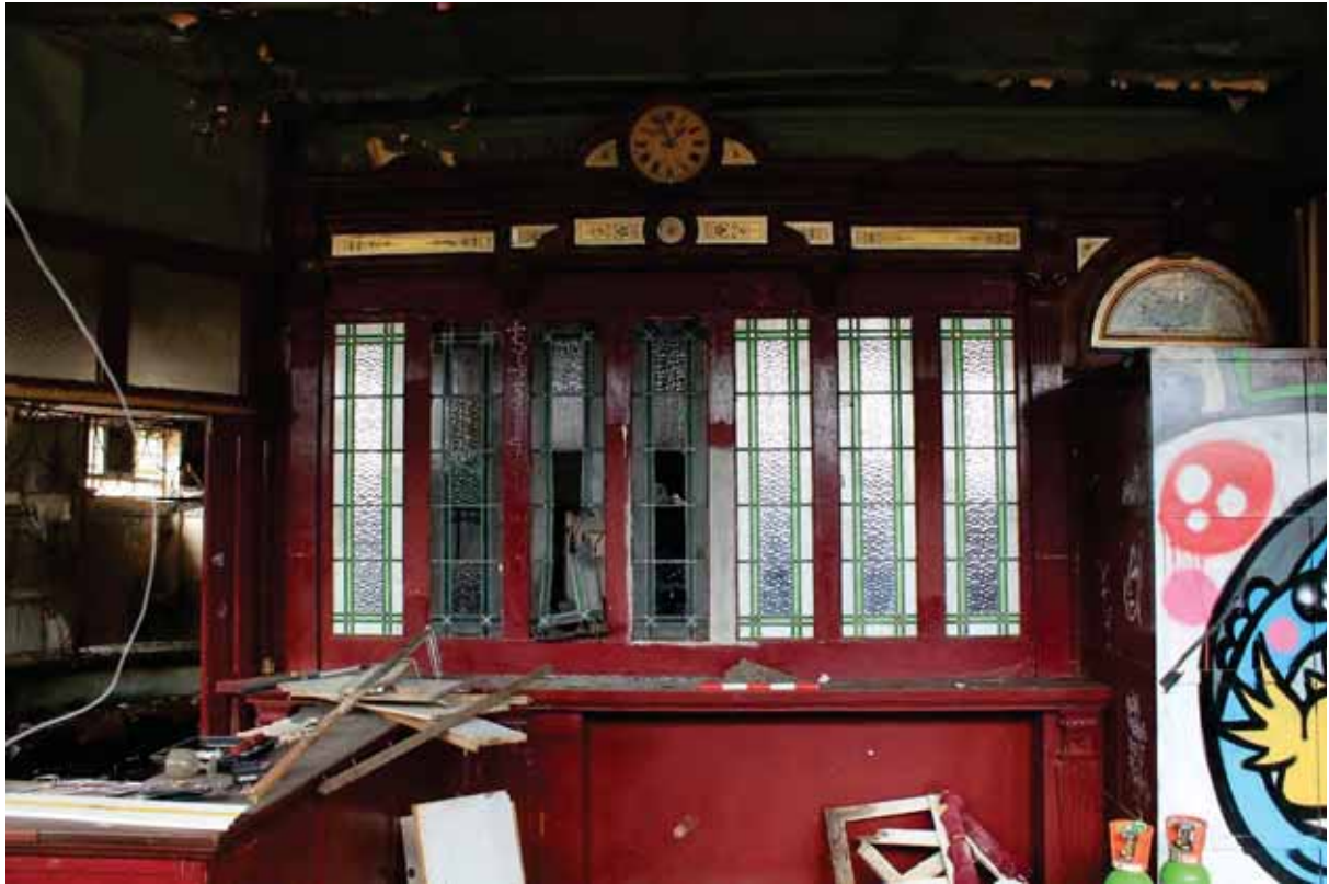
Plate 17 Part glazed partition wall in Bar GF2, looking west
