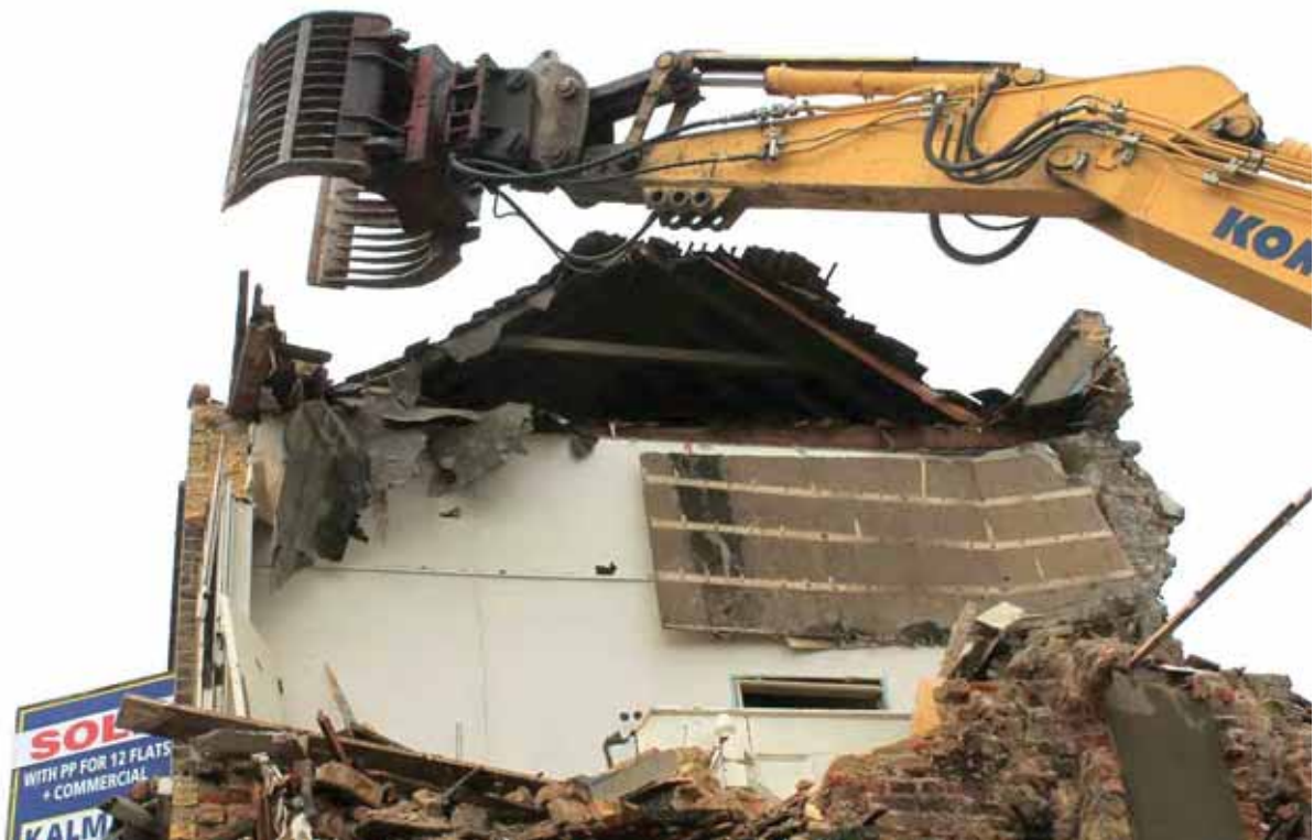
Plate 32 Mid 20 th century roof structure over the eastern (Phase 2) part of the building, looking south
