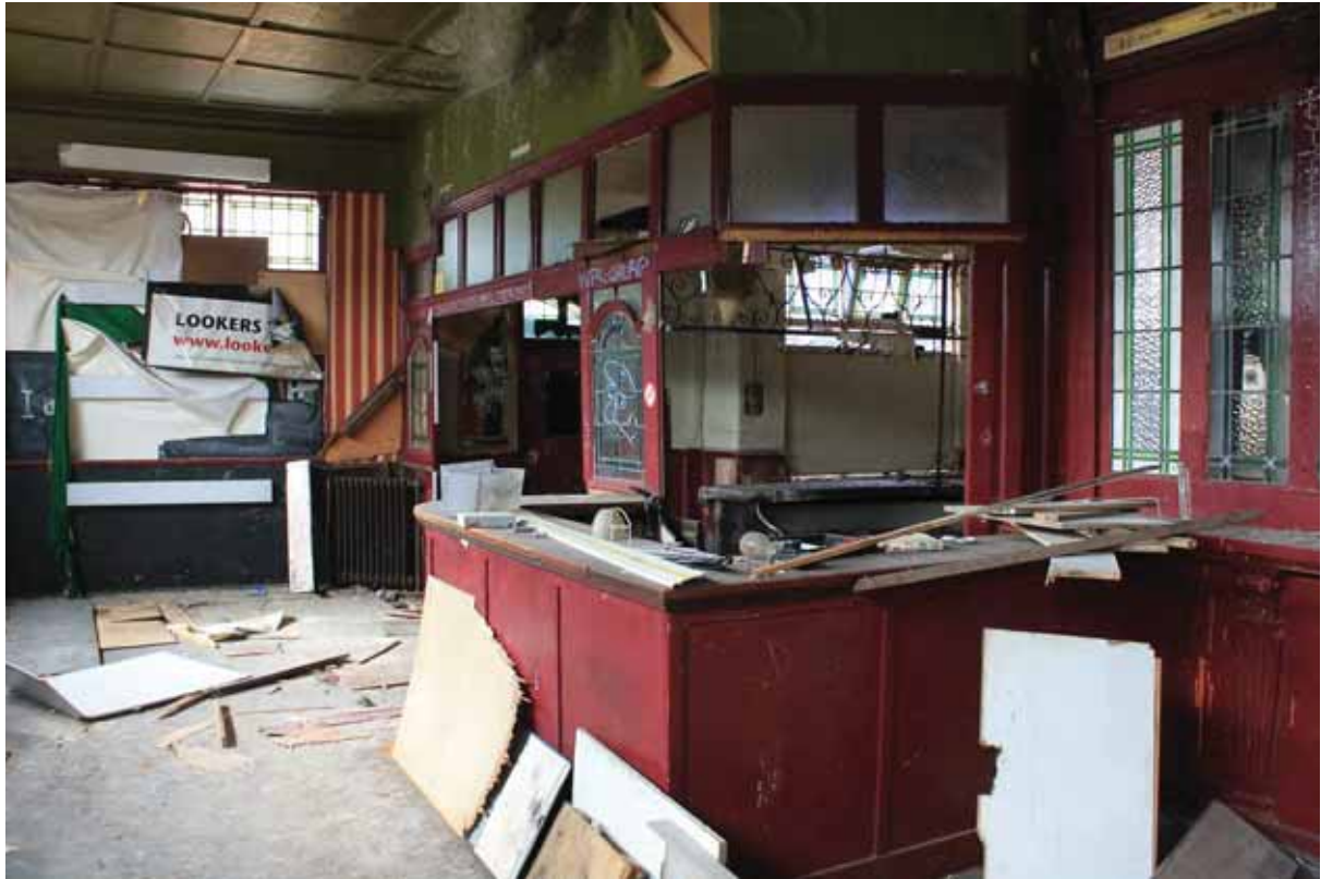
Plate 15 Bar Area GF2, looking south
