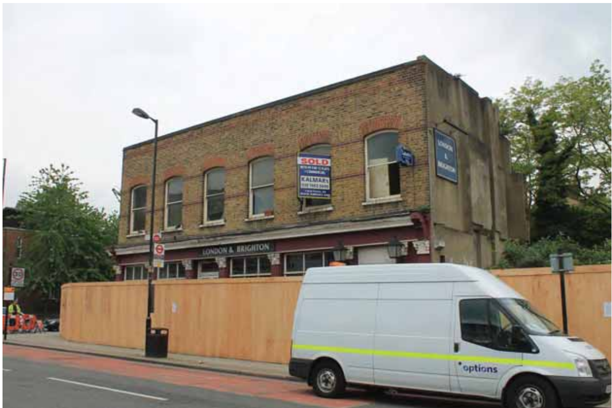
Plate 2 London and Brighton Asylum Road façade, looking south-west
