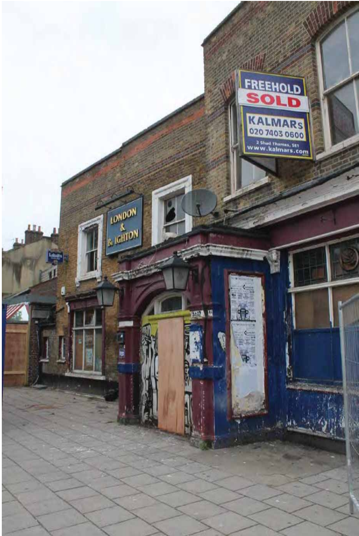
Plate 5 Queens Road (southern) elevation, looking north-west
