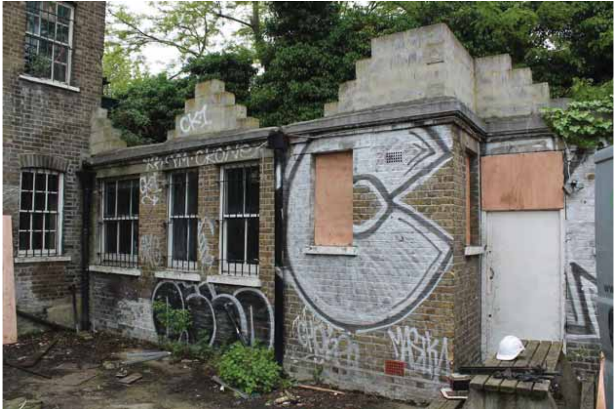
Plate 11 Rear (north) extension, looking south-west
