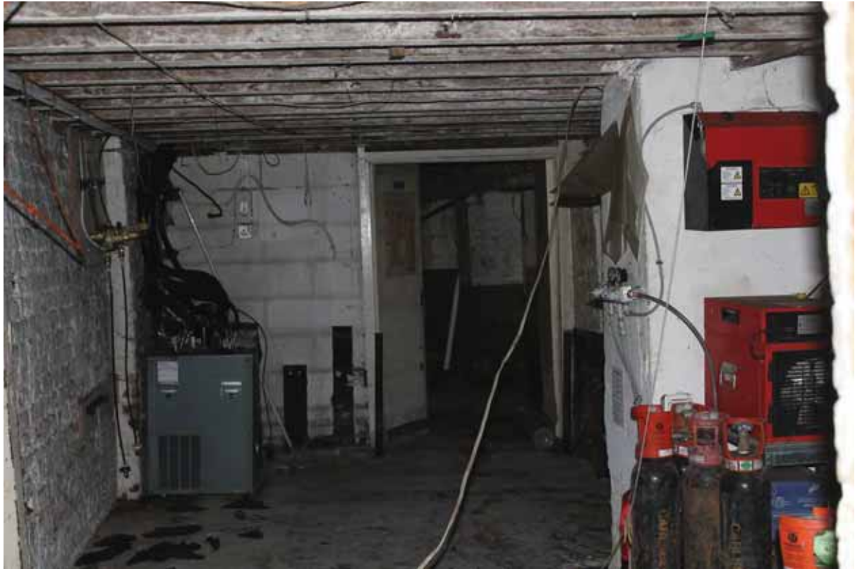
Plate 22 Basement, looking south
