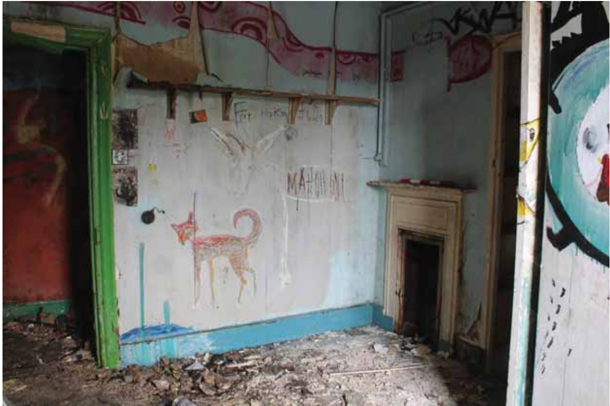
Plate 20 Room GF4, looking south-west
