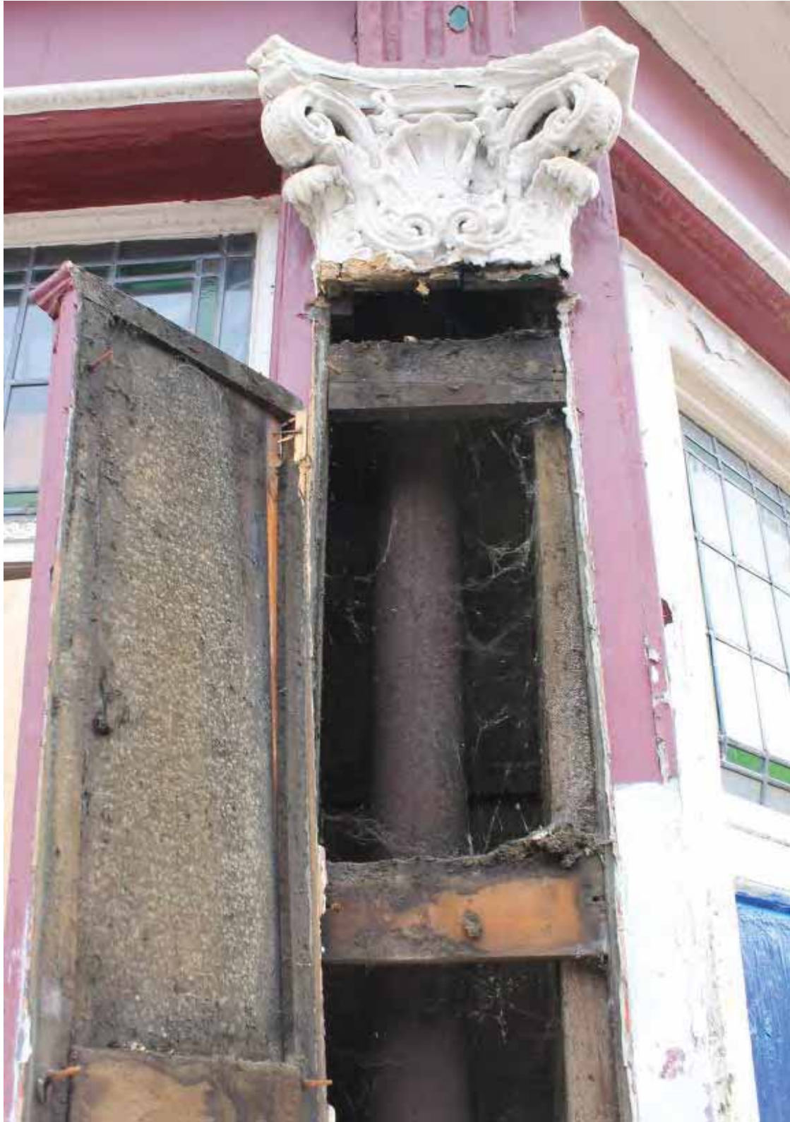
Plate 28 Box Pilaster and internal cast-iron column, looking north-west
