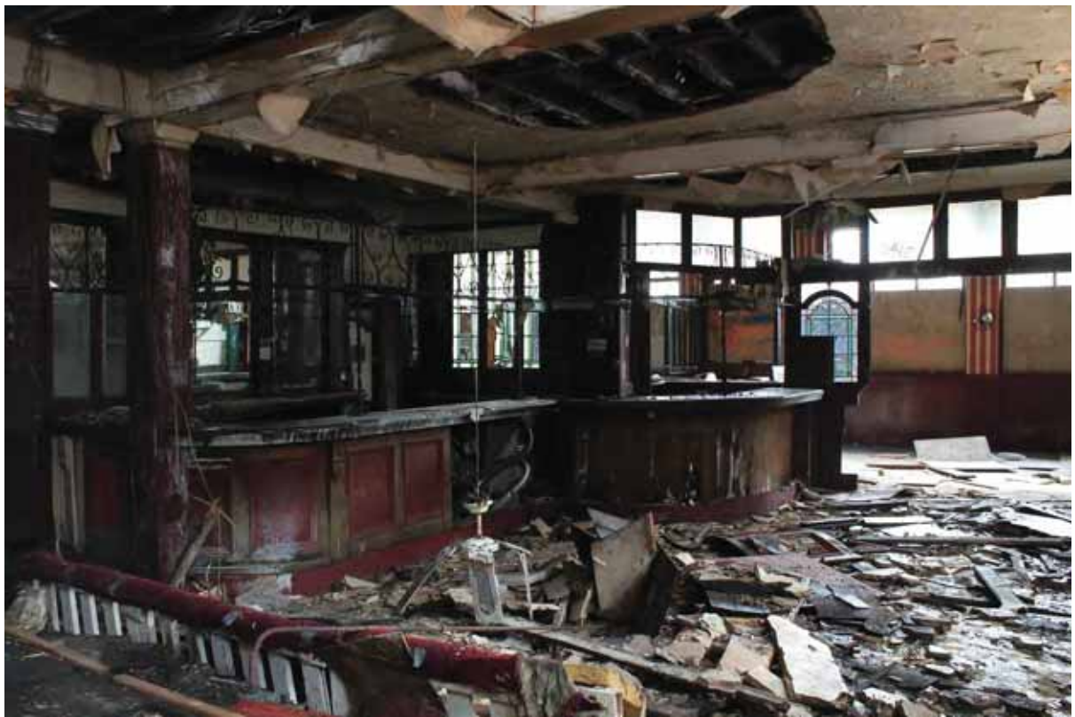
Plate 14 Bar Area GF1, looking east
