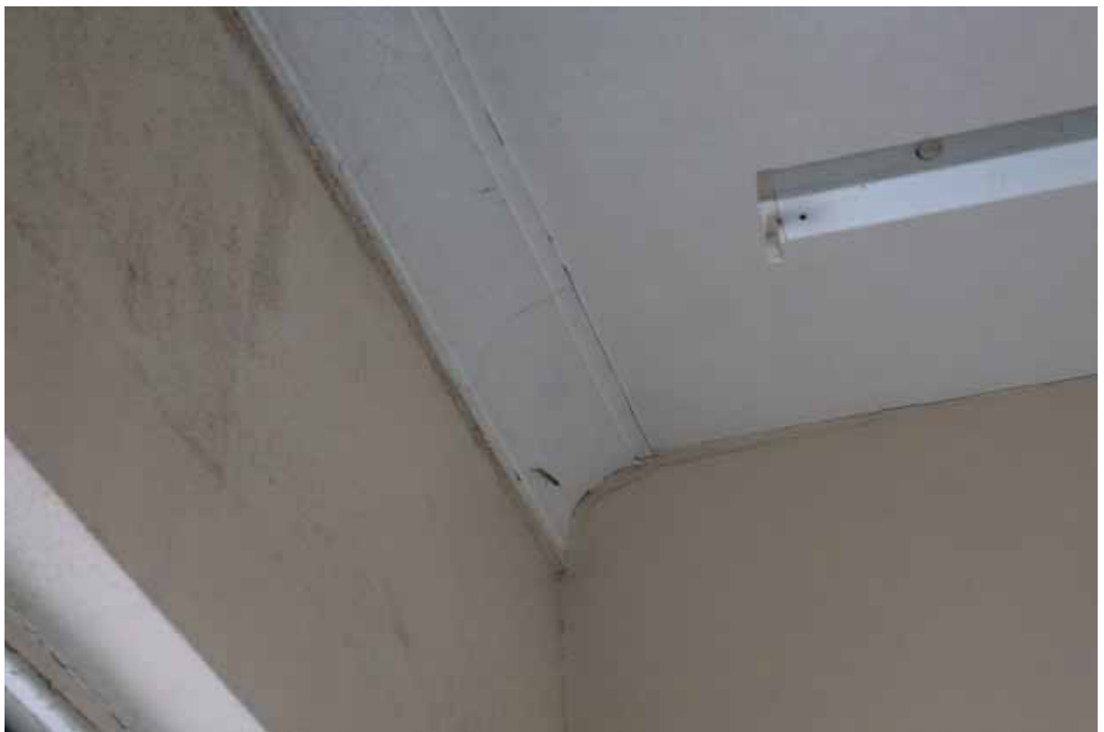
Plate 25 Plain cavetto cornice in FF2, looking south-east
