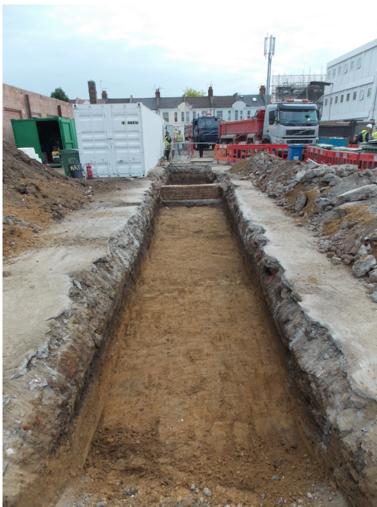
Plate 3: Overview of Trench 7, Facing Northeast
