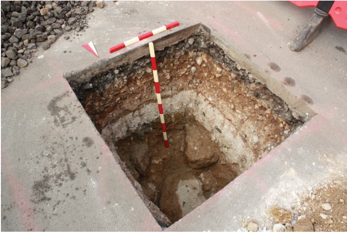
Plate 5. D1/8. Trial Hole2. Rubbly stone infill of abutment in base [7], overlain by white chalk levelling layer [6]. Scales 1m and 0.5m, looking SSW.
