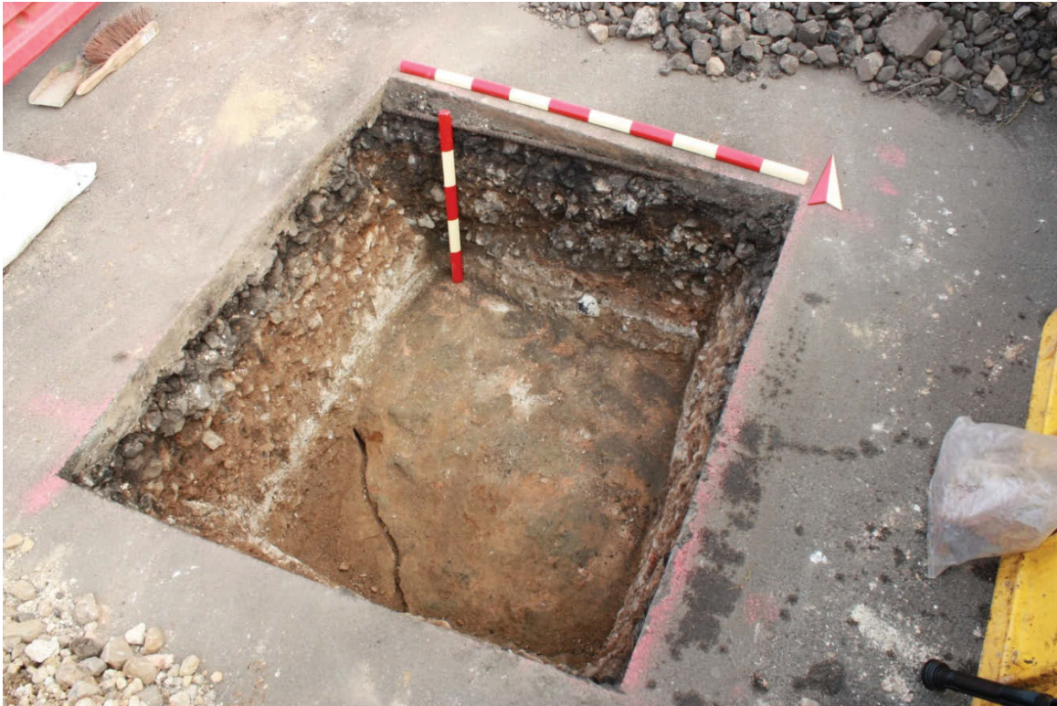
Plate 3. D1/10. Trial Hole 1. Inner back of stone arch [16] in base of trench. Scales 0.5m and 1m looking N.
