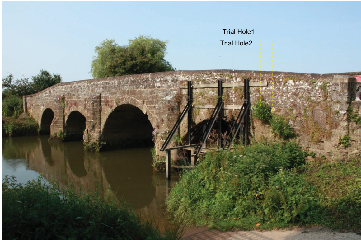
Plate 1 D1/23. East side of Old Swan Bridge, Pulborough crossing the River Arun, looking SW. The approximate positions of the trial holes is marked. Note 1990s steel supports below arch.
