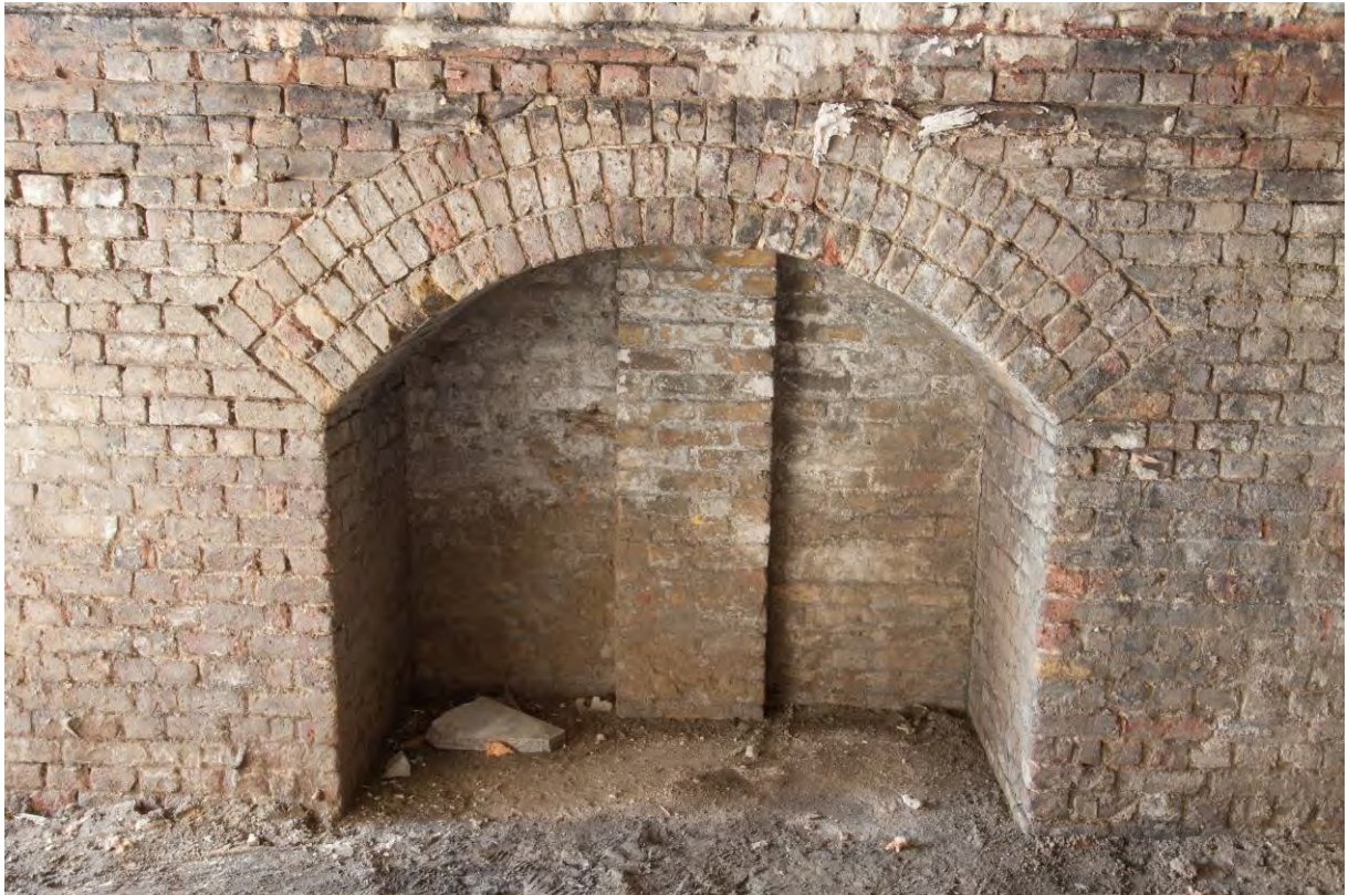
Plate 21 Transverse arch in Arch 11 looking west (RWV13 D101 8368-2)
