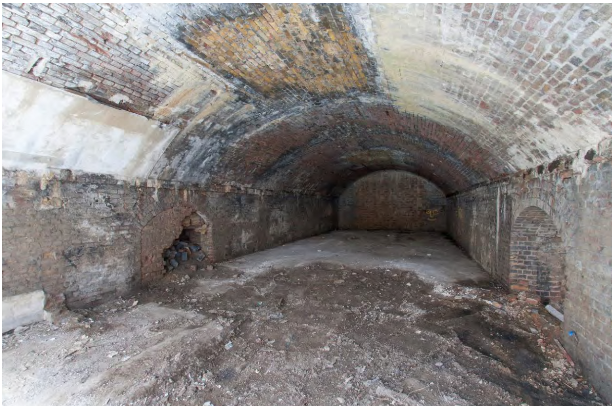
Plate 30 Arch 16 looking north (RWV13 D101 8328-2)
