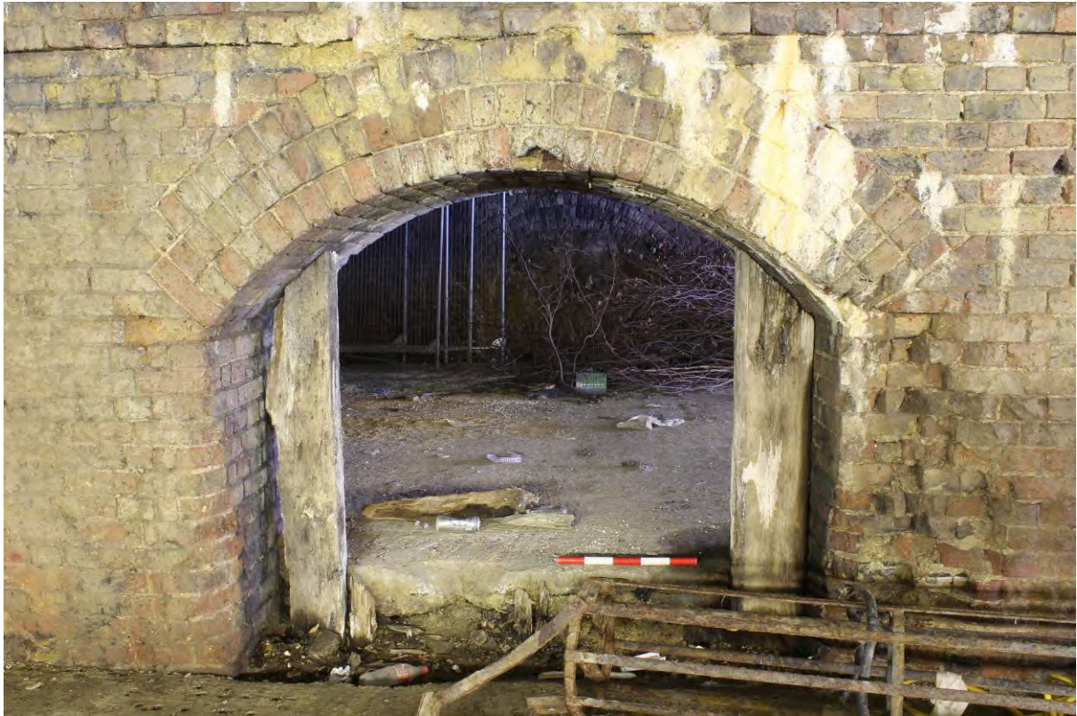
Plate 35 Transverse arch within viaduct Arch 17
