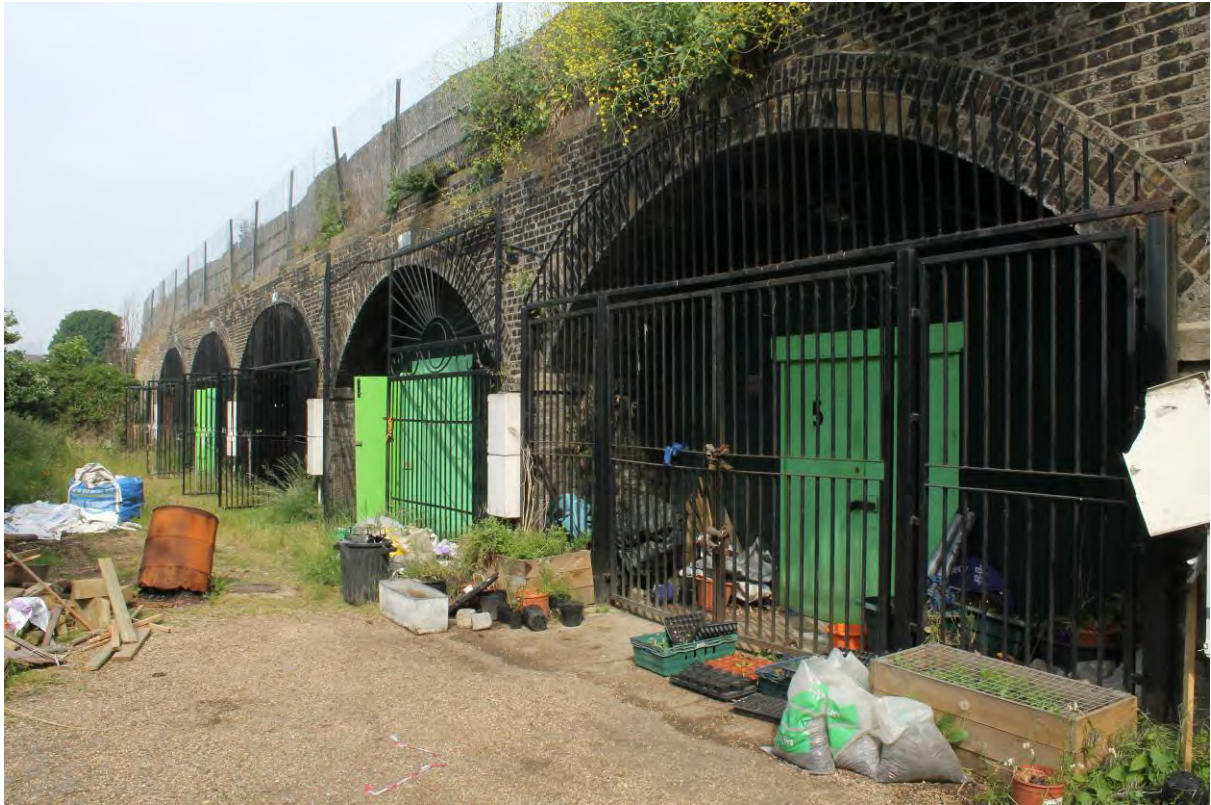
Plate 5 Apple Tree Yard, Arches 1-5 looking west
