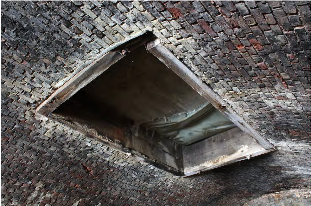
Plate 25 Timber-lined coal drop within Arch 13
