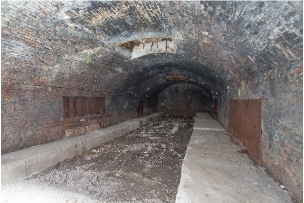
Plate 29 Arch 15 looking north (RWV13 D101 8340-2)
