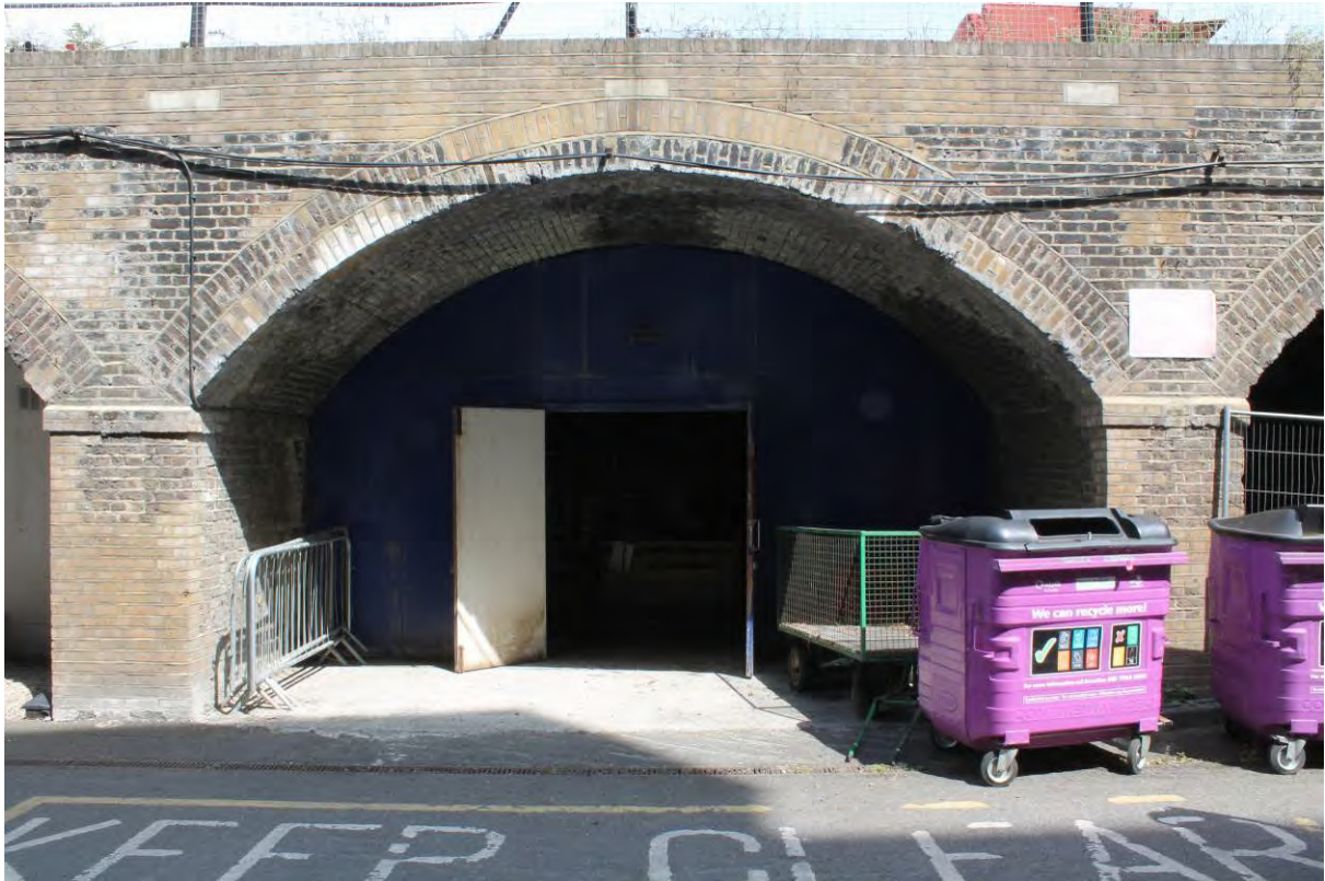
Plate 33 Arch 17 looking north
