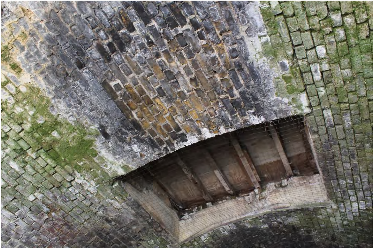
Plate 37 Later inserted opening into former blocking, Arch 19
