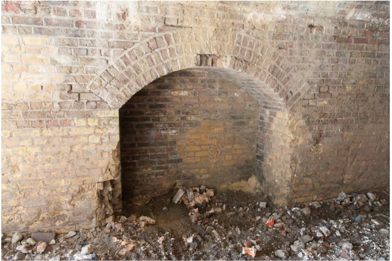
Plate 23 Transverse arch in Arch 12 looking west (RWV13 D101 8359-2)
