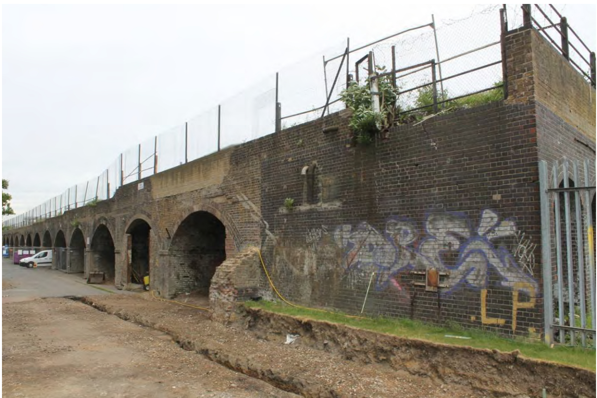
Plate 2 Viaduct at the eastern end looking west
