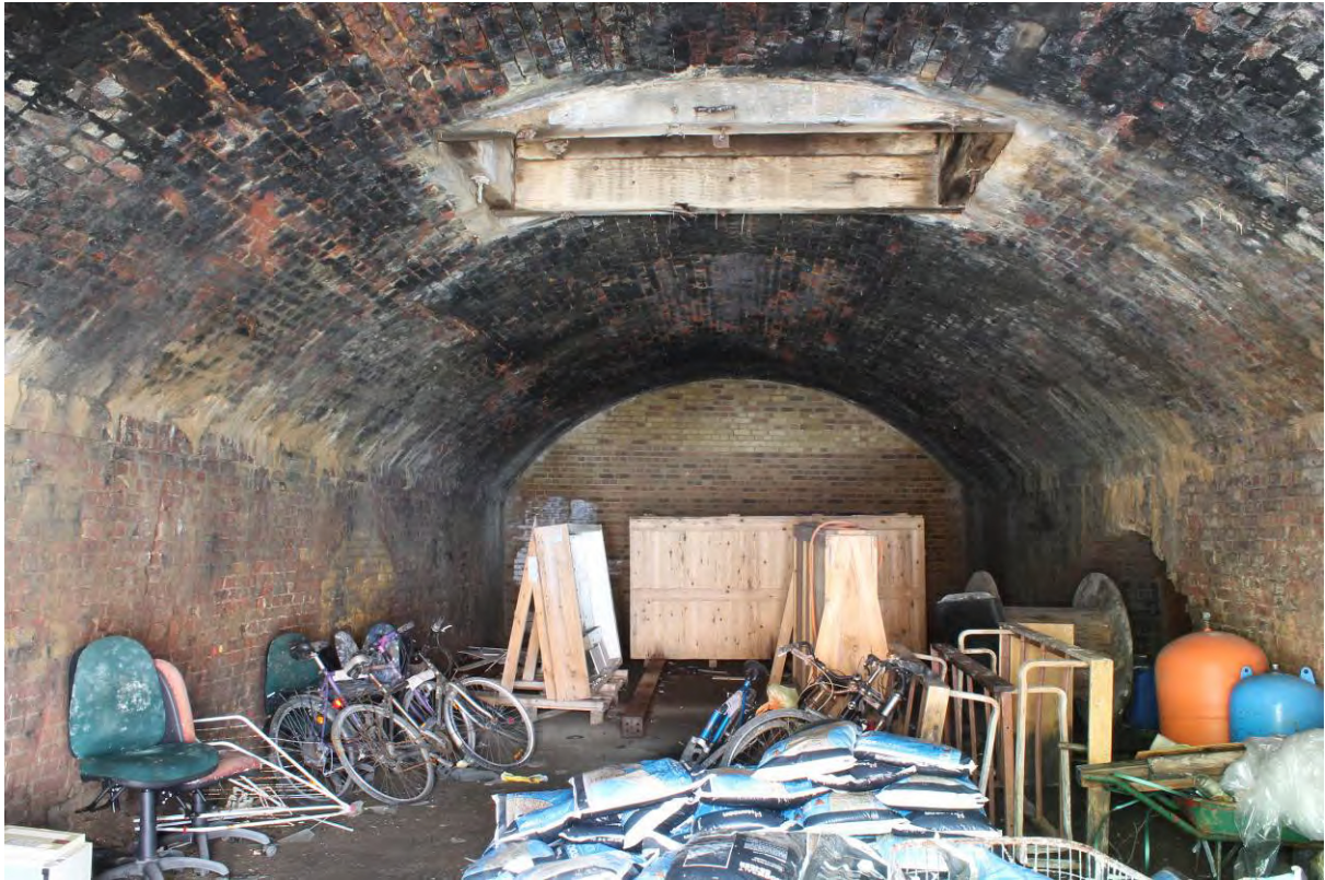
Plate 39 Arch 20 looking north
