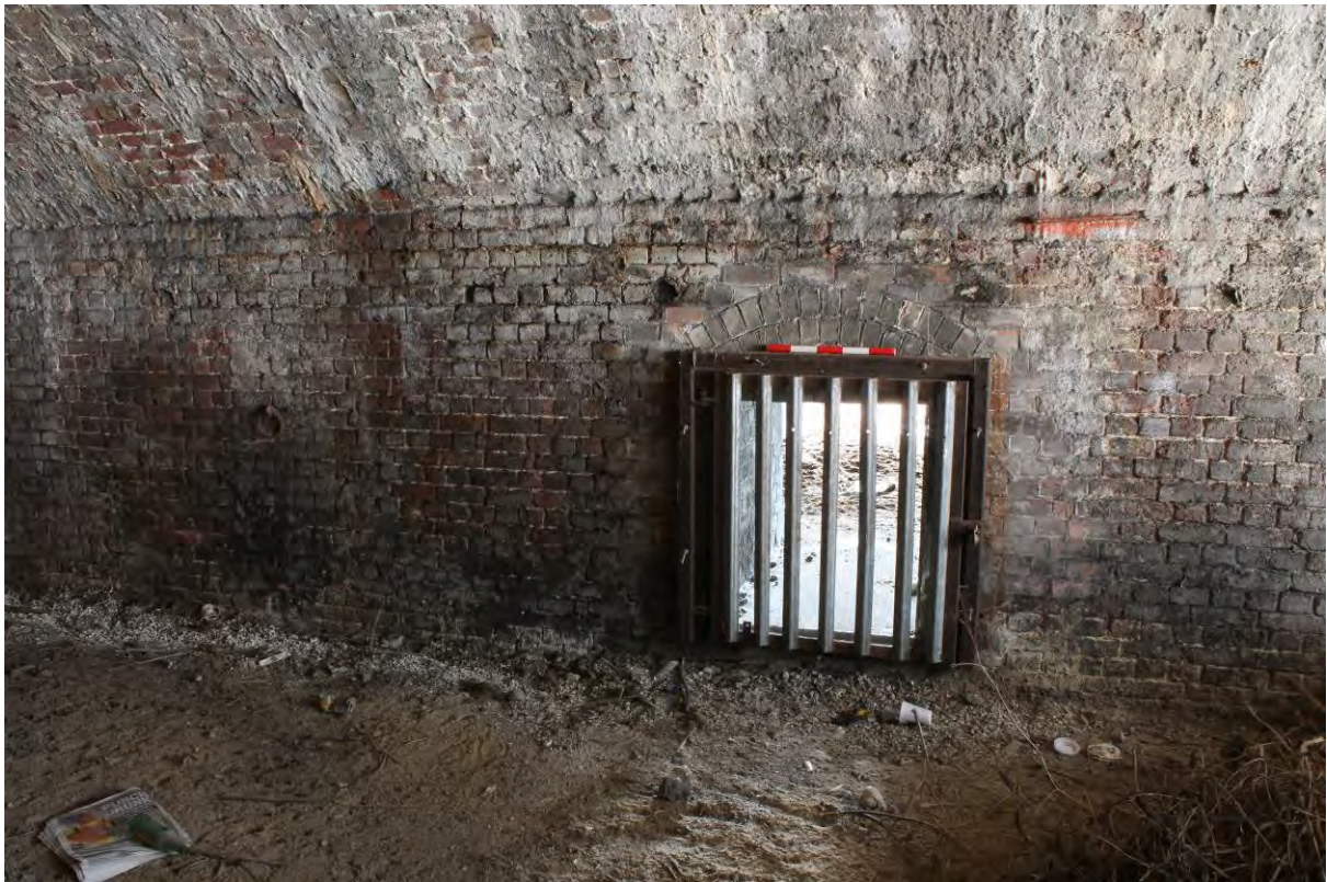
Plate 46 Inserted opening in Arch 25 east wall
