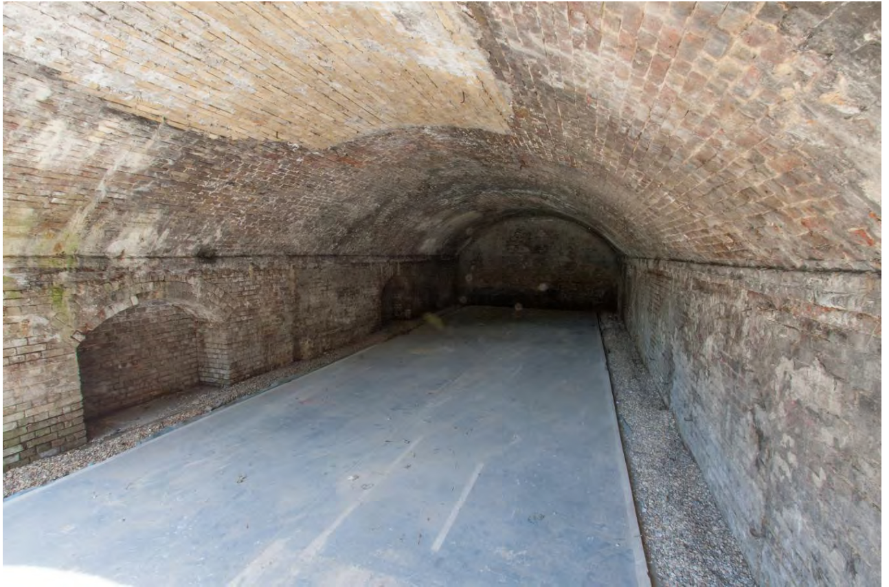
Plate 9 Arch 2 looking north (RWV13 D101 8398-2)
