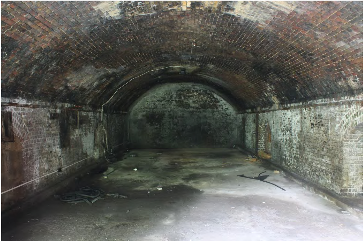
Plate 13 Arch 7 looking north
