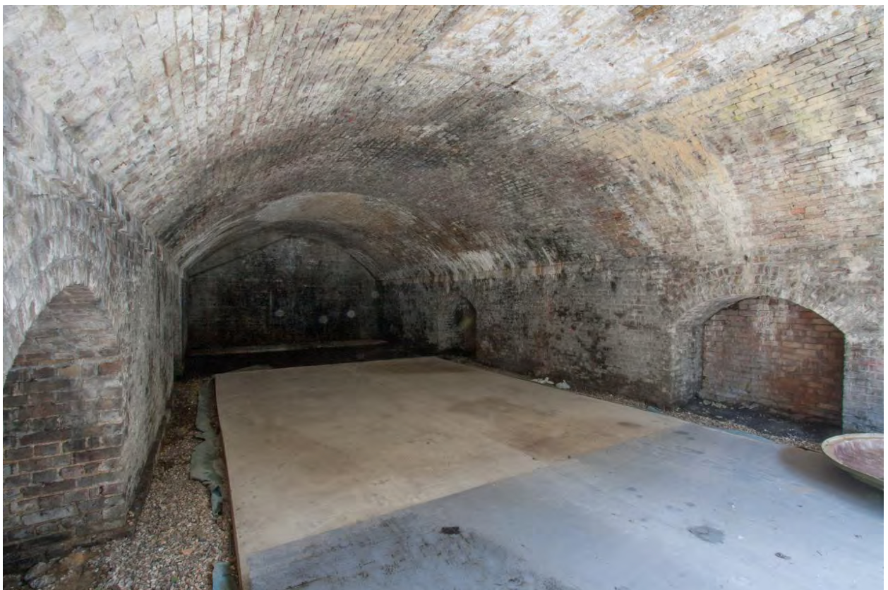
Plate 10 Arch 3 looking north (RWV13 D101 8392-2)
