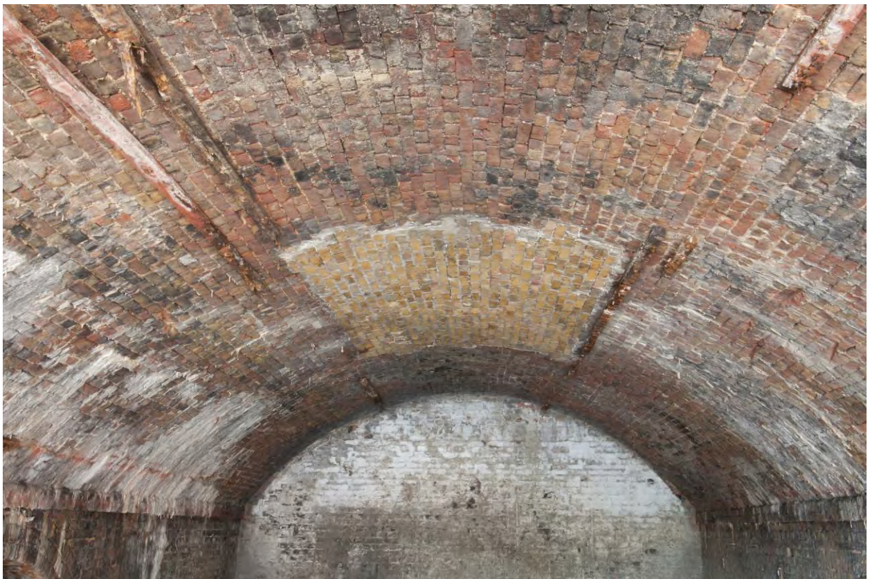
Plate 20 Blocked coal drop in Arch 11 looking north (RWV13 D101 8367-2)
