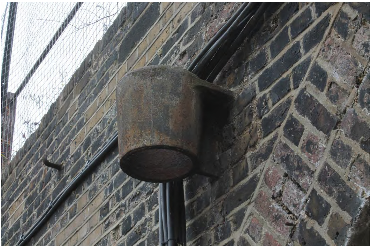
Plate 18 Cylindrical sleeve above Arches 10/11
