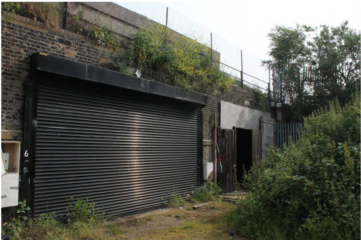
Plate 6 Apple Tree Yard, Arches 6-7 looking east
