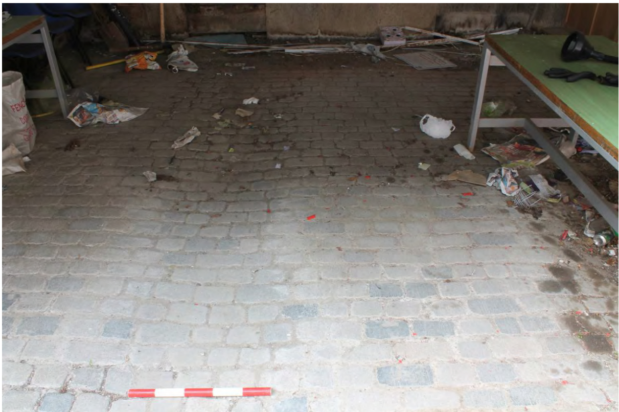
Plate 40 Granite sett floor Arch 21
