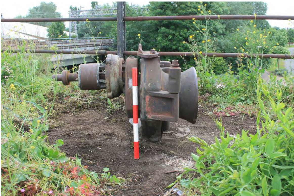
Plate 50 Mechanical winch looking east
