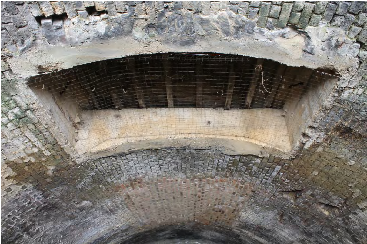
Plate 41 Later central coal drop Arch 23 with blocking to rear
