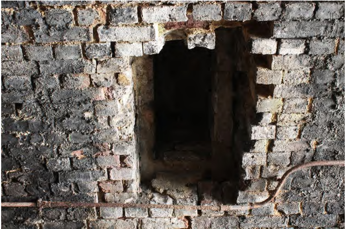
Plate 45 Smaller opening within vaulted ceiling of Arch 25
