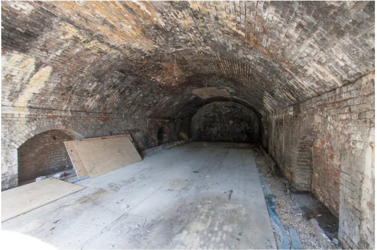
Plate 11 Arch 5 looking north (RWV13 D101 8379-2)
