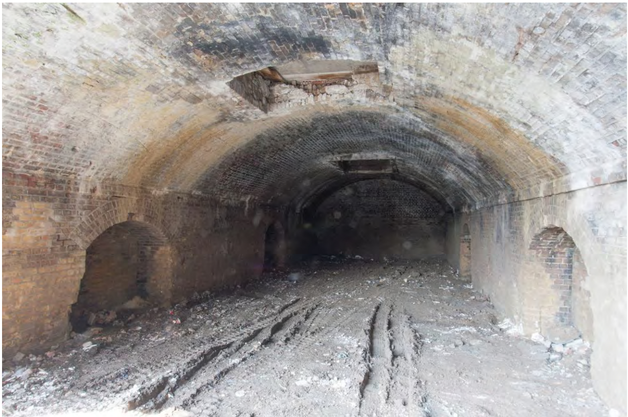
Plate 22 Arch 12 looking north (RWV13 D101 8352-2)
