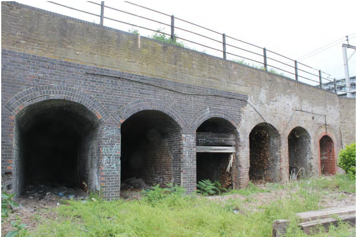
Plate 3 Eastern canal-side elevation looking north-west
