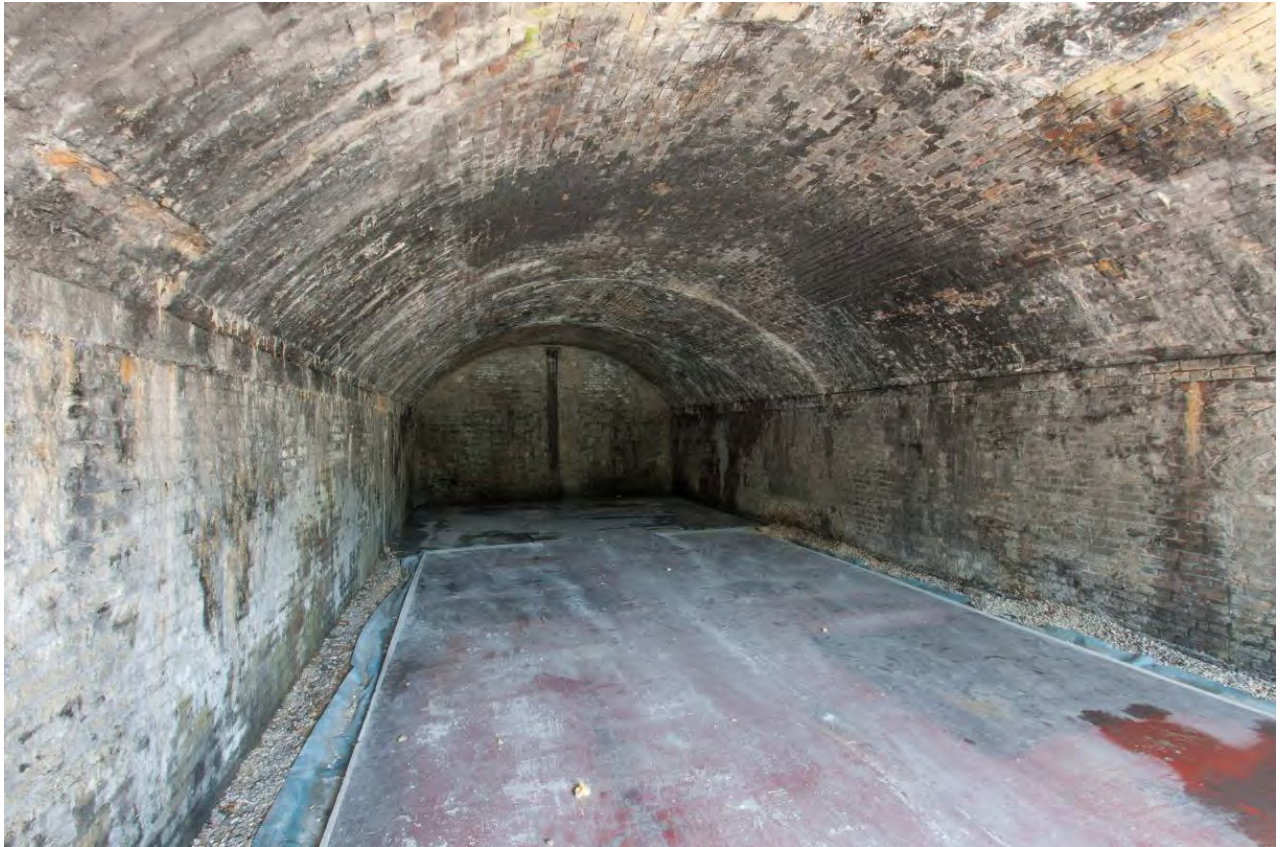
Plate 7 Arch 1 looking north (RWV13 D101 8403-2)
