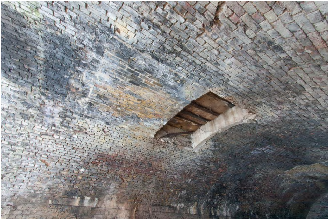
Plate 28 South coal drop in Arch 14 looking north-west (RWV13 D101 8345-2)
