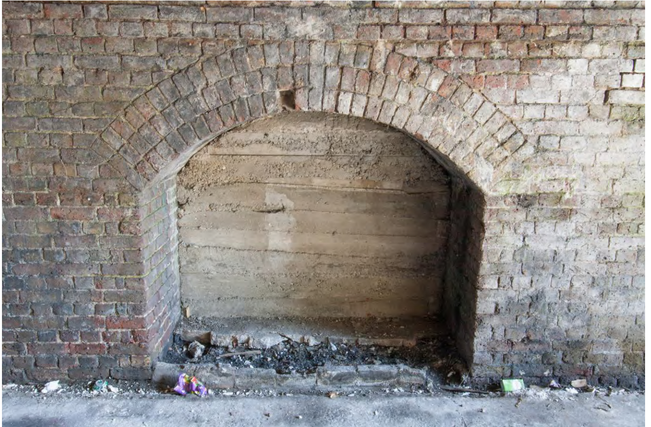
Plate 12 Transverse arch in Arch 6 looking east (RWV13 D101 8376-2)
