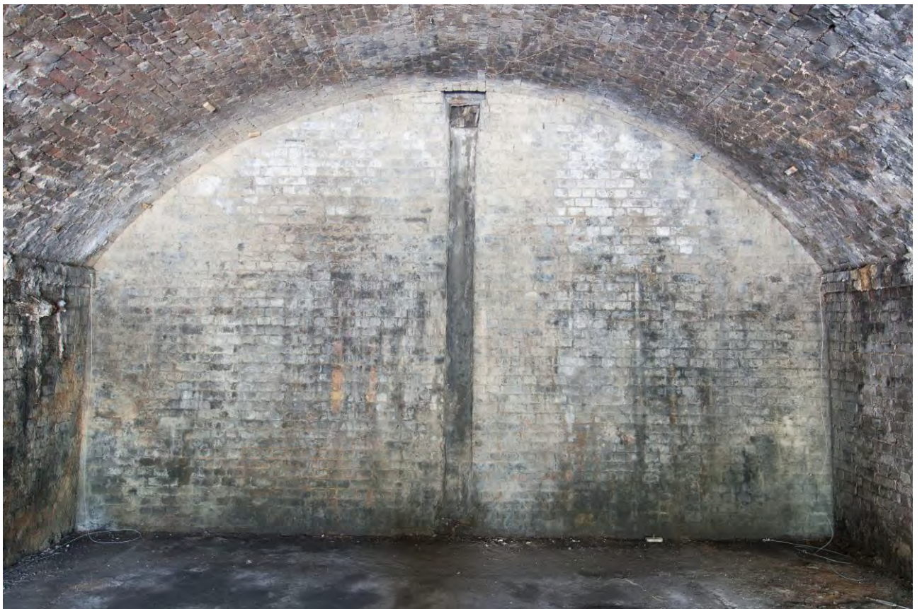
Plate 8 North wall of Arch 1 looking north (RWV13 D101 8406-2)
