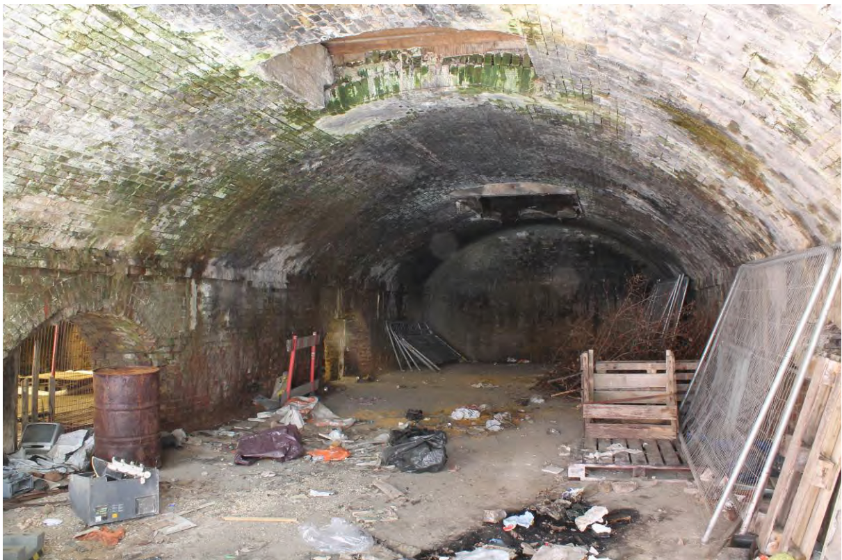
Plate 36 Arch 18 looking north
