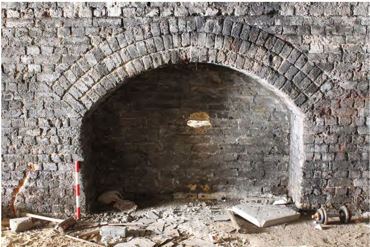
Plate 4 Typical transverse arch (blocked)
