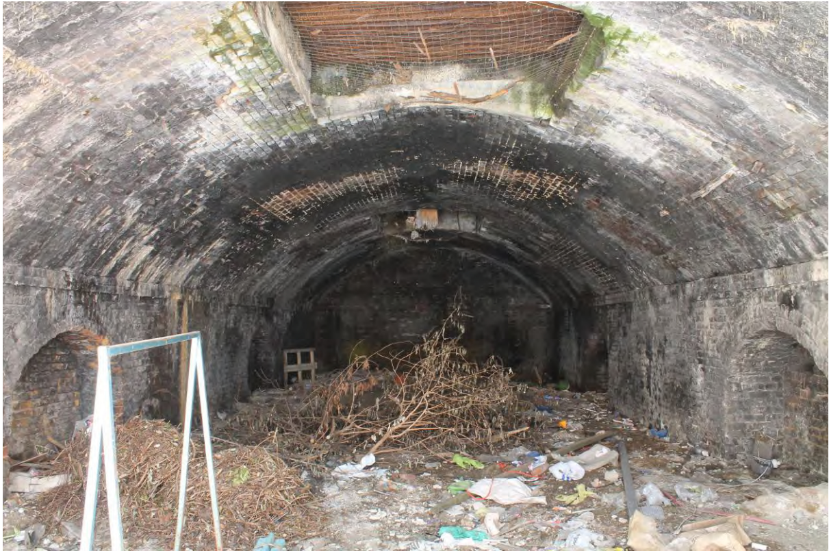
Plate 43 Arch 24 looking north
