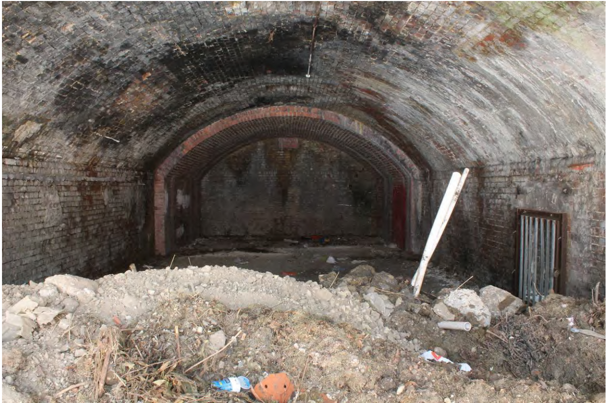
Plate 47 Arch 25 looking north, showing later inserted arch
