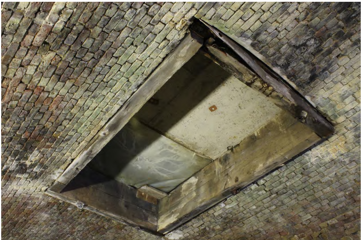
Plate 34 'Open' coal drop with timber lining in Arch 17
