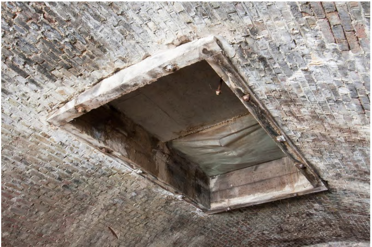
Plate 24 Timber-lined coal drop at the north end of Arch 12 looking north (RWV13 D101 8357-2)
