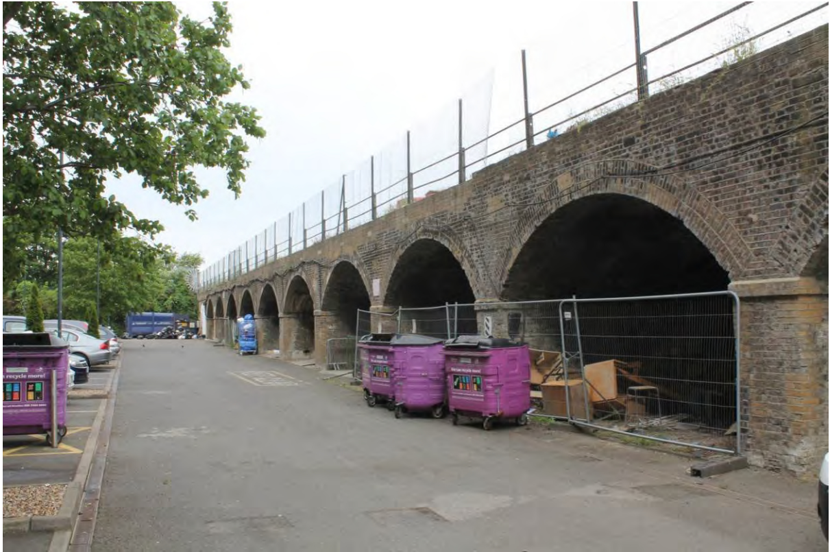
Plate 1 Viaduct from Arch 19 looking west
