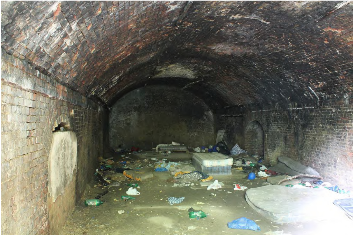
Plate 15 Arch 8 looking north
