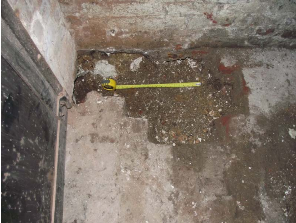
Plate 2: Test Pit 1 facing west Scale 0.50m
