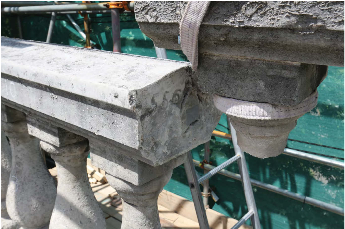
Plate 25 Lifting of coping stone 4 exposing the number on the north end of coping stone 10, looking south-west (CIS13 D1 3267)
