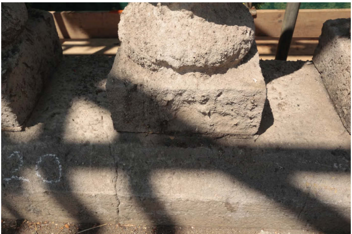
Plate 9 Cracks in plinth stone 20 and weathering on baluster 17, looking west (CIS13 D1 3217)
