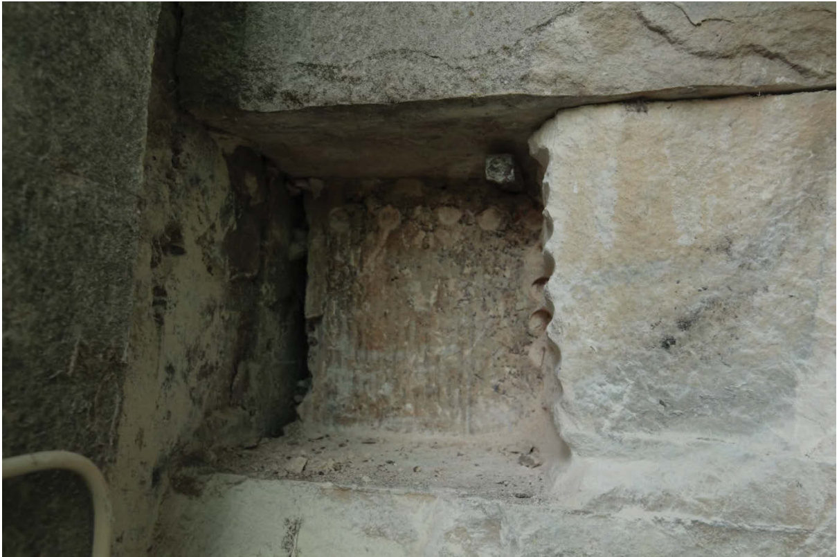
Plate 28 Metal fixing behind ashlar block, looking east (CIS13 D1 3294)
