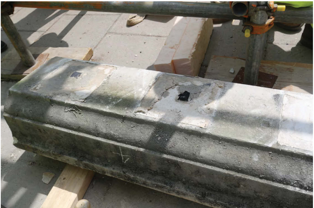
Plate 19 Underside of coping stone 4 with slate dowels, looking east (CIS13 D1 3273)
