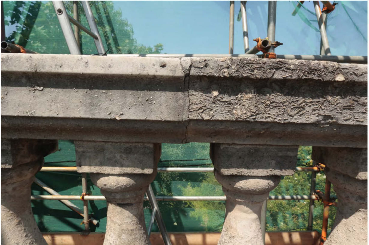
Plate 12 Differential height between coping stones 4 and 10, interior (east) elevation, looking west (CIS13 D1 3205)
