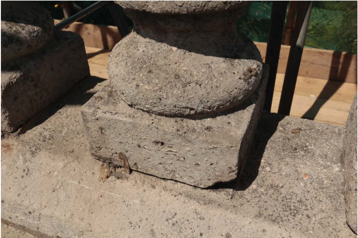
Plate 10 Detail of chip at base of baluster 7, interior (east) elevation, looking west (CIS13 D1 3201)
