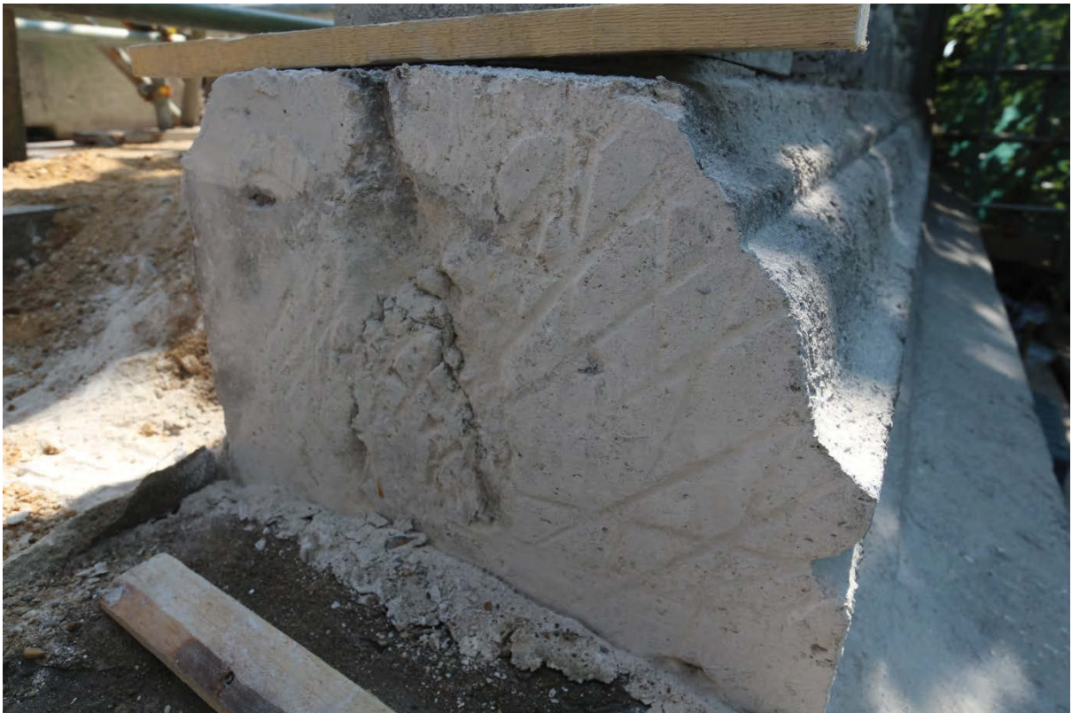
Plate 23 Joggle and poured cementitious mortar with aggregate in the north end of plinth stone 14, looking south-east (CIS13 D1 3279)
