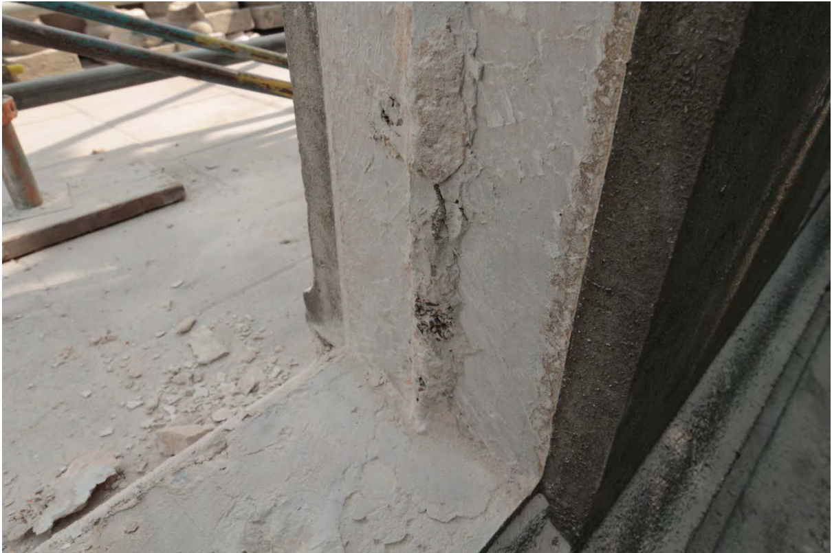
Plate 24 Removal of half baluster 22 exposing the upper surface of plinth stone 25 (left) and the north end of die stones 23 and 24 (right), looking south-east (CIS13 D1 3293)
