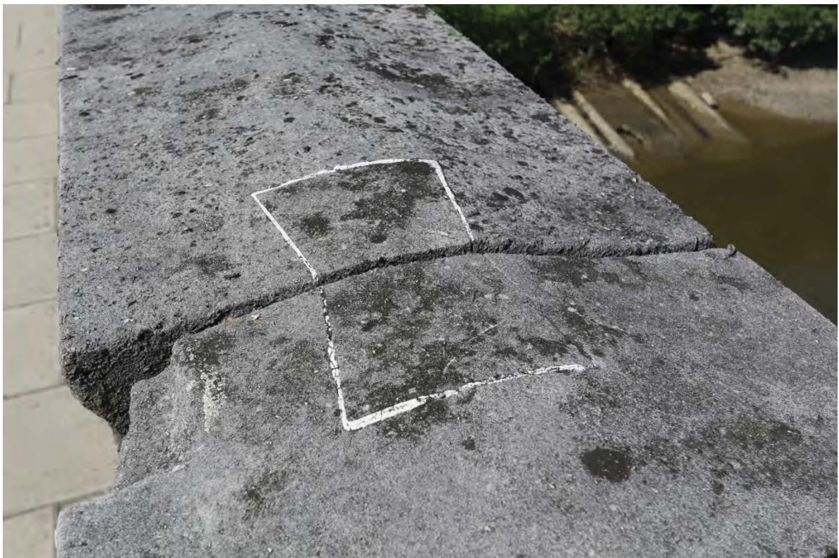
Plate 27 Butterfly repair, near the centre of the west side of the bridge, looking south (CIS13 D1 3257)
