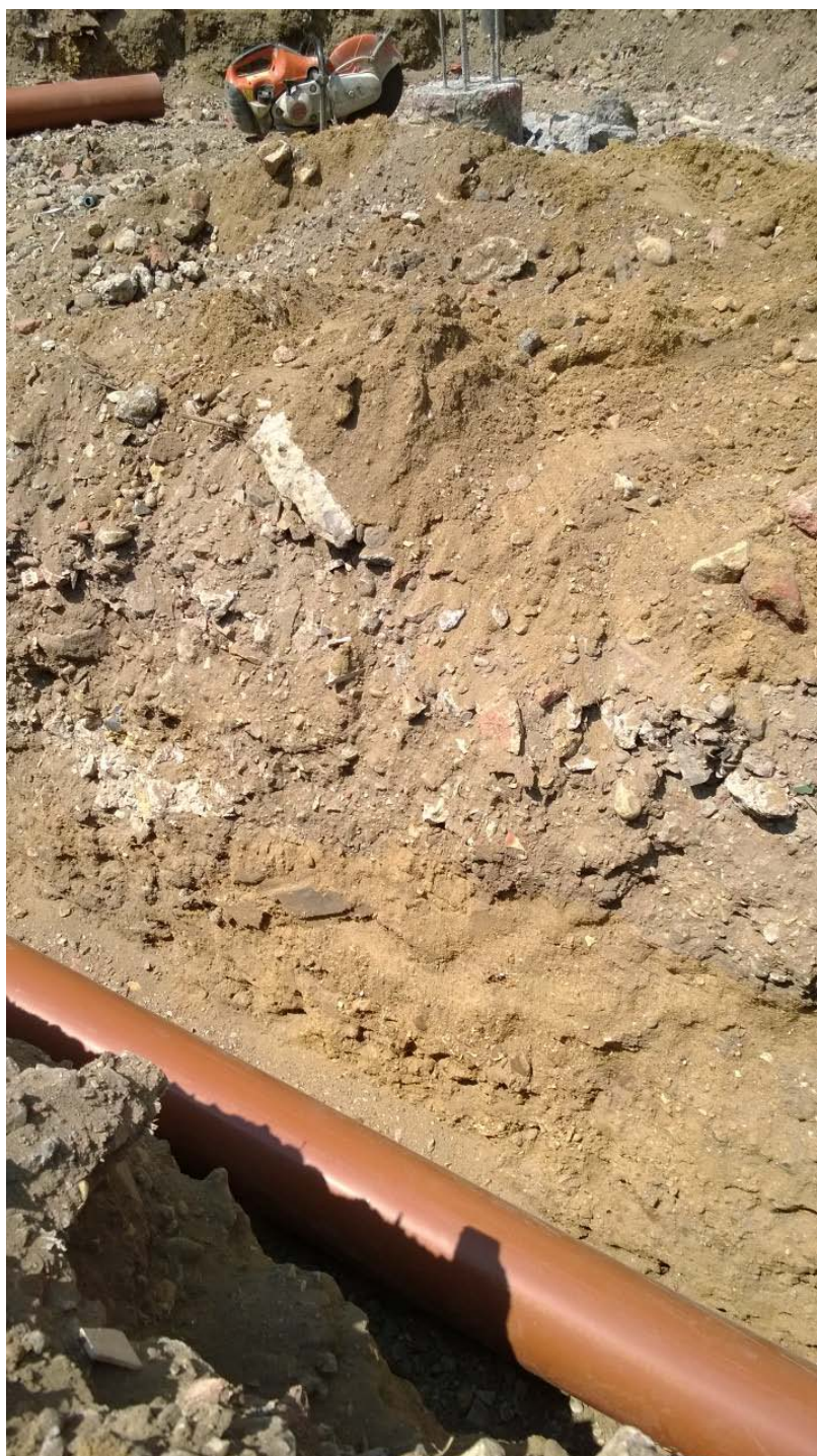
Plate 5: Southwest facing view of section within service trench
