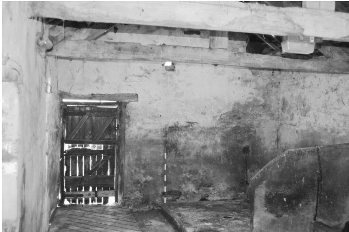
Photograph 24: Combination barn, south range, stable room interior, end wall (scale 1m)
