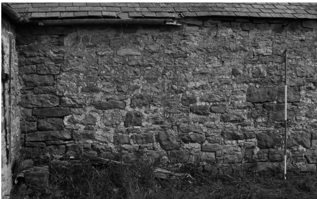
Photograph 8: Combination barn, south range, south facing elevation (west part) (scale 2m)
