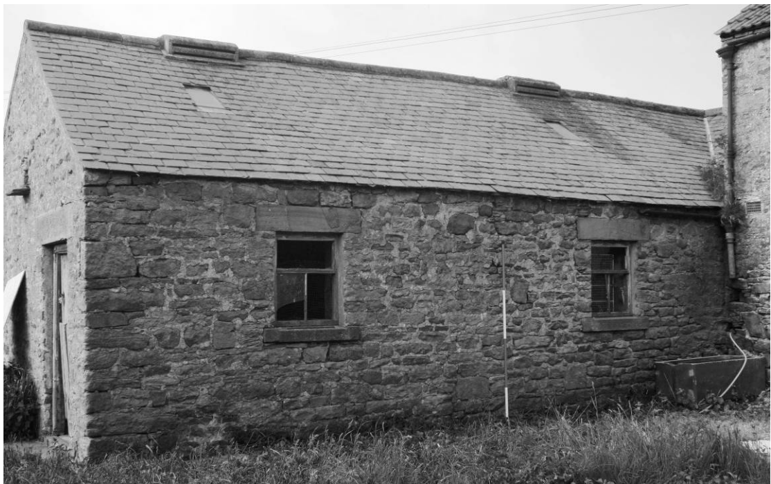
Photograph 6: Combination barn, south range, north facing elevation (oblique) (scale 2m)
