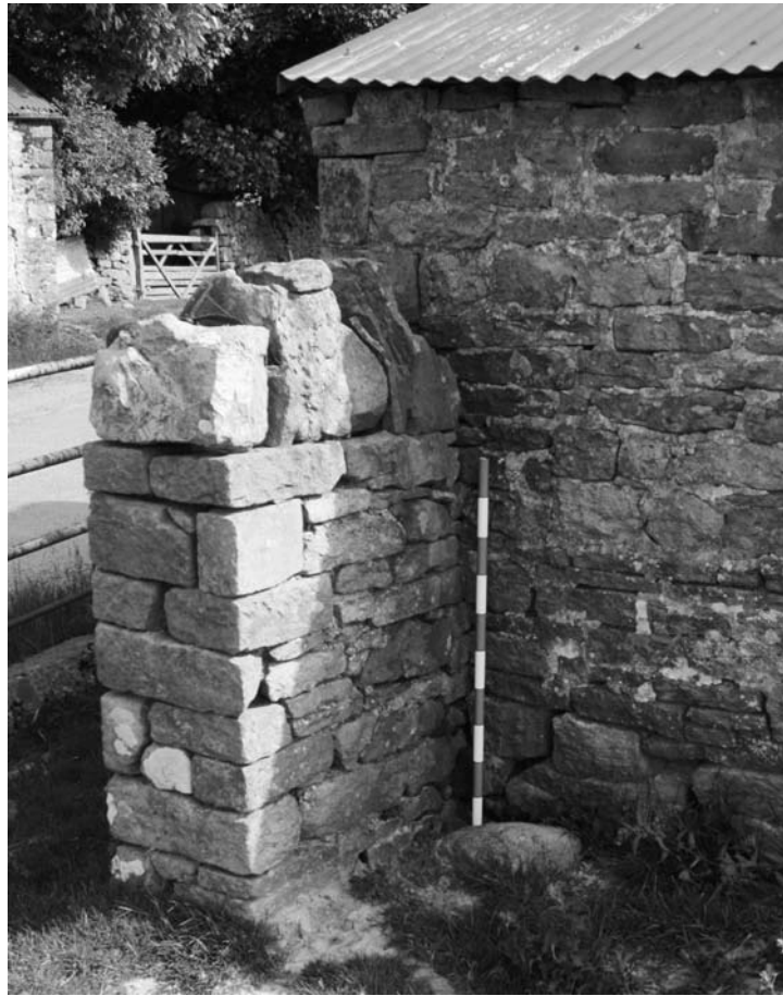
Photograph 33: Lean-to barn, section of wall external to south-west corner (scale 1m)
