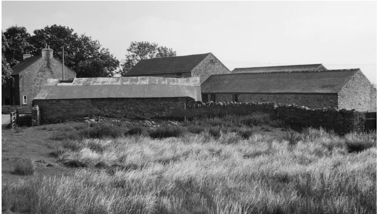
Photograph 32: Overview of complex, looking north-east (scale 2m)
