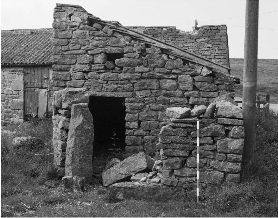
Photograph 27: Animal housing, north-west range, north-east facing elevation (scale 1m)
