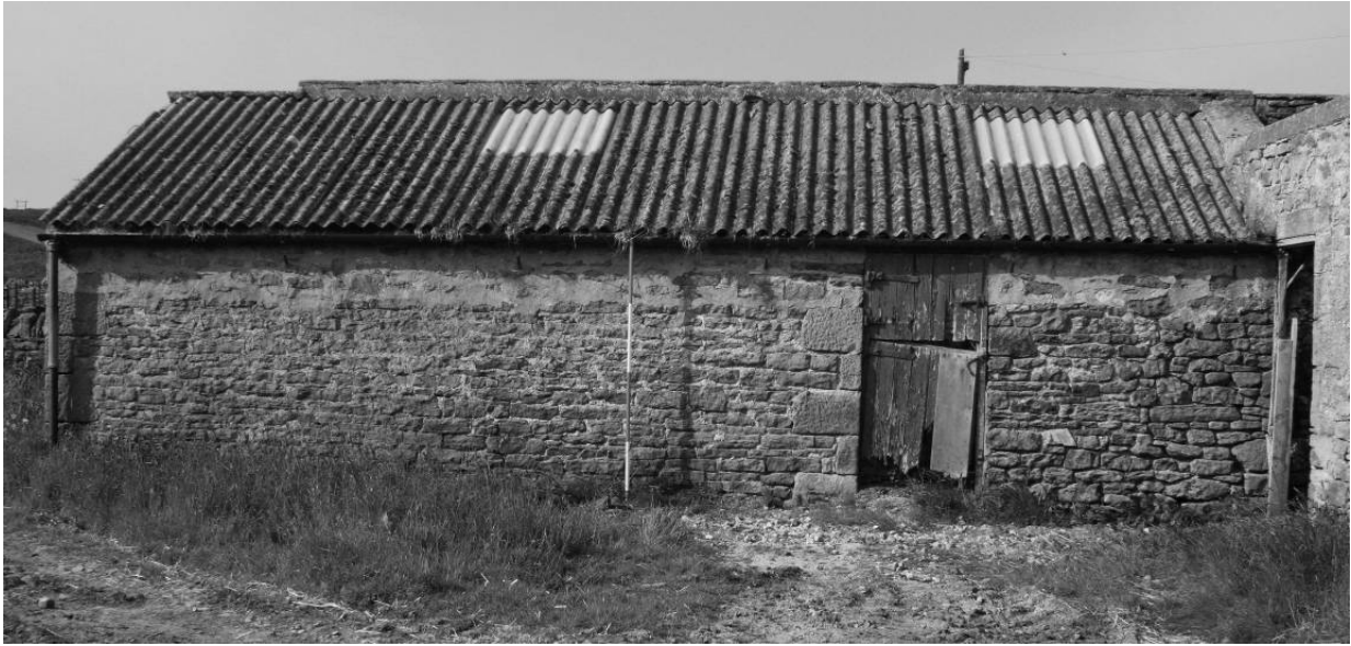
Photograph 29: Animal housing, south-west range, north-east facing elevation (scale 2m)
