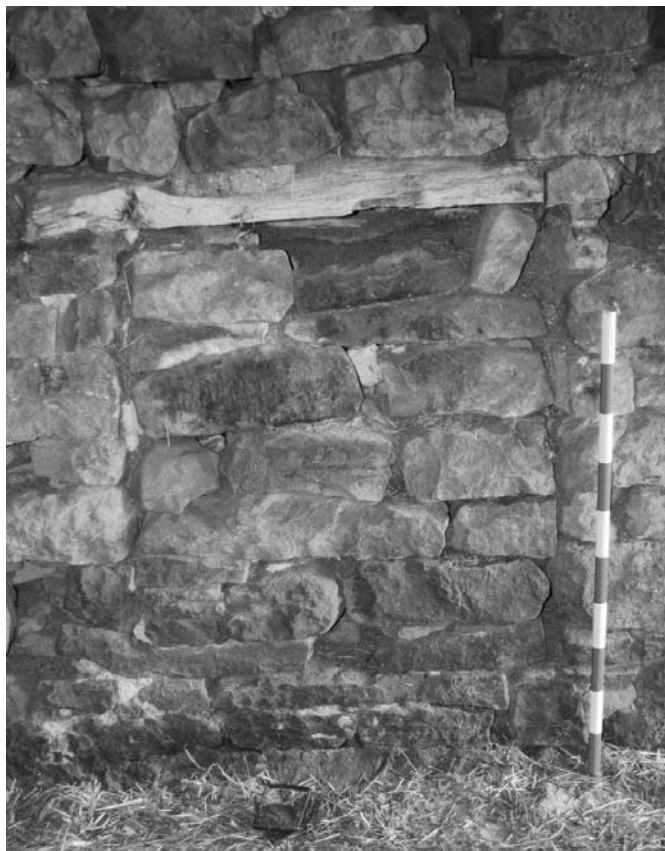
Photograph 38: Lean-to barn interior, north-east wall, detail of infilled opening (scale 1m)
