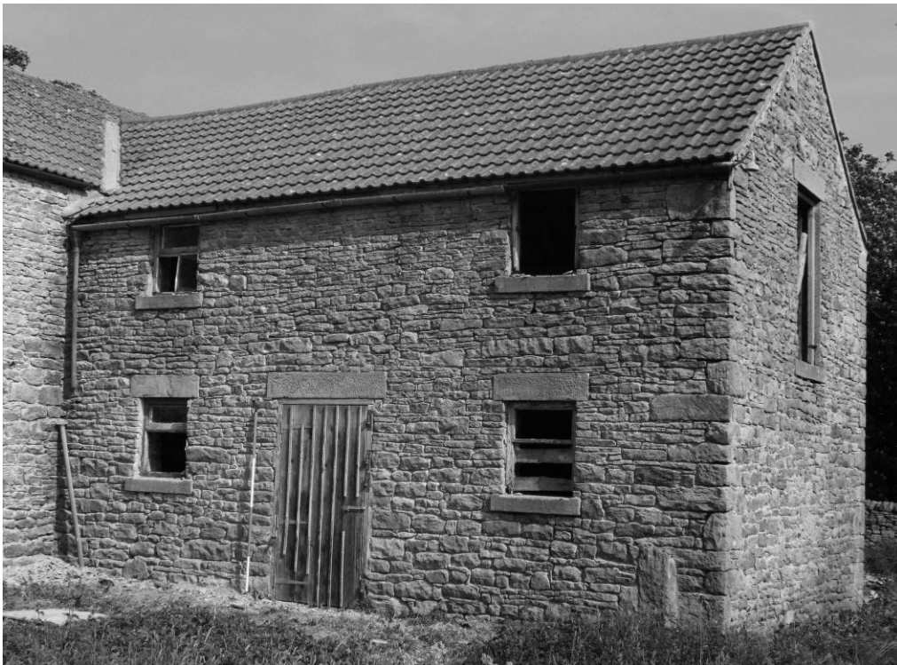
Photograph 4: Combination barn, north range, south facing elevation (oblique) (scale 2m)
