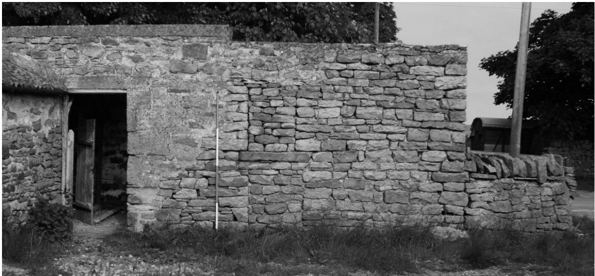
Photograph 28: Animal housing, north-west range, south-east facing elevation (scale 2m)
