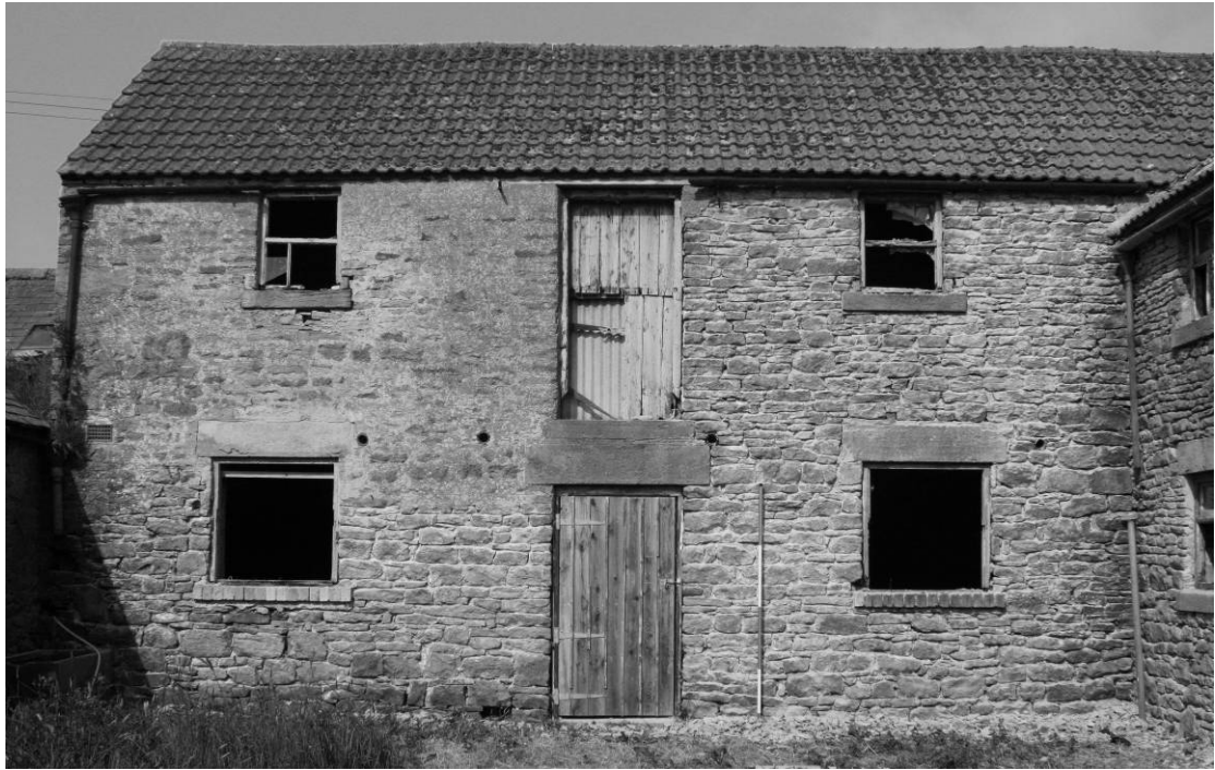
Photograph 5: Combination barn, west range, north part, east facing elevation (scale 2m)
