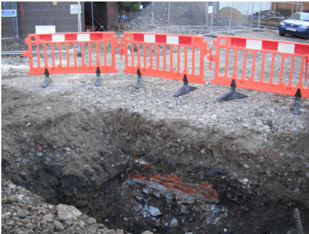
Plate 4: Section of Footing 4C showing surviving brick and chalk wall, facing south
