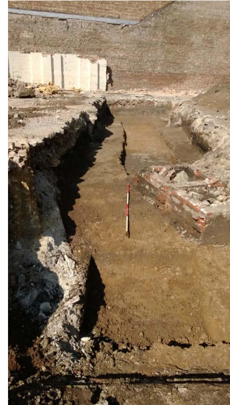
Plate 2: Trench 1 north-east facing
